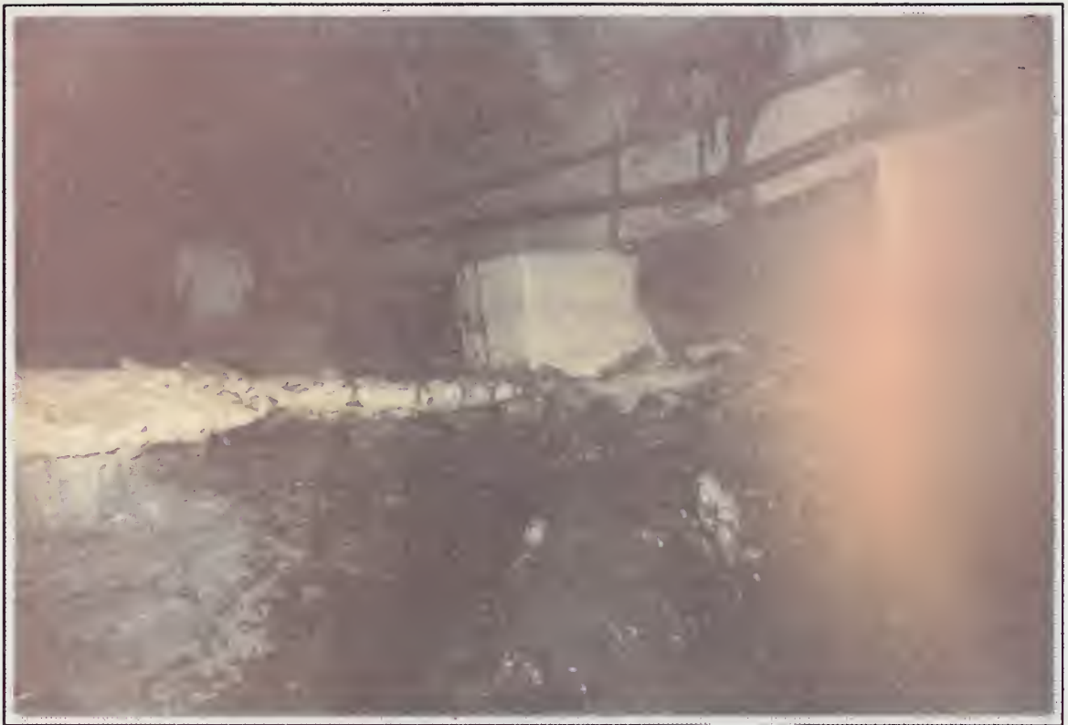
3.3 Pedestal and Erosion of the Tunnel Invert (About Sta. 190+00)
