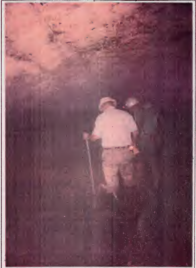
3.8 Tunnel Crown. Shotcrete or gunite treatment. (About Sta. 60+00 Whittington Branch)
