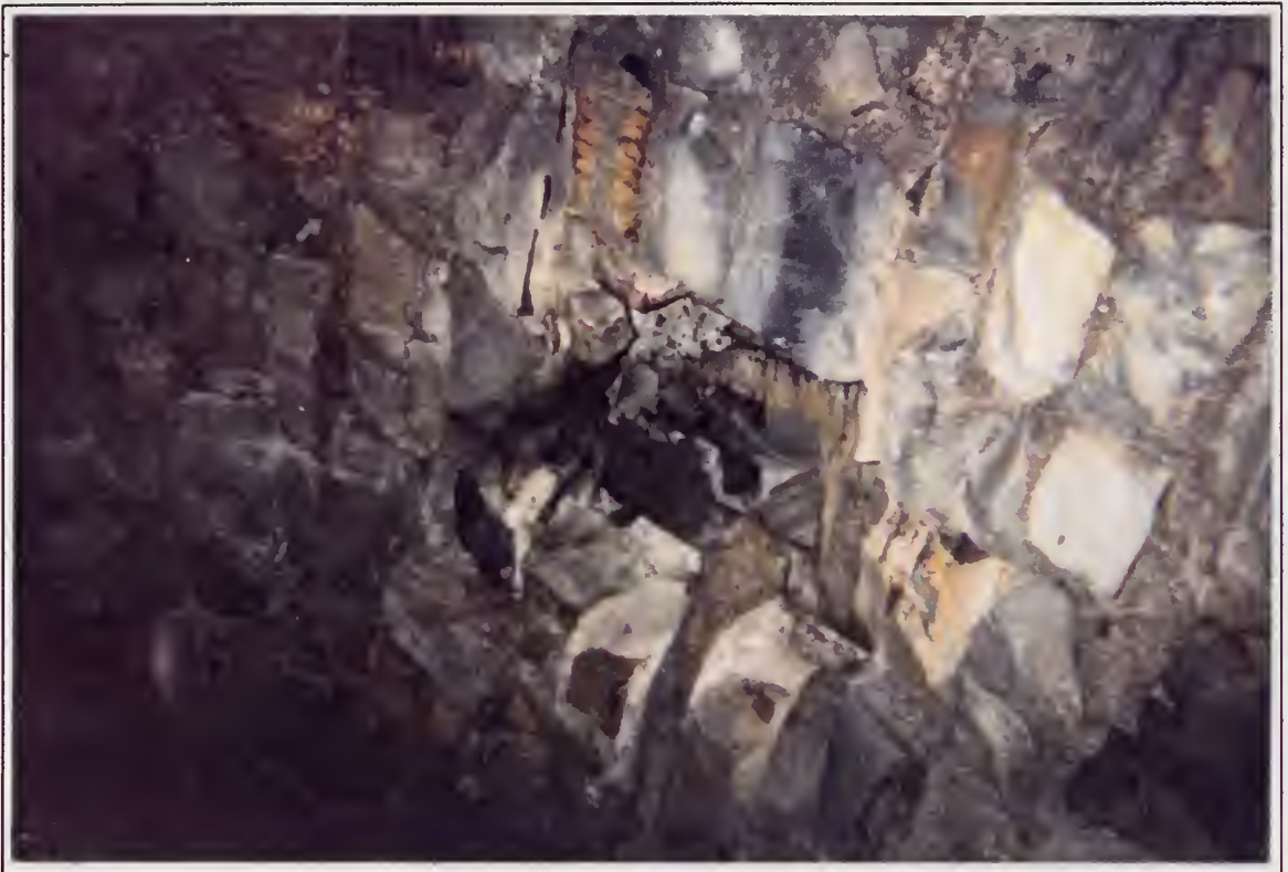
3.6 Crown of the Tunnel. Wooden blockout for drainage into the tunnel is visible in the crown. (About Sta. 200+00)
