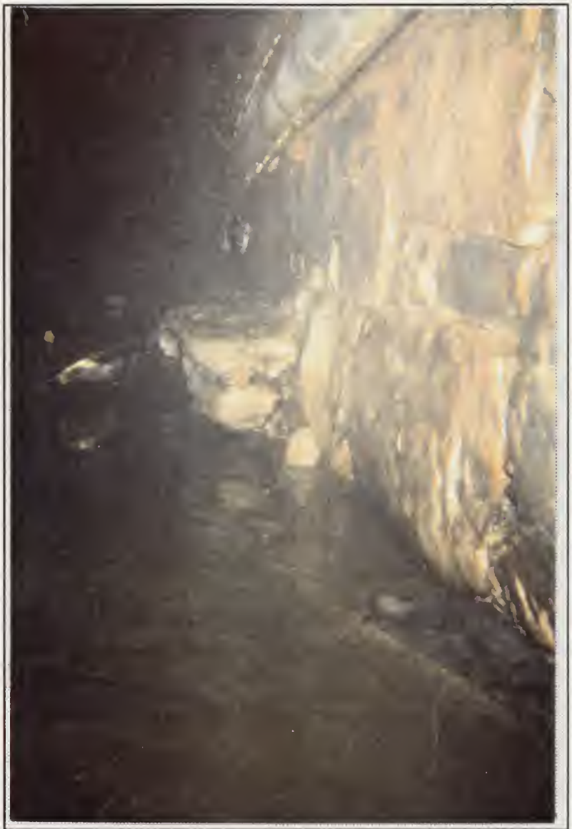
3.13 Erosion of the Base of the Sidewalls of the Tunnel. Erosion of previously placed concrete is visible. (About Sta. 240+00)
