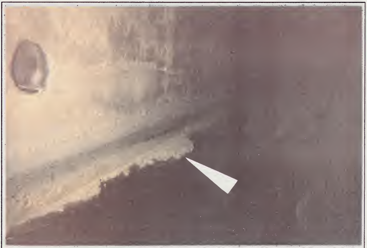
3.2 Sidewall of the Tunnel. The base of the sidewall has been severely undercut. The concrete traces the base of a previous repair. (About Sta. 187+00.)
