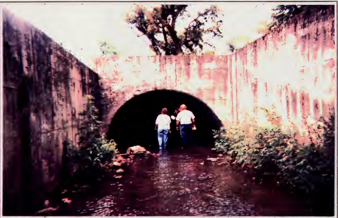
3.7 Whittington Avenue Entrance. The structural steel plate is just visible inside the tunnel. (About Sta. 72+00 Whittington Ave Branch COE Map Figure 2.3)
