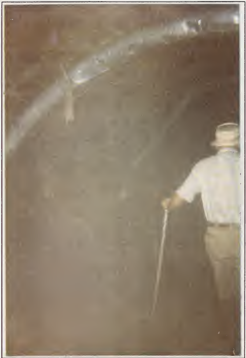
3.9 Insulated Piping Crossing the Tunnel Crown.
