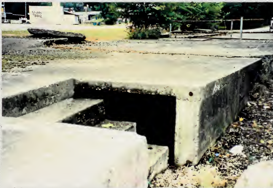
3.12 Vault near Arbor and Loadstone. Unprotected opening and slab thickness are shown.
