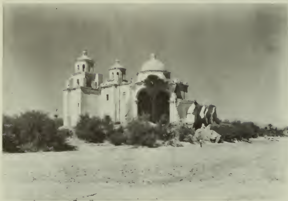
Mission La Concepcion de Nuestra Senora de Caborca. A view from the dry Magdalena River bed, showing how the flooding had undermined major parts of the church. (photo, courtesy of John Clonts, WACC, Tucson, Arizona)
