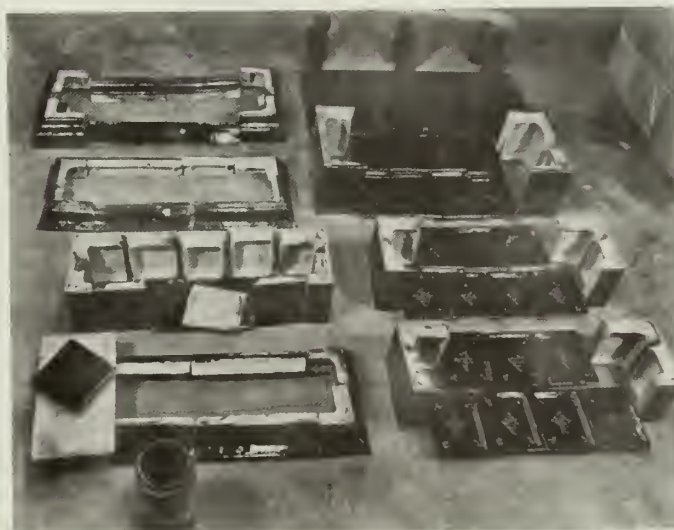
FIGURE 278. PARTS TO MAKE THE STOVE SHOWN IN FIGURE 277. NOTE STOVE TILES (FROM BIVANS, 1972).
