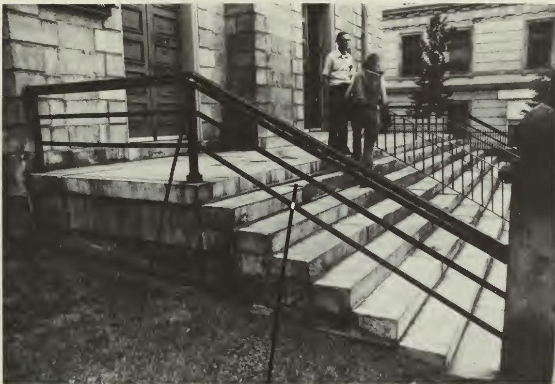
a,b. TWISTED OR ROTATED SLABS CAUSING POSSIBLE WATER PENETRATION AND MORTAR LEACHING - NEEDS FUTURE ATTENTION
