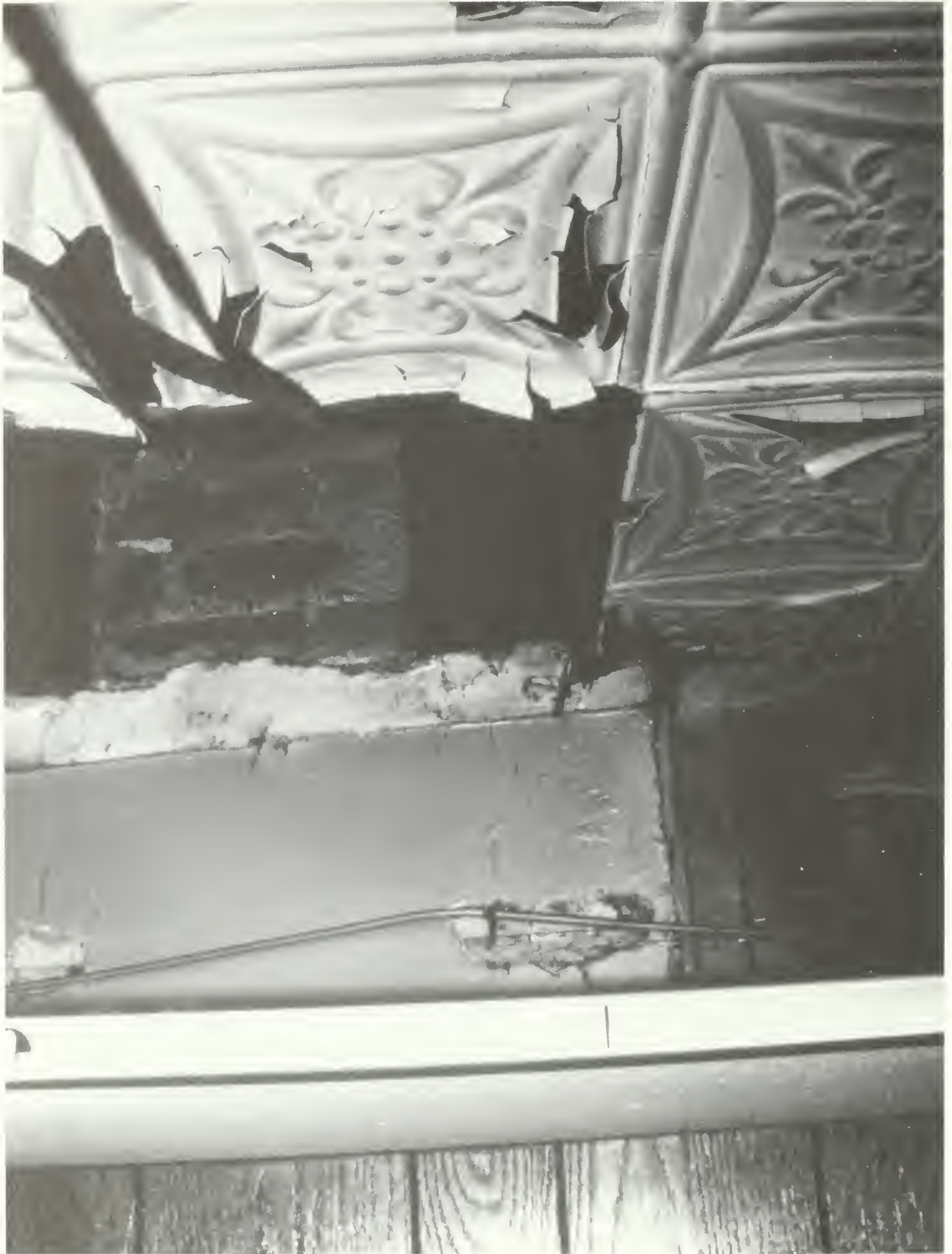
Figure 28. Room 101, exposed pressed-metal ceiling.
