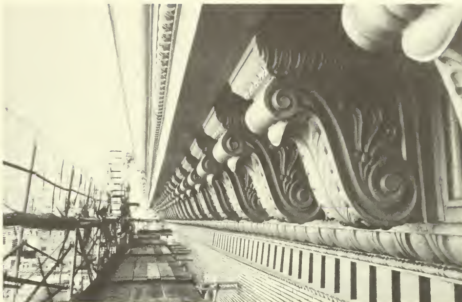
Figure 11. The completed cornice is shown after painting and immediately prior to removal of the scaffolding. Photo: Richard Pieper.
