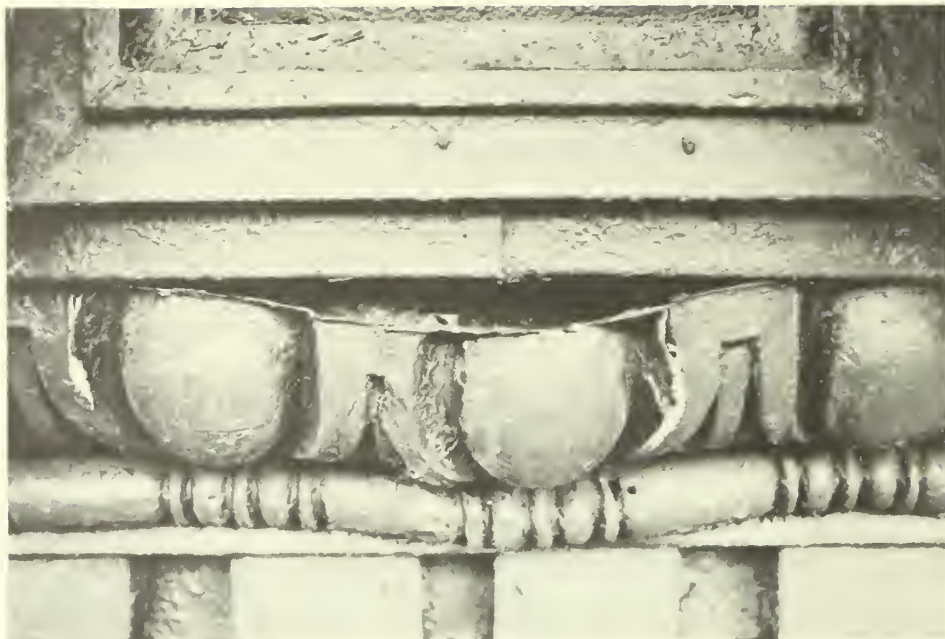
Figure 5. Most of the egg and dart molding on the cornice had deteriorated over the years and required replacement. Photo: Richard Pieper.
