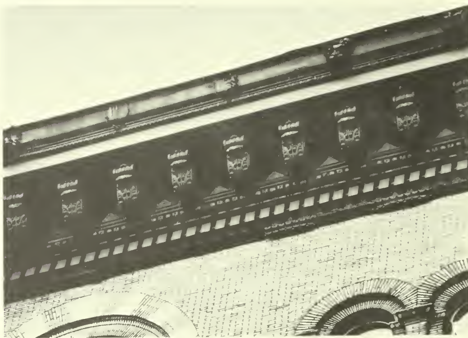
Figure 6. Three of the components of the metal cornice which required replacement because of serious deterioration are shown in this view. They are the lions' heads on the crown molding (several are missing due to failed soldered joints), modillions, and the egg and dart molding at the base of the cornice. The brake-formed galvanized steel that comprised the lineal moldings of the cornice, the soffit and dentil band were in sound condition. Photo: Richard Pieper.
