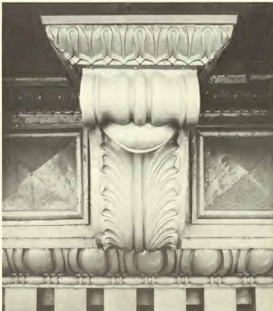
Figure 12. Detail of the completed cornice shows the new zinc modillion and the leaf and egg and dart moldings attached to the historic cornice. This repair approach, which involves in-kind replacement of deteriorated components, is the recommended treatment for such distinctive features as this cornice. Photo: Michael Devonshire.
