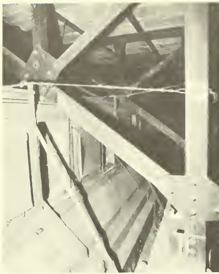
Figure 1. Large steel trusses cantilever out from the masonry parapet to support the cornice. Metal facing of the cornice was bolted to small iron or steel ribs (as at left). Wire ties helped to pull the center of the cornice tight to the bottom member of the truss. Photo: Richard Pieper.
