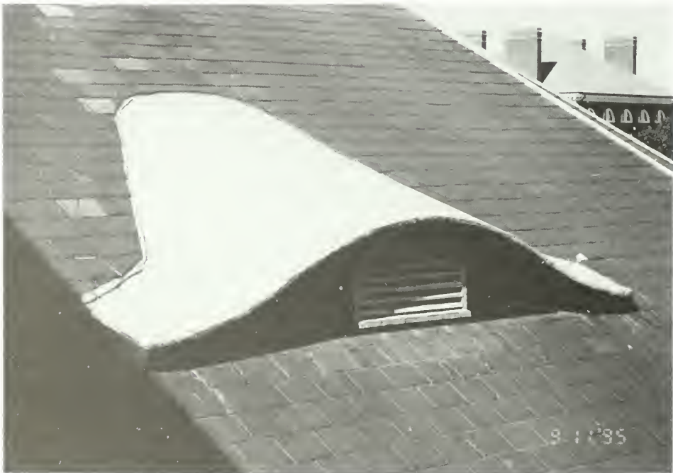
Figure 58. Addition exterior: roof and south "eyebrow" window (W201).
