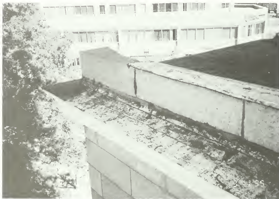
Figure 98. Tower exterior: base, north end of west parapet. Note inappropriate use of bituminous asphalt to seal masonry joints and to parch the copper flat-seam roof; flashing is missing from parapet wall.
