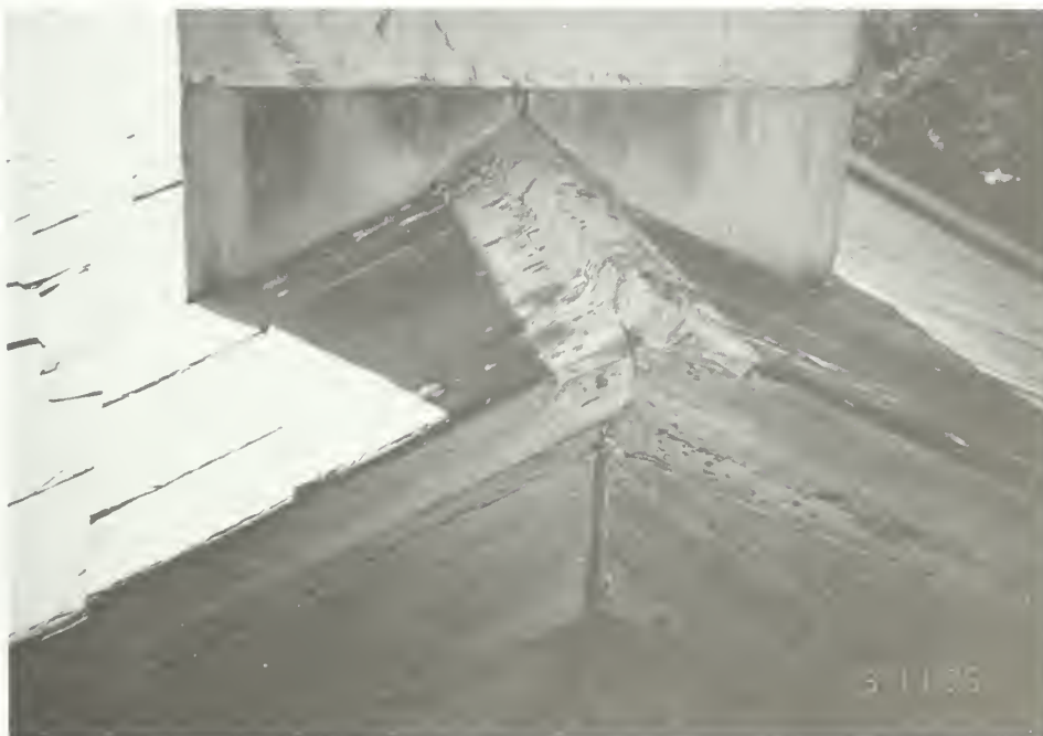
Figure 72. Church exterior, roof ridge cap at east end.
