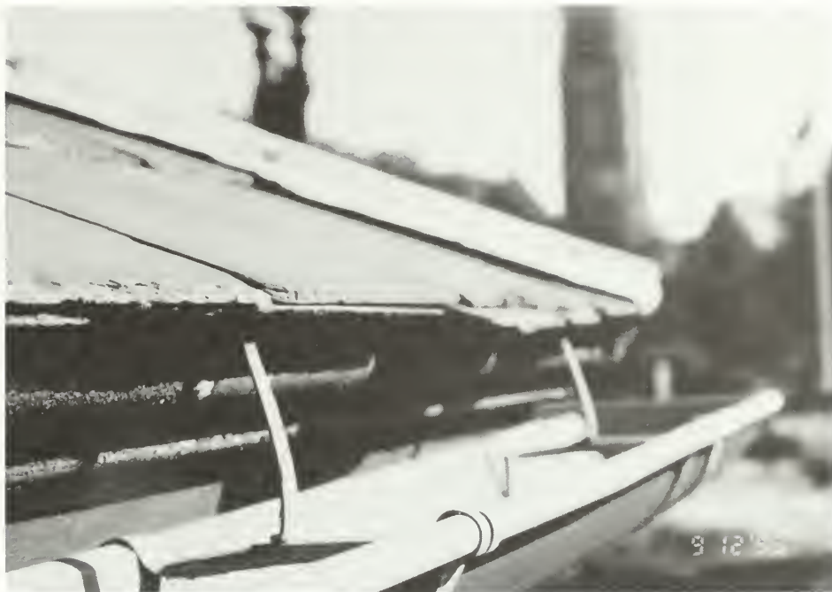
Figure 103. Addition exterior: east end of south half-round copper gutter and cornice. Note lifting slates and hip ridge cap, and peeling paint, dry wood, and open joints of cornice.
