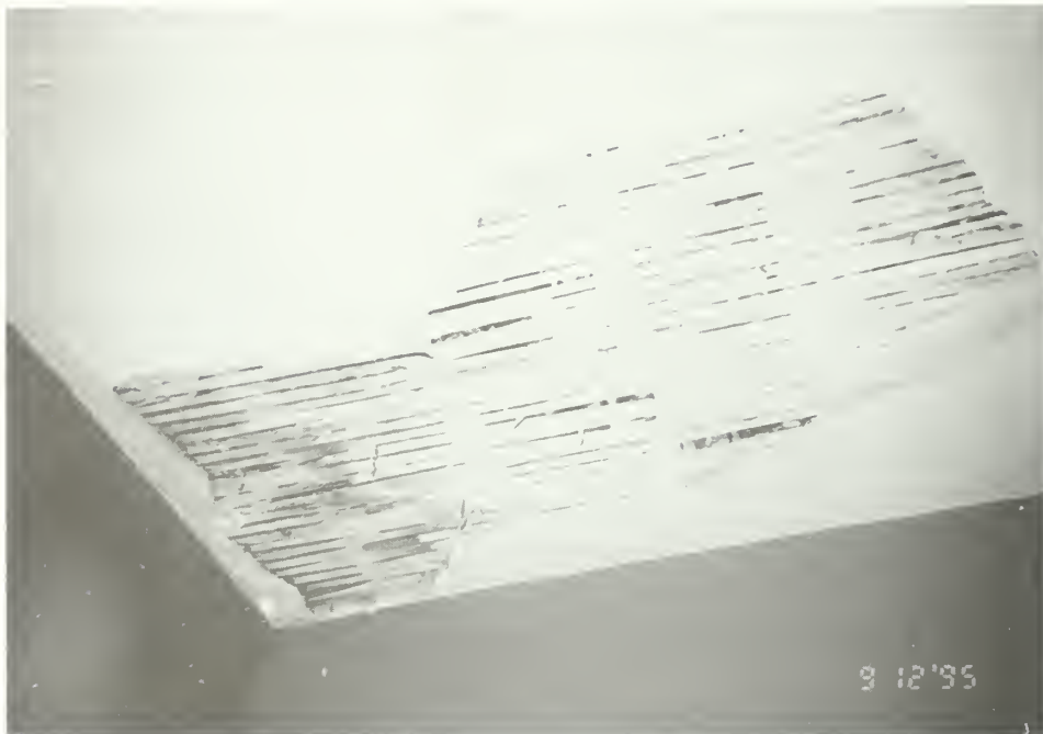
Figure 119. Tower interior: second-story vestibule south room (Room 202), southeast corner of ceiling where plaster has fallen due to failed plaster keys due to roof leaks.
