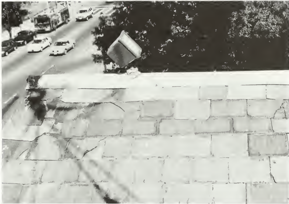
Figure 67. Tower exterior: west portico, slate roof with copper ridge cap. Note cracked and repaired slates, bituminous patches, loose copper flashing, and spotlight screwed to ridge cap.
