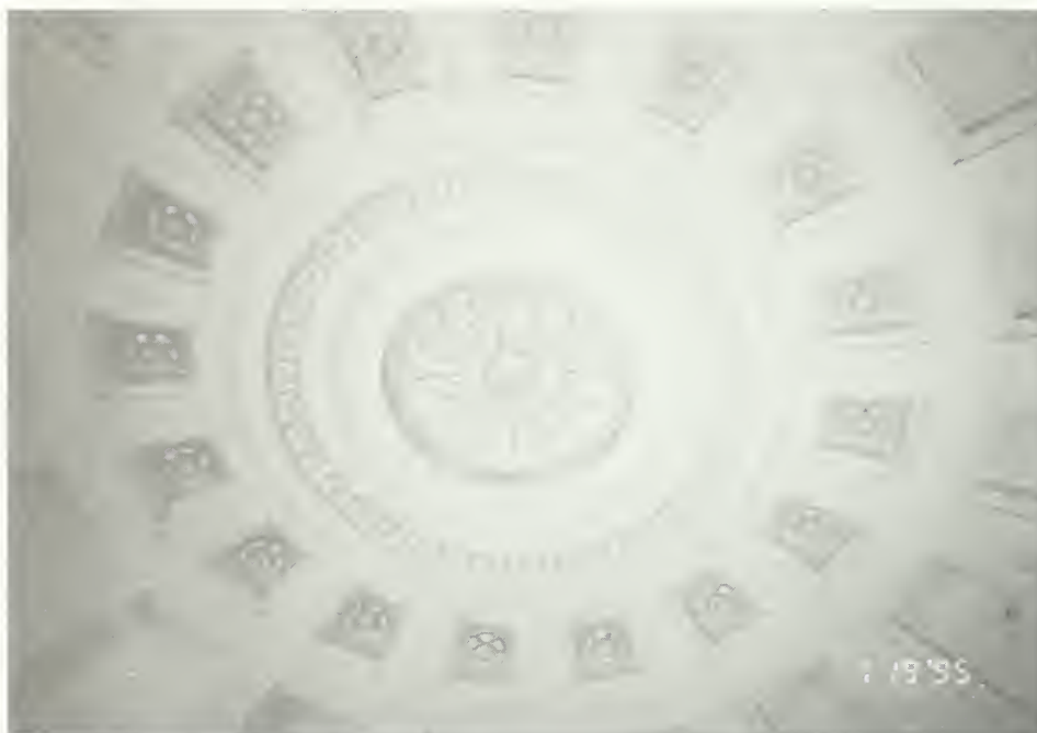
Figure 115. Church interior: sanctuary (Room 103), coffered dome ceiling. Note minor areas of diagonal cracks and water stains from roof leaks.
