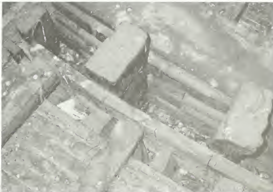
Figure 110. Church interior: attic, view of plaster keys of sanctuary's coffered ceiling dome. Note accumulation of debris and pigeon droppings, although bird access now seems blocked.
