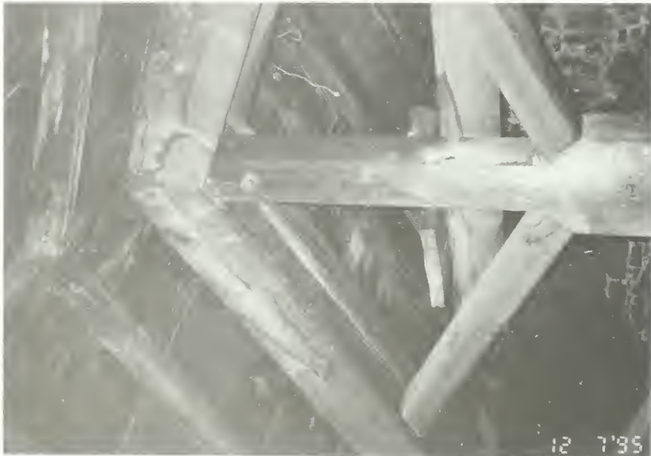
Figure 111. Church interior: attic, westward view of king post, rafter, and sheathing. Note water damage from leaks, mold growth, and rusting chicken wire.
