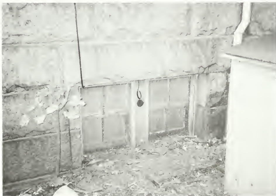
Figure 108. Addition exterior: north wall, basement window (W015). Note wire security mesh, soil above sill level, peeling paint, and biological growth, which affect both windows and the granite foundation.
