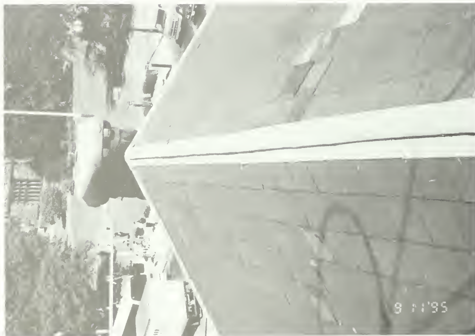
Figure 101. Addition exterior: slate roof and copper ridge cap, view eastward. Note replacement shingles, rolled copper ridge cap, and granite chimney.
