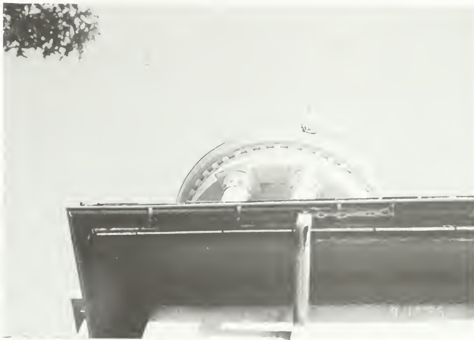
Figure 75. Church exterior: southwest corner of roof, showing hanging half-round copper gutter and rectangular downspout, with oxidation and pitting of the copper.
