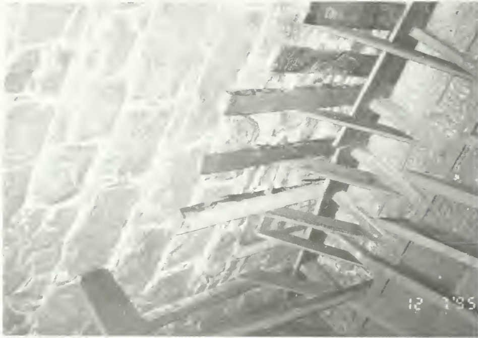
Figure 112. Church interior: attic, north end of east wall, at intersection with sanctuary ceiling. Note repointed mortar joints of wall.
