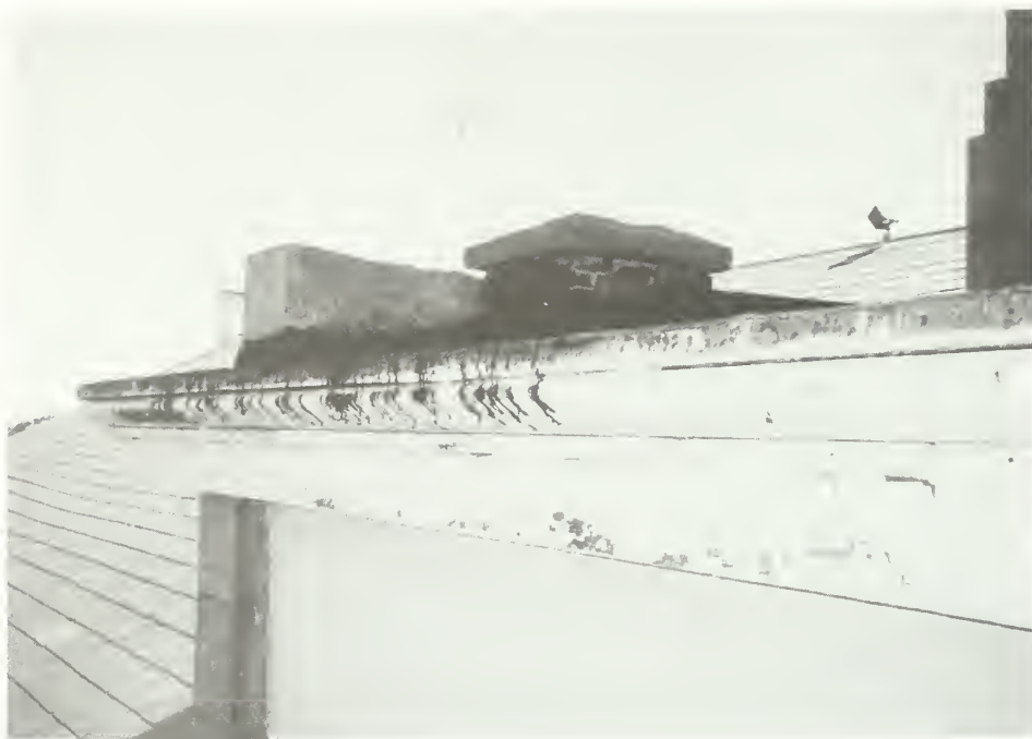
Figure 97. Tower exterior: base, cornice of north side of roof. Note careless application of bituminous asphalt over flat-seamed copper roof, and typical lack of maintenance of inaccessible areas.
