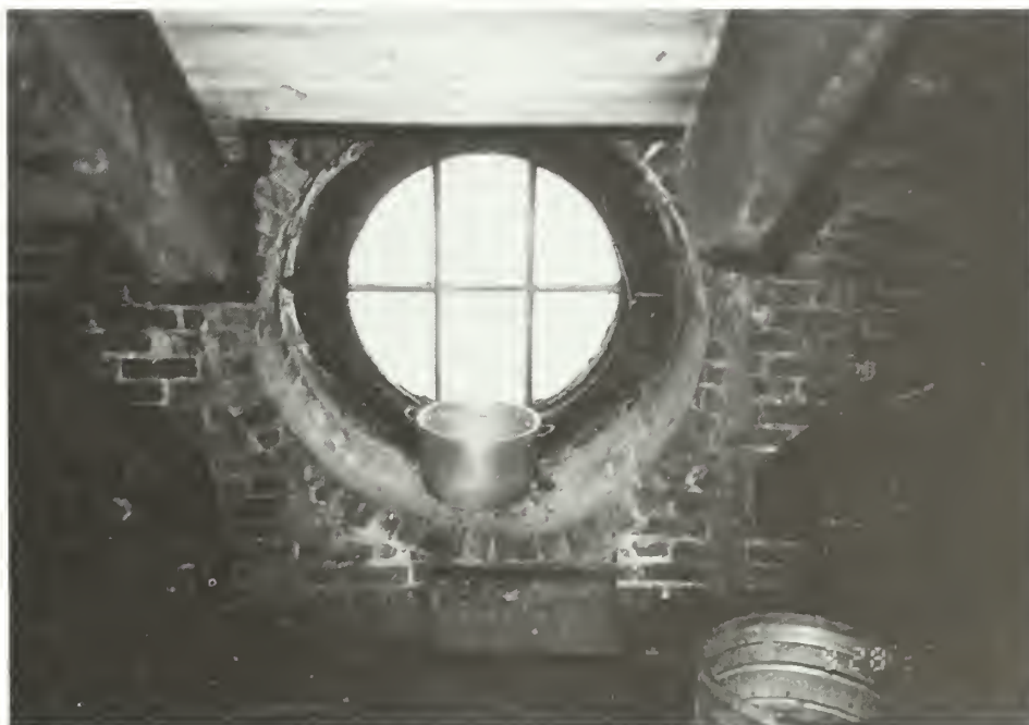
Figure 104. Addition interior: east wall, attic oculus (W202). Note effects of leaks through the flashing and/or the open joints of the sash and surround, and repointing of brickwork.
