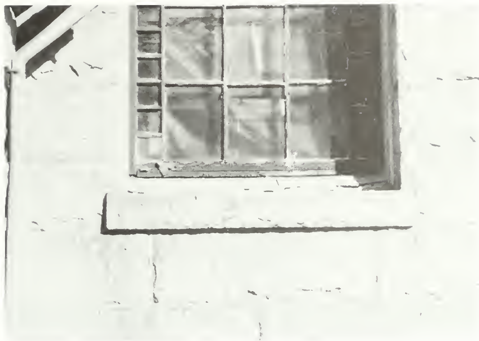
Figure 107. Addition exterior: south wall, bottom of center window (W108). Note dry wood, peeling paint, and open joints of both sash and surround.
