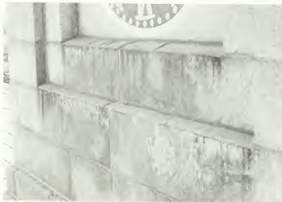
Figure 94. Tower exterior: shaft, north side below clock face. Note minor stains and discoloration and open joints of granite.
