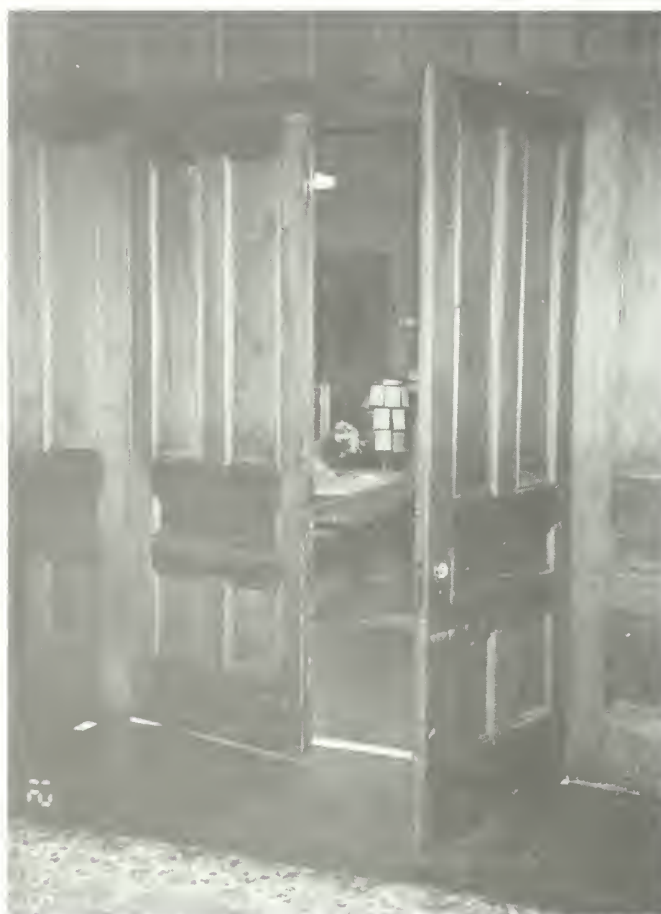
Figure 66. Addition interior: Ladies' Parlor (Room 107), west partition wall that can be lowered from attic.
