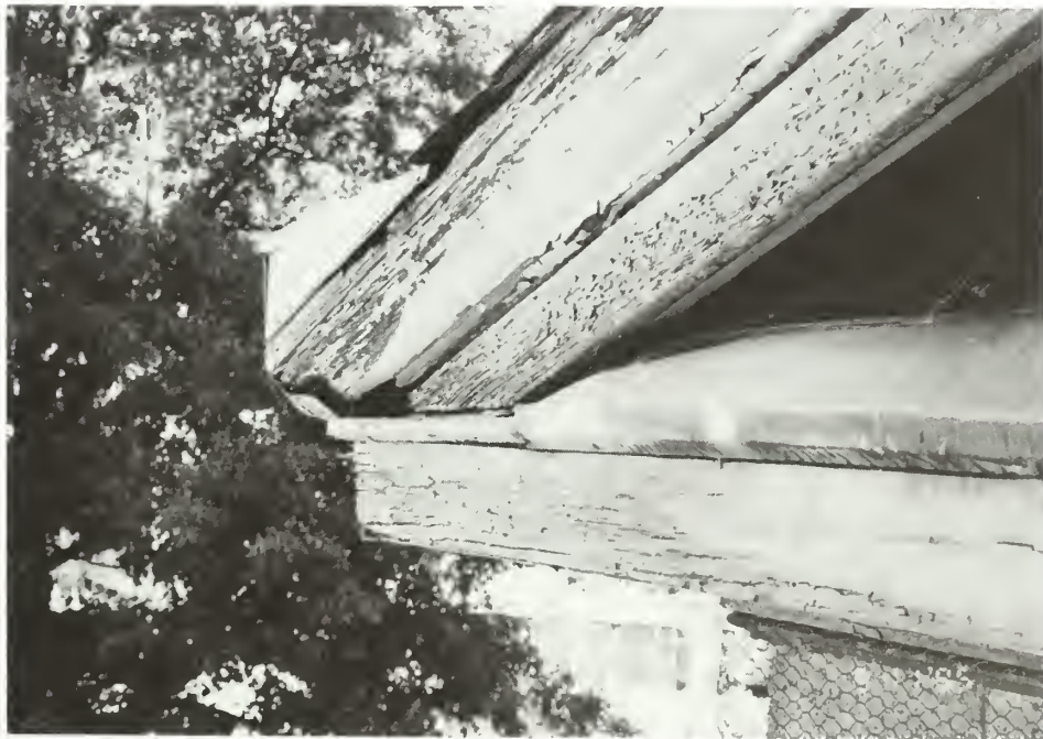
Figure 68. Tower exterior: west portico, north end of entablature. Note peeling paint, cracked moldings, open joints, and granite stains from rusting chicken wire.
