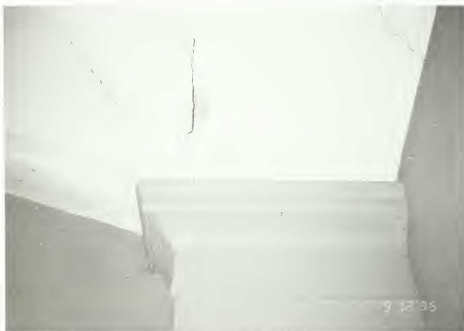
Figure 116. Church interior: sanctuary (Room 103), southwest corner at intersection of ceiling and wall pilaster. Note largest plaster-wall crack and water stains from leaks.
