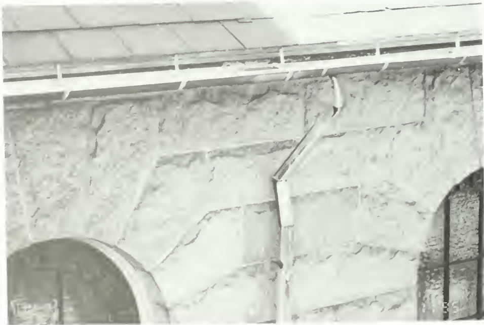
Figure 106. Addition exterior: north wall, gutter and downspout.
