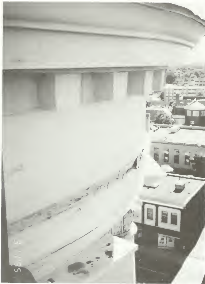
Figure 91. Tower exterior: belfry, modillioned cornice.
