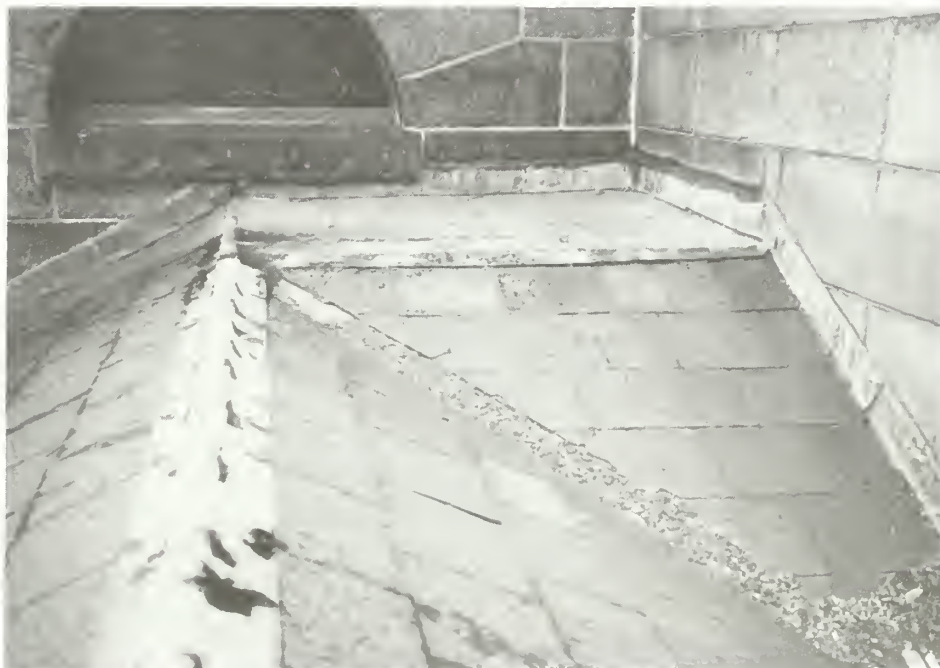
Figure 100. Addition exterior: intersection of north wall with church, showing roof of north porch and lunette window. Note bituminous patches on copper ridge cap and slate roof, clogged valleys, and peeling paint and open joints of window.
