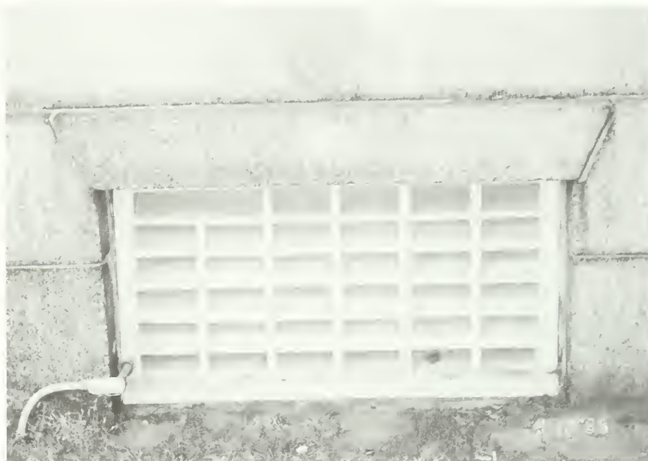
Figure 89. Church exterior: north wall, basement window (W016), showing sash replaced with metal furnace room ventilation panel. Note that grade is above sill level.
