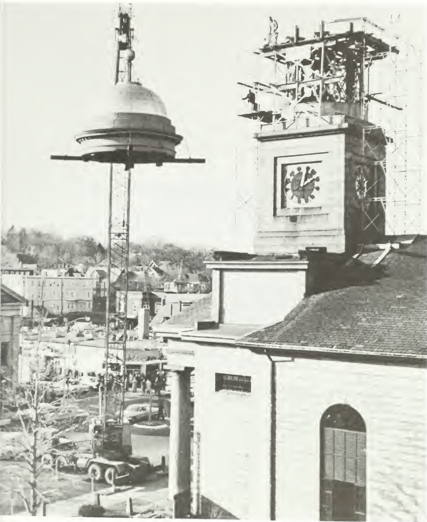
Figure 48. Belfry repairs and dome removal (photograph ca. 1964).
