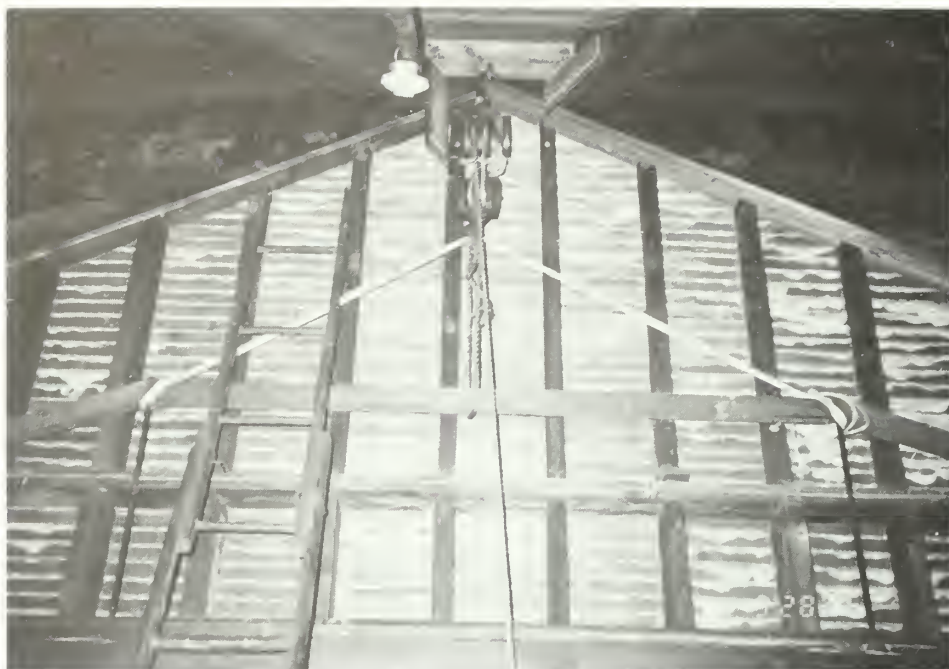
Figure 65. Addition interior: attic (Room 205), west wall and pulley system for lowering partition wall.
