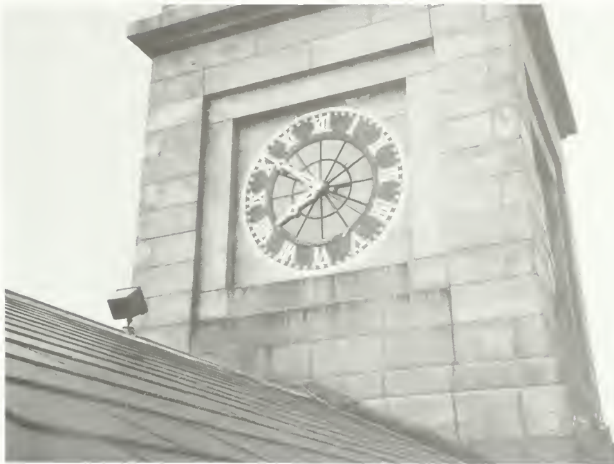
Figure 95. Tower exterior: shaft, east side with glazed clock face. Note open joints and stained granite, and spotlight attached to copper ridge cap.
