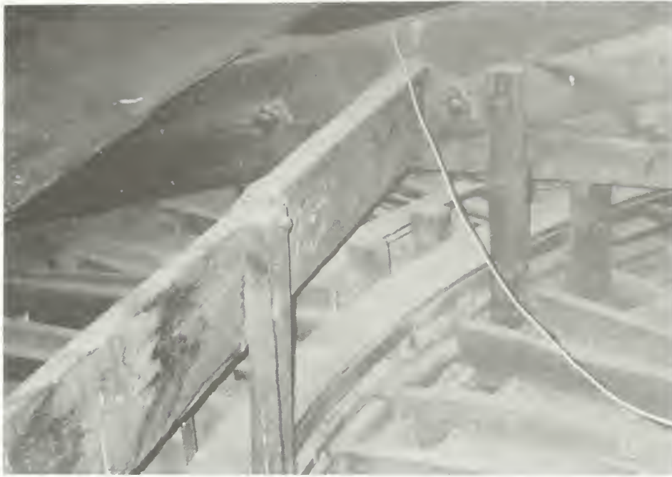
Figure 109. Church interior: attic, view of framing of sanctuary's coffered ceiling dome. Note scissors truss and water stains from roof leaks on many of the wooden elements.
