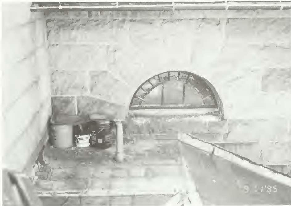
Figure 99. Addition exterior: intersection of south wall with church, showing roof of south wing and lunette window. Note surplus supplies left after last repair with bituminous asphalt; window has peeling paint and dry wooden components.
