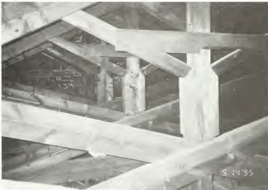
Figure 59. Church interior: attic, eastward view of scissor trusses.
