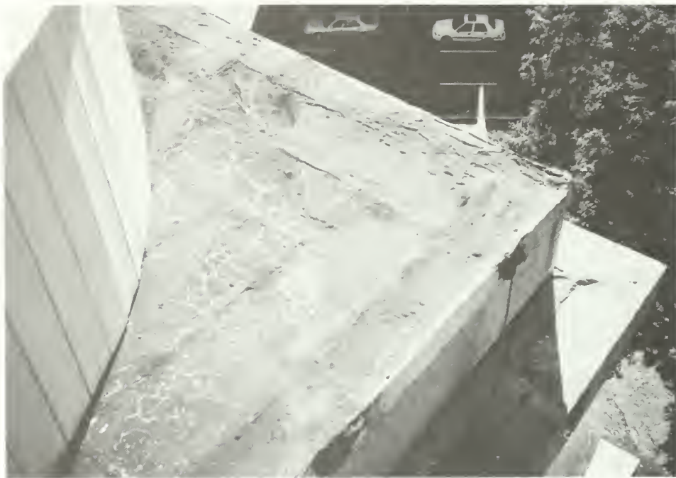
Figure 93. Tower exterior: belfry drum and roof of shaft at southwest corner. Roof of bituminous asphalt over flat-seam copper now weathered, dry, and brittle.
