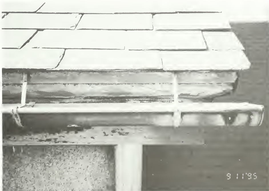
Figure 76. Church exterior: southeast corner of the roof, showing hanging half-round copper gutter with oxidation and pitting, and peeling paint and open joints of the wooden cornice moldings.
