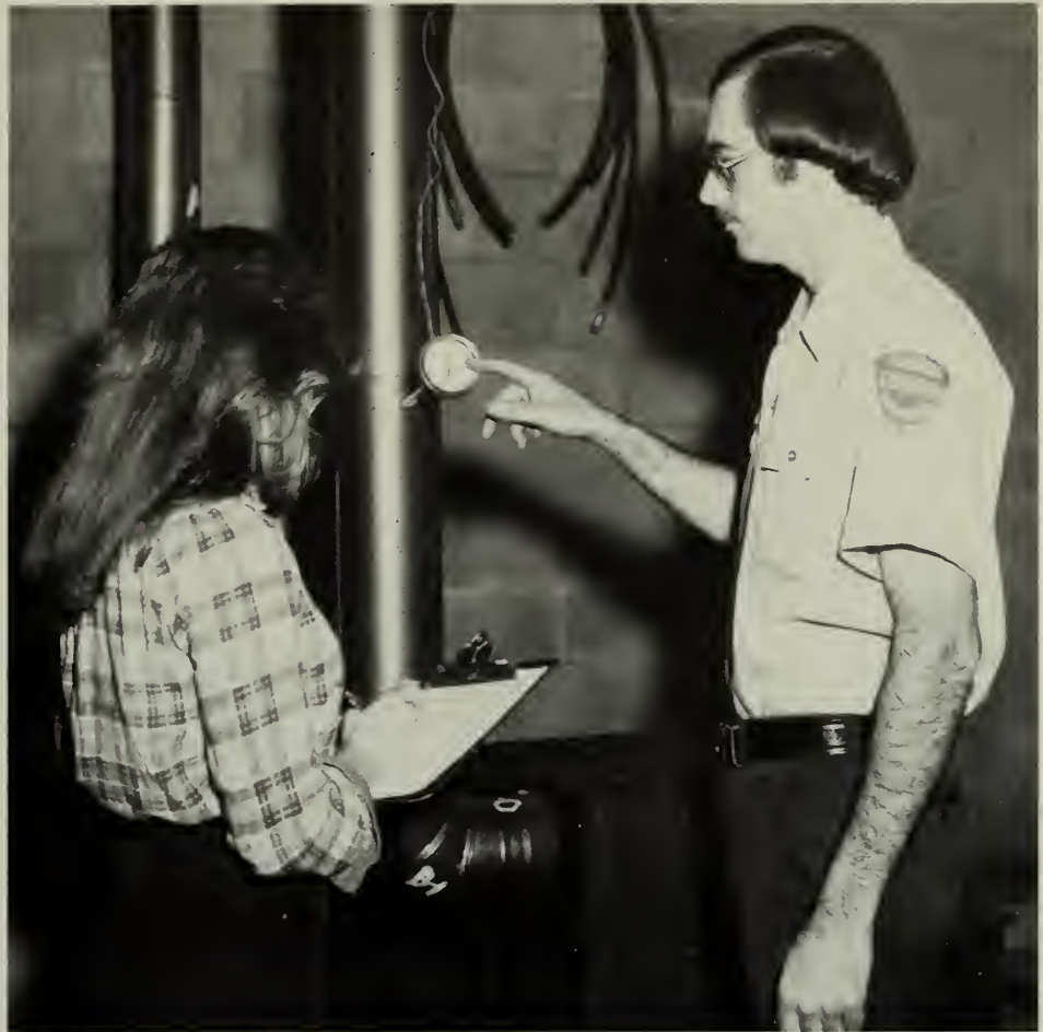
Flue gas temperatures were recorded and air inlets adjusted to maintain temperature between 300-350°F.
