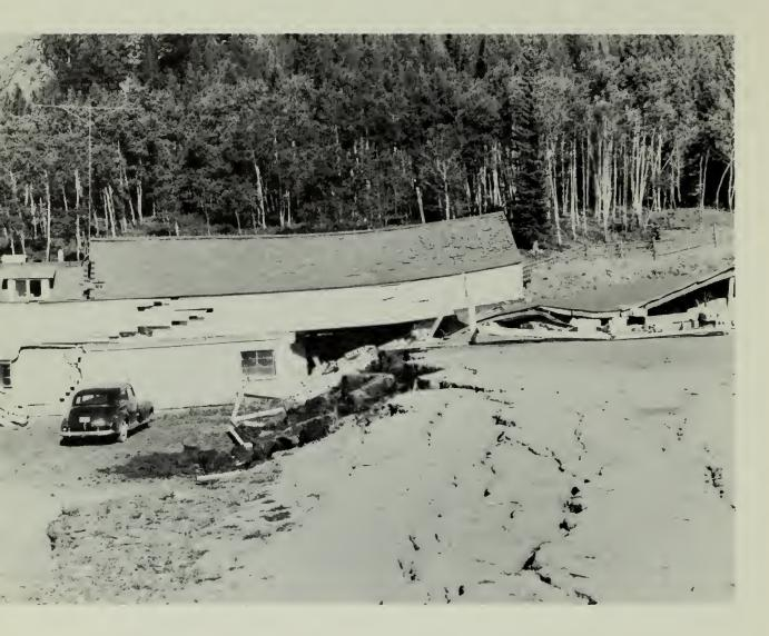
EARTHQUAKE DAMAGE. Severe damage caused by reactivation of a fault during the Hebgen Lake Earthquake of August 17, 1959. The building is on the Blarneystone Ranch, about 10 miles north of West Yellowstone, Montana, and  $1\frac{1}{2}$  miles west of the west boundary of Yellowstone National Park. (Fig. 54)
