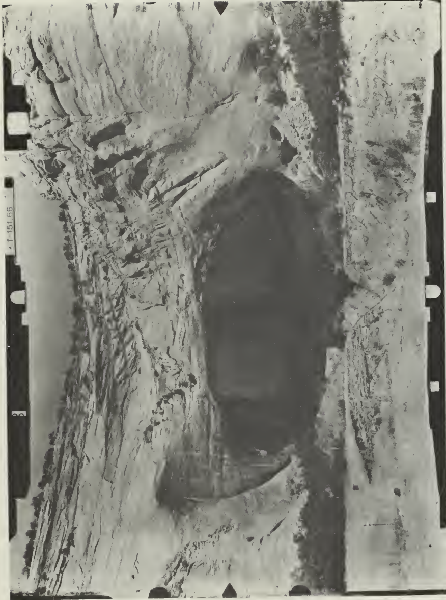
Figure 70 - Right photograph of photogrammetric stereopair of Keel Seal from valley floor approximately 650 ft. in front of cliff opening. Taken with Galileo-Santoni phototheodolite, focal length 151.66 mm, 13 x 18 cm format. Base distance to left camera station 57.21 ft. Camera axis angled upward 15°. Photograph by Perry E. Borchers.
