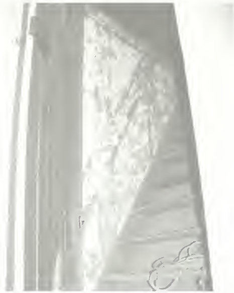
Figure 34 View of timber-framed bousillage construction, whitewashed, visible in stairwell to attic. (NPS-SERO-CRS, 2001)
