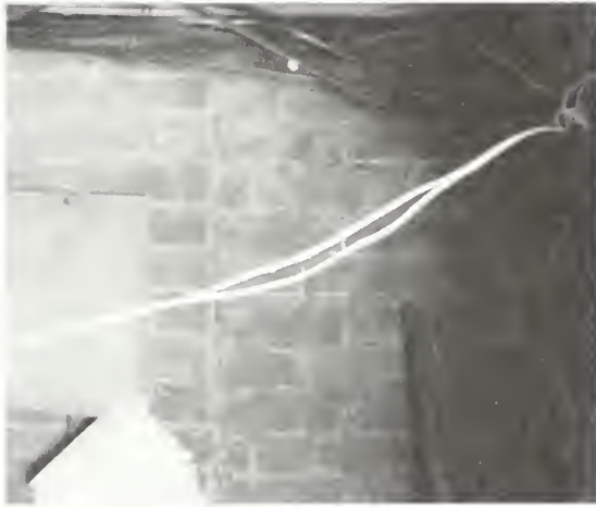
Figure 33 Detail of north wall of gas room (106), showing two earliest generations of brick work, both with mortar joints pencilled in white over red. (NPS-SERO-CRS, 2001)
