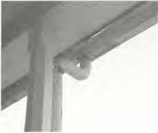
Figure 36 Typical semi-octagonal gutter and round downspouts, which date to early twentieth century. (NPS-SERO-CRS, 2001)
