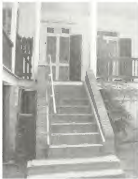
Figure 44 Brick stairs to rear gallery, shown here, and similar stairs to the south gallery replaced wooden stairs after World War II. Brick stairs to front gallery date to the nineteenth century. (NPS-SERO-CRS, 2001)
