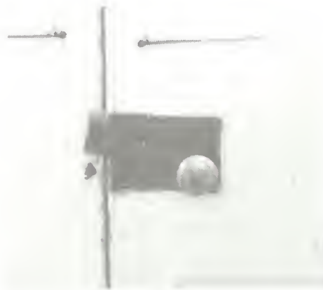
Figure 53 Early spring lock on French doors in dining room. (NPS-SERO-CRS, 2001)
