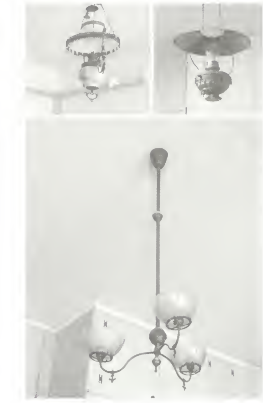
Figure 112 Top, view of nineteenth-century kerosene light fixtures and, below early twentieth-century gas light fixtures, all of which were converted to electricity in the late 1930s.
