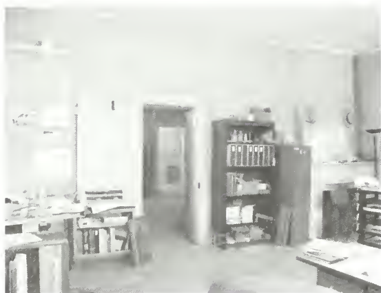
Figure 68 View northeast in master bedroom, showing door to dining room. The line of the back wall of the original house can be identified in the change in materials that is visible along the right edge of this opening. (NPS-SERO-CRS, 2001)
