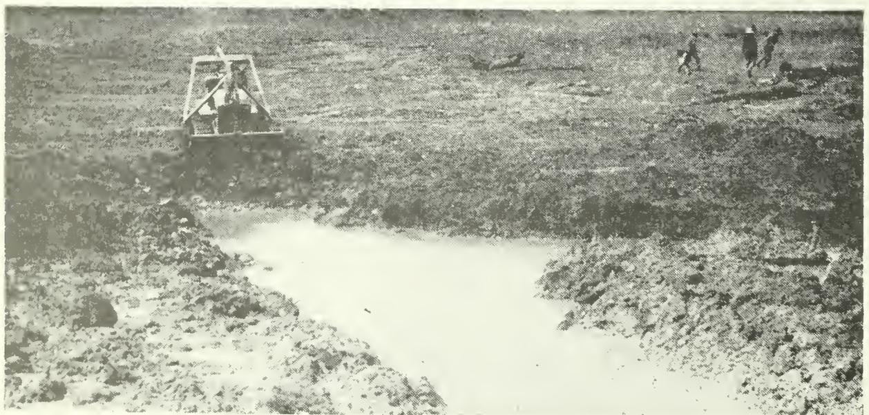
All undesirable materials have been blasted from trench in the boggy area. The tractor is now starting to cut the trench on the hillside. This good clay is used to fill the trench across the bottom.
