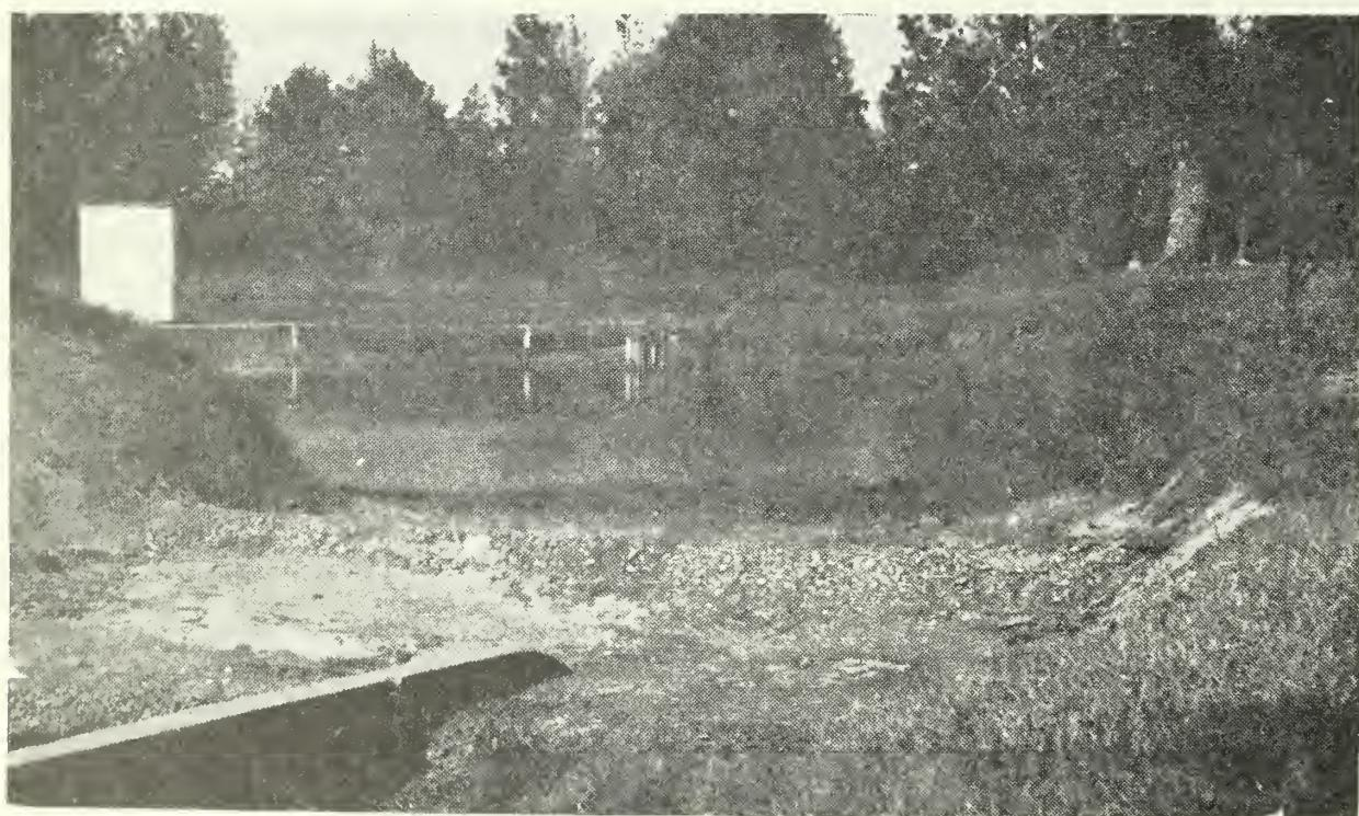
This concrete spillway for a 1.3-acre pond has a low wall across it to obtain desired water level in the pond. The entire floor is paved to prevent erosion and the end of dam is faced with concrete to prevent flood water damage.
