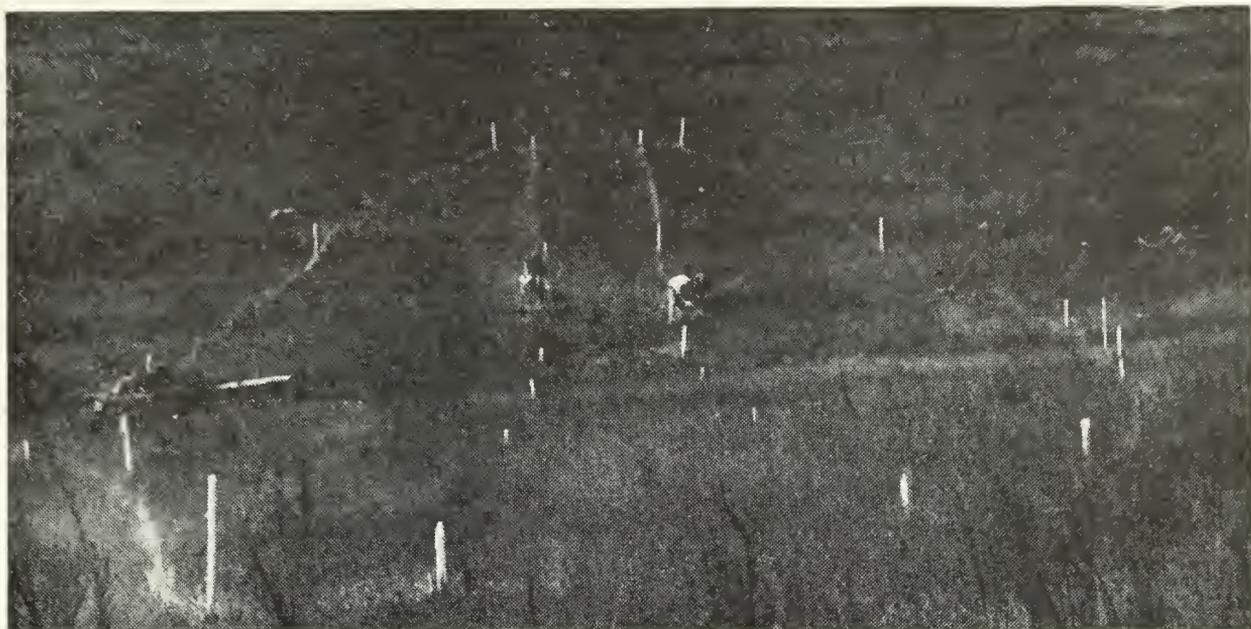
—In the layout of proposed base of dam shown here, the two straight lines of stakes across the hollow outline the width of top of the dam when it is completed. The outside rows of stakes (toe-stakes) outline the area that the base of the dam will cover.
