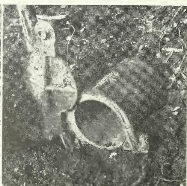
The brass-fitted gate valve at left is being set into place over the pond end of an asbestos-cement drain pipe. Shown at the right is a brass-fitted shear gate valve. The wedges hold the flap tightly closed.
