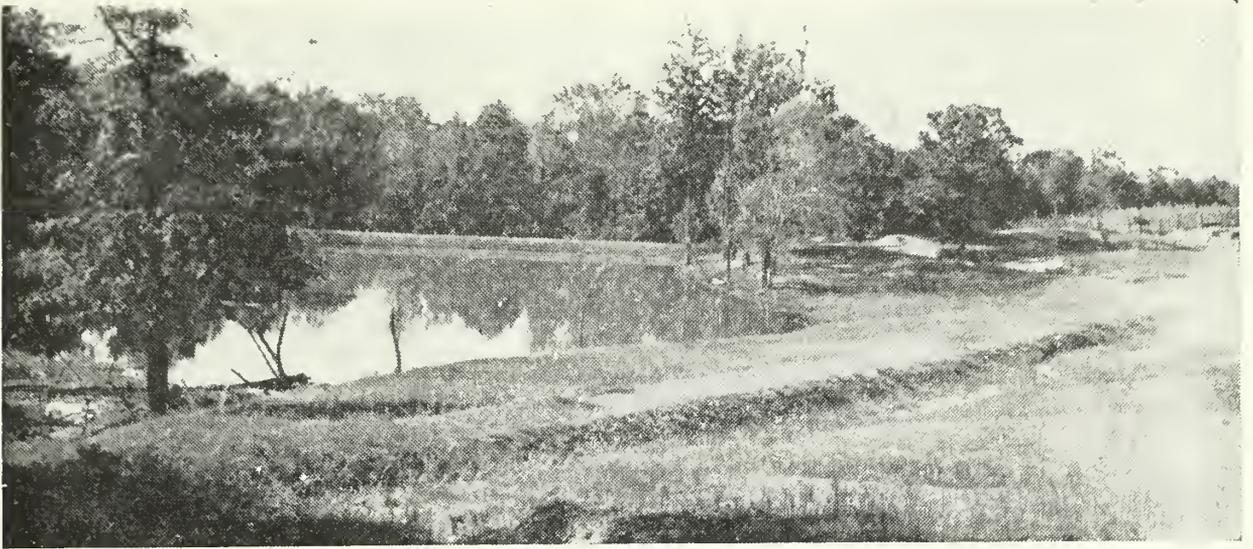
A diversion ditch is built on hillside to by-pass excess water around the pond. This ditch is sodded to prevent erosion.
