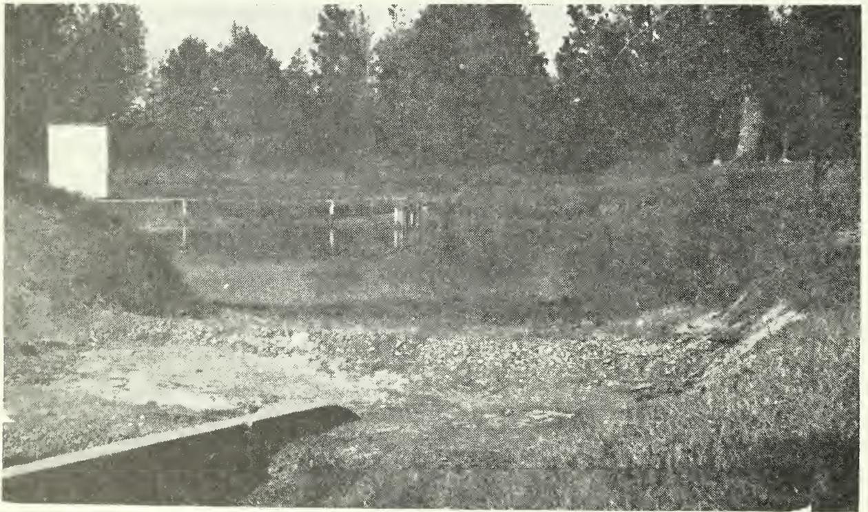
This concrete spillway for a 1.3-acre pond has a low wall across it to obtain desired water level in the pond. The entire floor is paved to prevent erosion and the end of dam is faced with concrete to prevent flood water damage.
