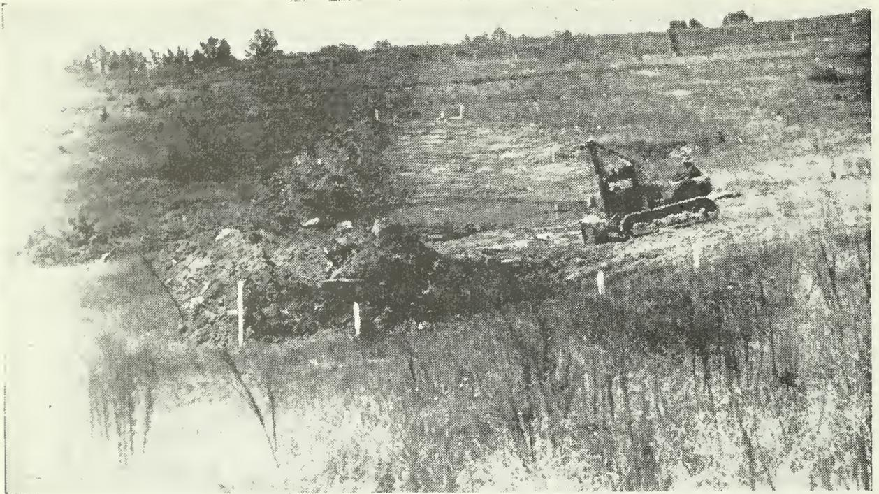
Tractor with bulldozer attachment pushes topsoil from base of the dam to the down stream toe. This operation is done prior to cutting the core trench.
