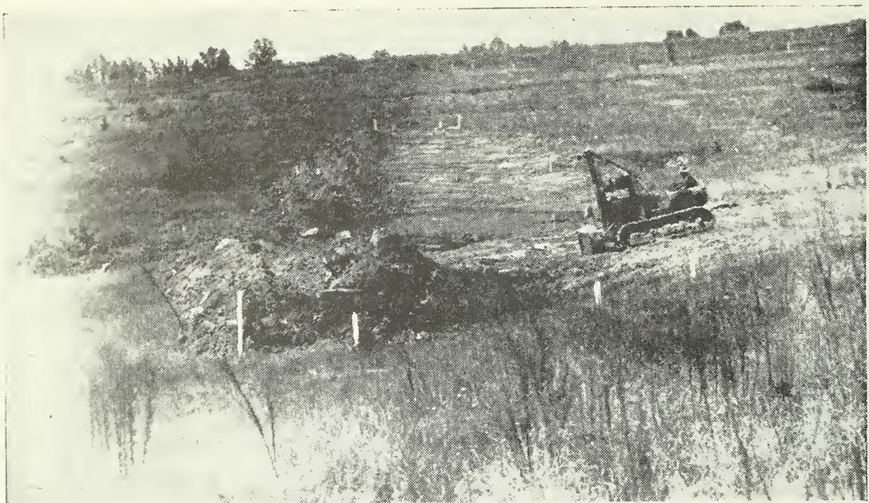
Tractor with bulldozer attachment pushes topsoil from base of the dam to the down stream toe. This operation is done prior to cutting the core trench.
