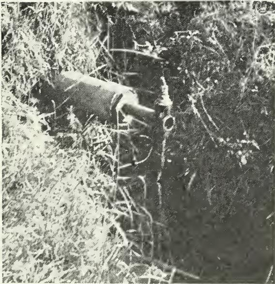
—A pipe with a valve is used for controlling the water entering the pond through the diversion dam.
