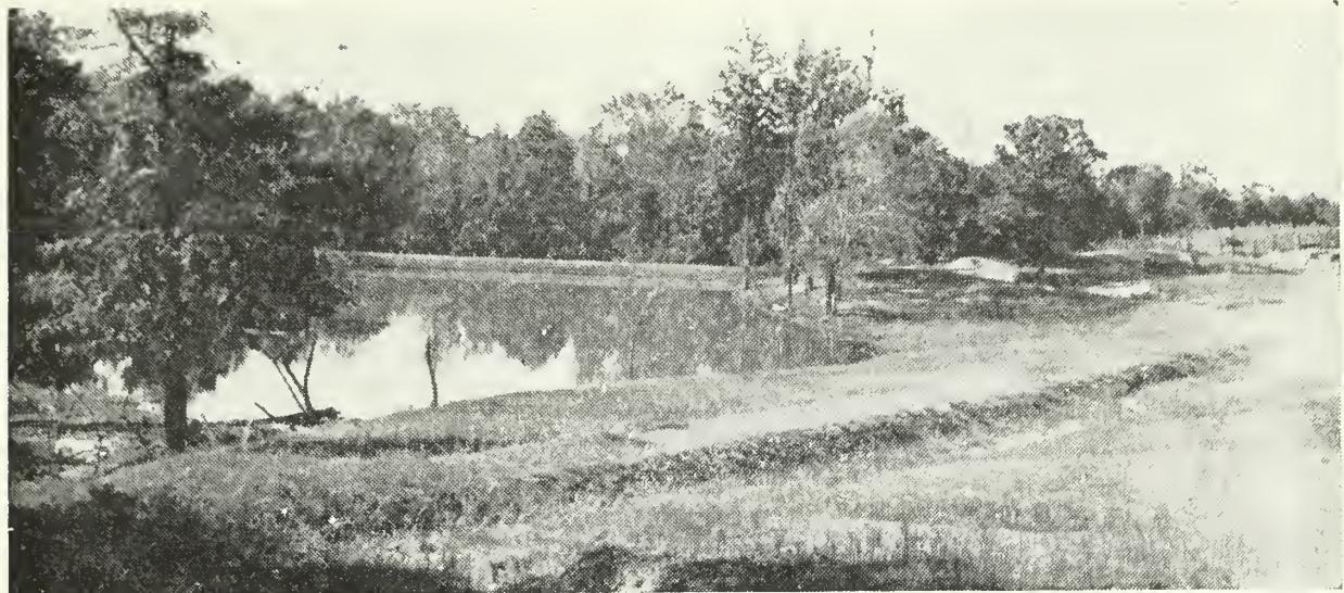
A diversion ditch is built on hillside to by-pass excess water around the pond. This ditch is sodded to prevent erosion.
