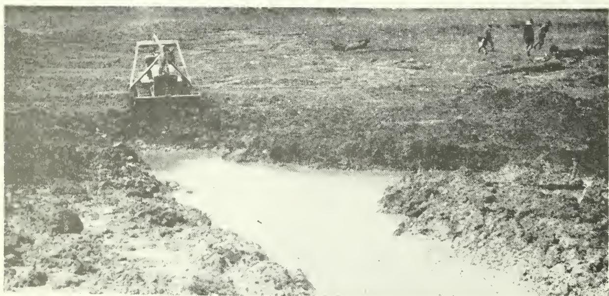
All undesirable materials have been blasted from trench in the boggy area. The tractor is now starting to cut the trench on the hillside. This good clay is used to fill the trench across the bottom.
