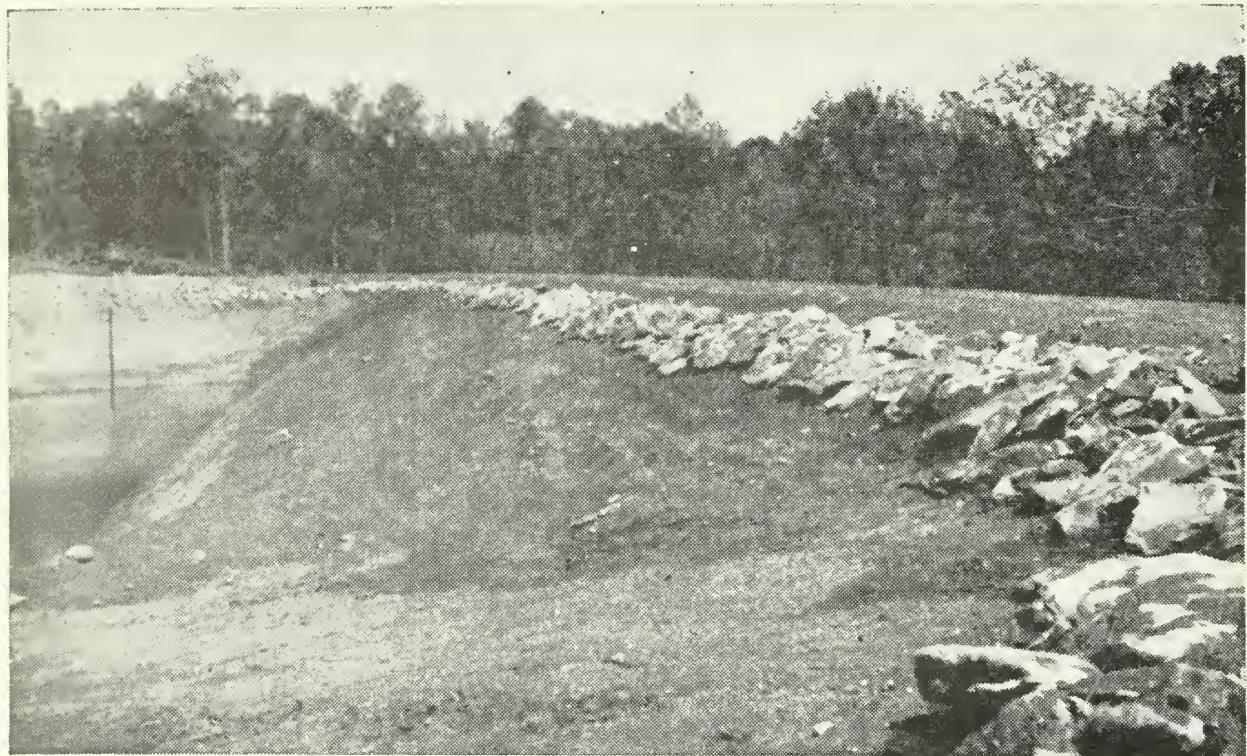
Water line riprapped with rocks 1 foot above and 1 foot below water line.
