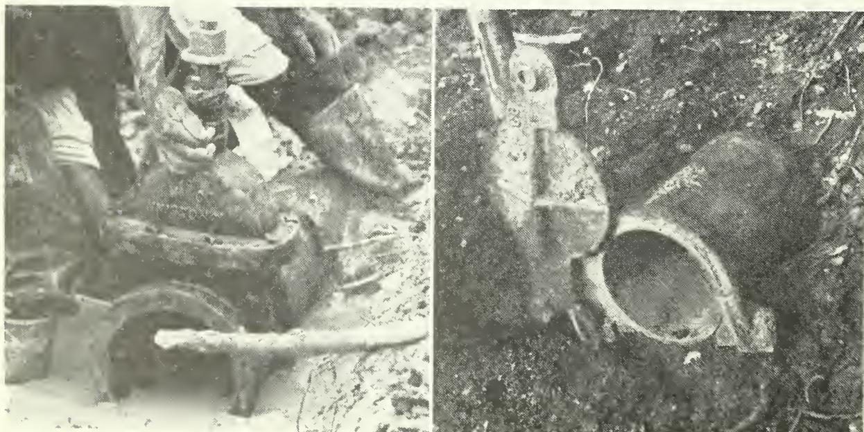
The brass-fitted gate valve at left is being set into place over the pond end of an asbestos-cement drain pipe. Shown at the right is a brass-fitted shear gate valve. The wedges hold the flap tightly closed.
