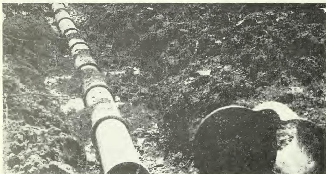
Joints of cast iron soil pipe are laid in the ditch. Here the line is being straightened and held in place with dirt preparatory to caulking and concreting the joints. The flap valve at the right will be placed later in the bell joint of the drain pipe in foreground.
