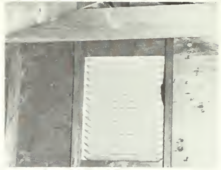
Gable louvre for attic ventilation above the insulation, usually 1/300 of attic floor area.
