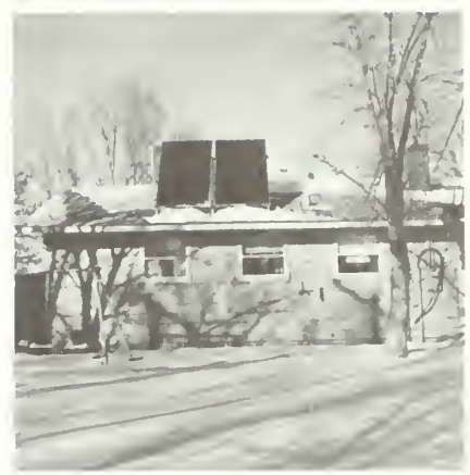
Solar domestic hot water system on residence in Theodore Roosevelt NP (ND).
