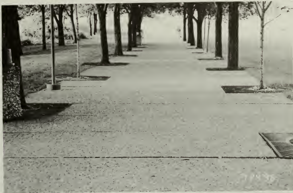
Figure 66: Exposed aggregate sidewalks. (Bellavia, 1996).
