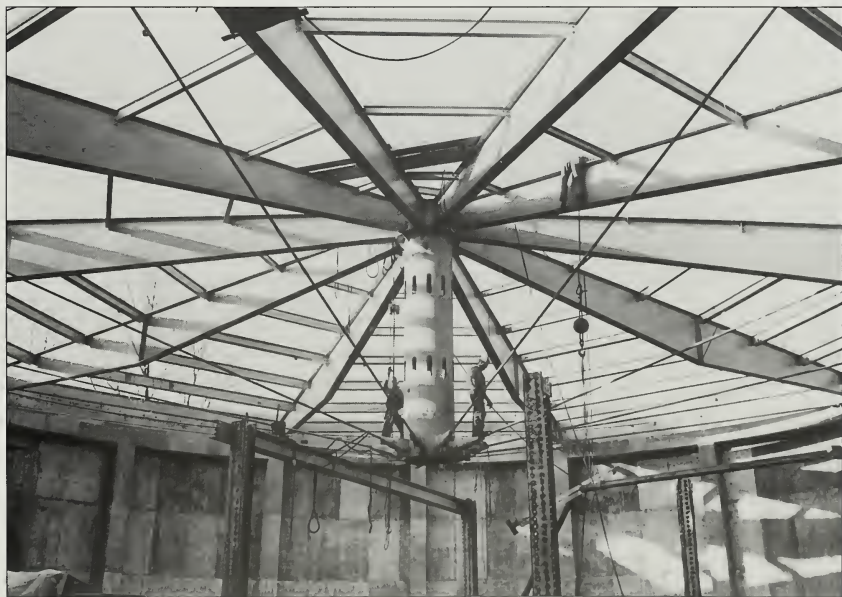
Figure 36. Gettysburg Visitor Center and Cyclorama, view of the roof structure under construction, December 1960. Courtesy National Park Service Technical Information Center, Denver Service Center.
