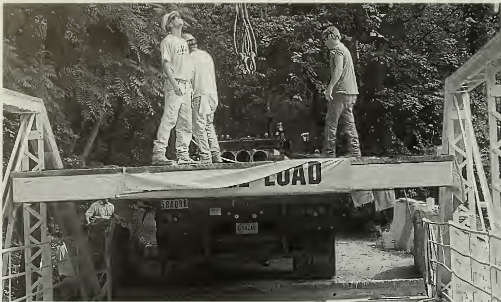
Figure 10. When the deck arrived at the site, the trailer was backed onto the bridge approach and crane cables secured to the deck. Although the road beyond that side of the bridge is a dead end, the truck driver was able to maneuver across a vacant site to get the deck on the opposite side of the creek.
