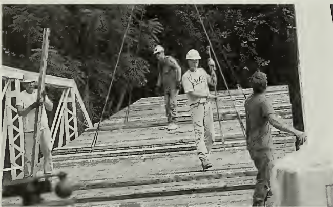
Figure 11. As the deck was lifted off the trailer and onto the floor beams, workers wedged timbers and bars along the sides to prevent the deck from damaging the truss and to help place the deck in position.
