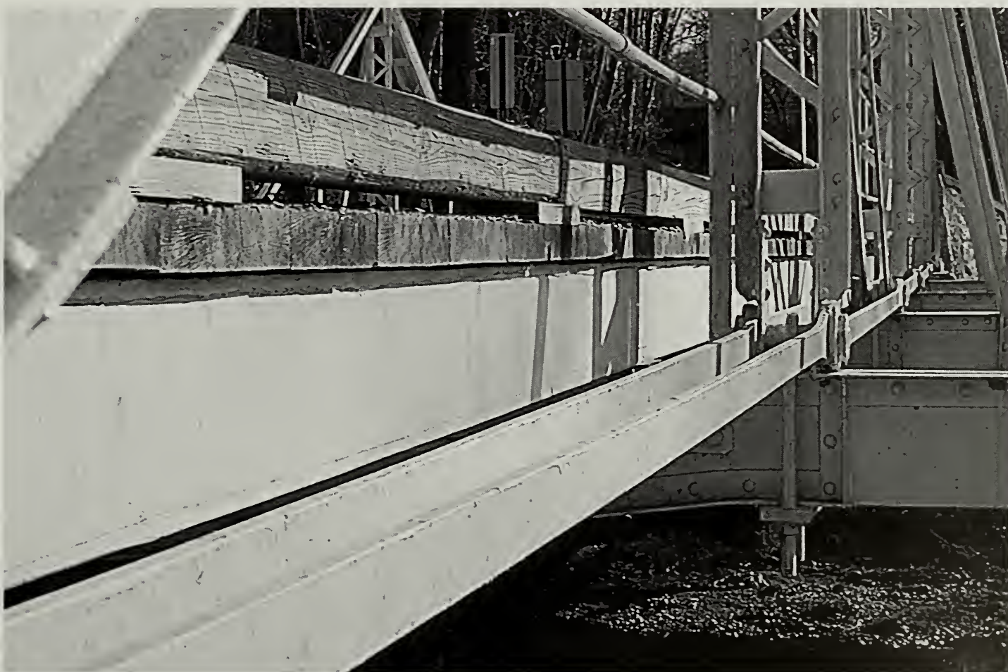
Figure 14. The composite deck, painted to match the superstructure, is visually compatible with the historic bridge as it originally appeared with timber stringers. The new deck and wearing surface are the same thickness as the previous system of steel stringers, nail-laminated deck, and bituminous surface. Photo: Chad Randl.
