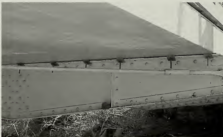
Figure 12. To secure the deck to each floor beam, lag bolts with steel clips were inserted into predrilled holes in the deck surface and fastened tight against the floor beam's upper flange.
