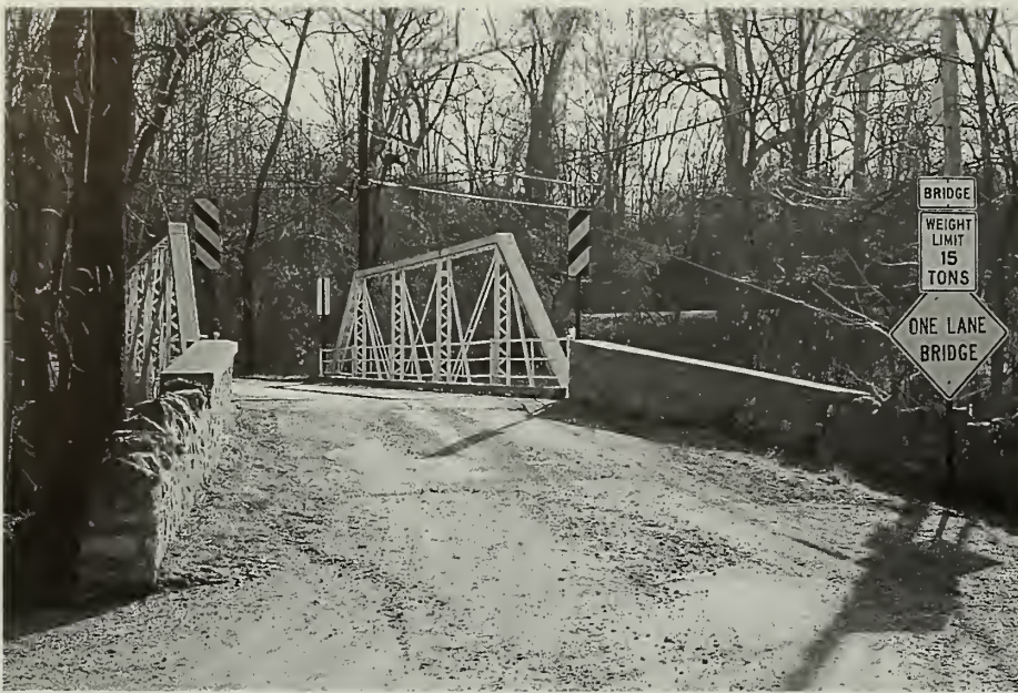
Figure 15. The landscape surrounding Wilson's Bridge has changed little since the span was constructed in the 1800s. The use of a composite deck and plank wearing surface in place of the deteriorated, fourth generation deck was an innovative solution that allowed the bridge to remain in place and in use with little change to its historic character. Photo: Chad Randl.
