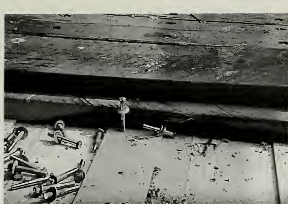
Figure 13. After the deck was locked to the floor beams and the crane cables removed, remaining oak planks that made up the wearing surface were bolted to the composite deck.
