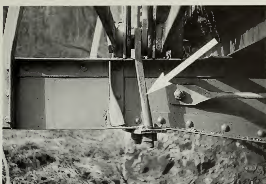
Figure 8. U-bolts connected each of the four floor beams to the superstructure above. Prior to rehabilitation, some bolts, like the one in the photo, showed signs of impact damage. The engineers determined that all of the wrought iron bolts were near the threshold of their stress level and called for replacement with high-strength steel U-bolts of the same dimensions.
