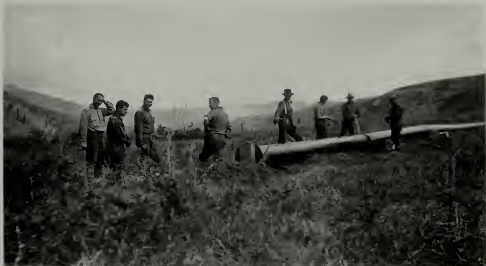
A Kantishna Hydraulic Mining Company crew putting pipe together near Kantishna, 1922.
