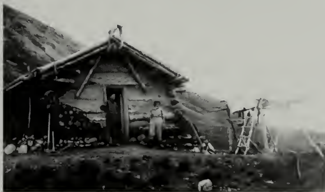
O.M. Grant’s cabin at the base of Copper Mountain, c. 1926. Note the large earthen berms (piled up dirt, sod and rocks) around the base of the cabin and the heavy chinking on the exterior walls. Today, these berms are the only evidence of the Grant cabin. The Herning cabin, which is still standing, was built in front of the remains of this cabin.
