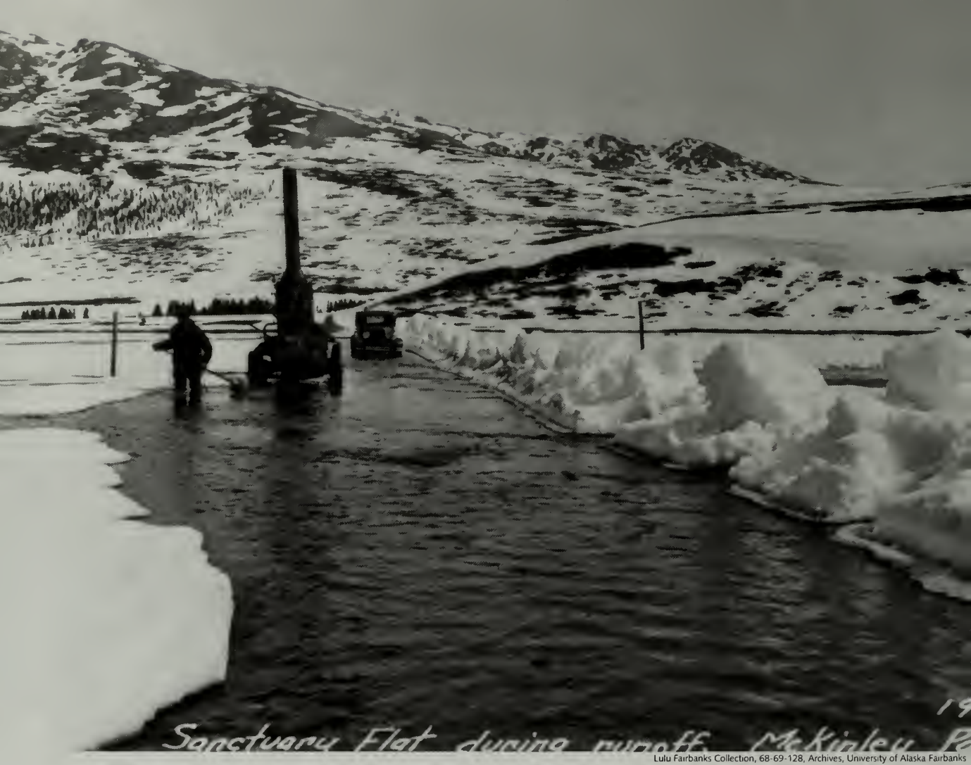
Steaming culverts, spring road opening, 1937.
