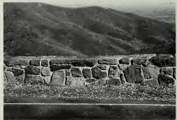
Figure 30, 31: A 75-mile portion of Skyline Drive at Shenandoah National Park overlooking the Blue Ridge Mountains of Virginia required the rehabilitation of a 22"-high, dry-laid stone wall. The new wall was built to a height of 27" – code normally requires a height of 36". The wall was constructed of precast concrete, clad with split stone and mortar joints. To achieve visual compatibility recessed mortar joints were arranged in a random pattern (courtesy Robert R. Page)
