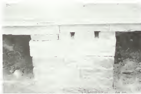
Figure 17 Typical brick foundation pier with original wood blocking. (NPS-SERO-CRS, 2001)
