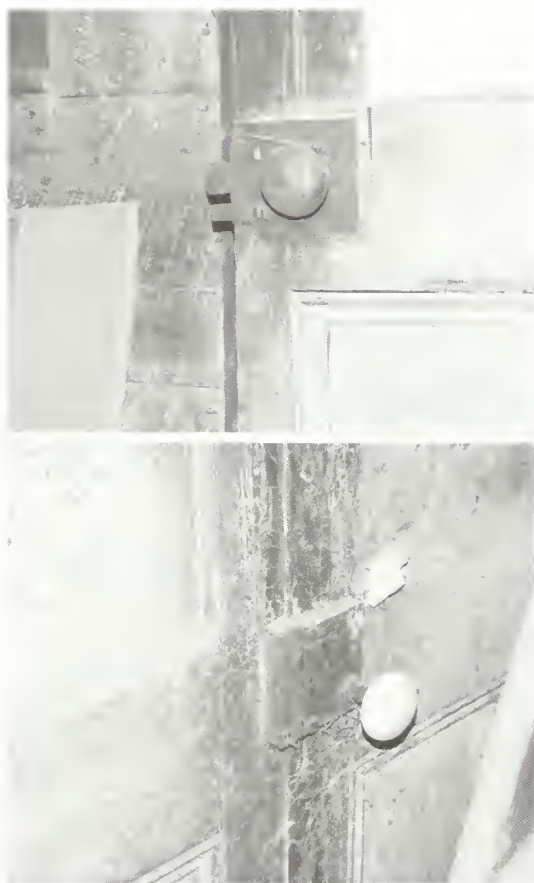
Figure 23 Top, view of spring latch at back door; bottom, view of rim lock with porcelain knob at front door. (NPS-SERO-CRS, 2001)
