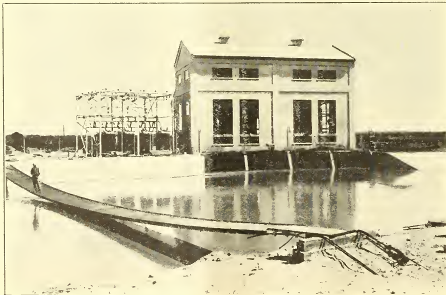
Siphon drop power plant, Yuma project, Ariz.-Calif., showing suspension bridge used for gaging
