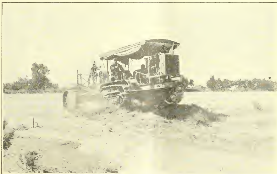
Leveling land with tractor on the Newlands project, Nevada
