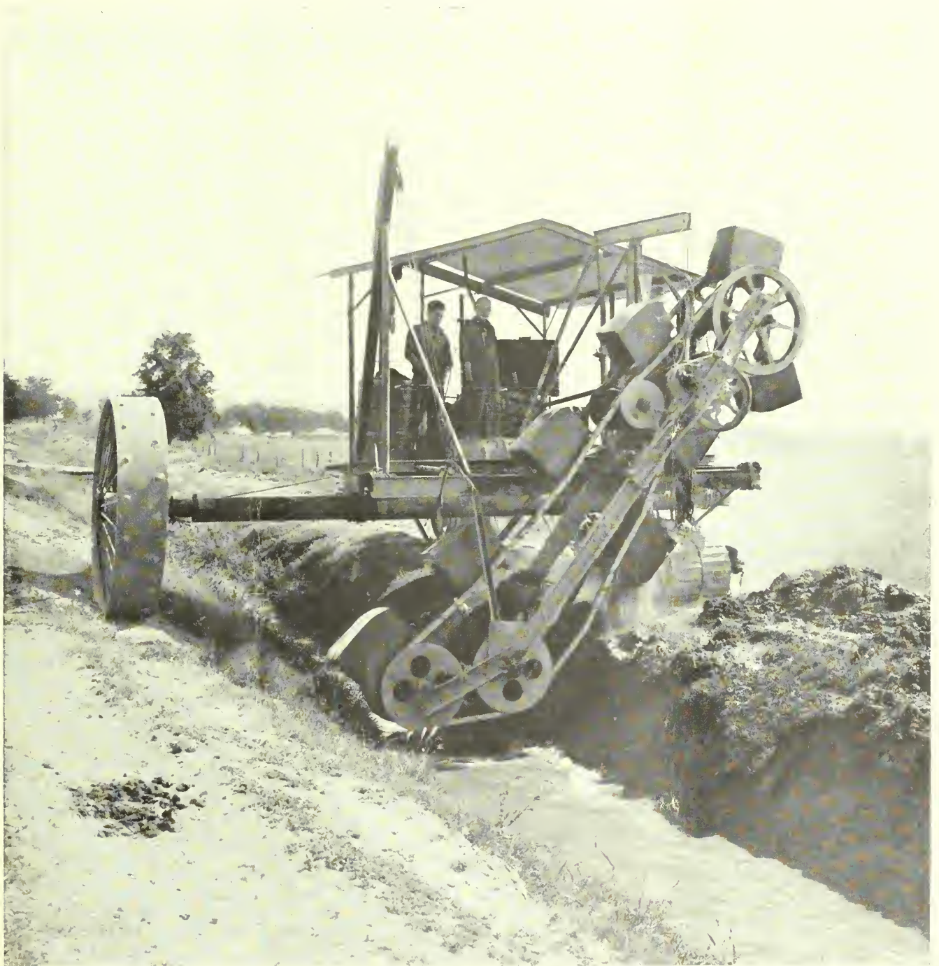
DREDGER CLEANING AN IRRIGATION CANAL
