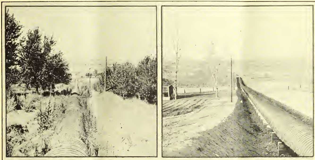
Mabton siphon before and after replacement
