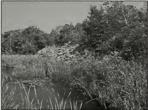
Figure 2.24 This embankment near the ginning of Bureau of Public Roads Project 4A2 is located east of the Beaver Dam Pond and supports the road as it gradually climbs around the northeast slope of Champlain Mountain. (Acad0300_3.431, OCLP 2005)
