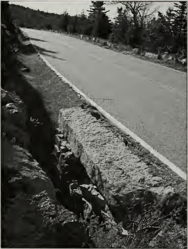
Figure 2.93. There are 25 waterways along Cadillac Mountain Road, and all but two are paved. (Acad0013_2.246, OCLP 2005)
