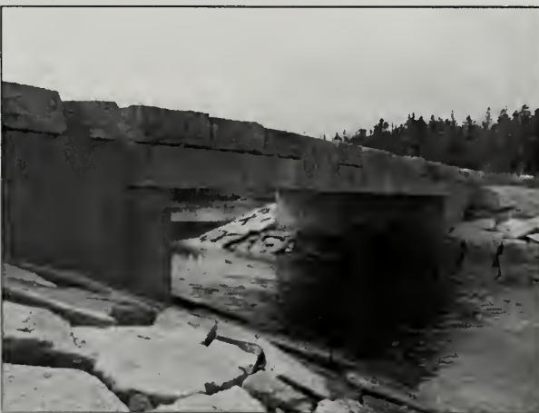
Figure 2.108. The concrete bridge is the only one in the park without a masonry facing. (Acad0301_0.044(1), OCLP 2005)
