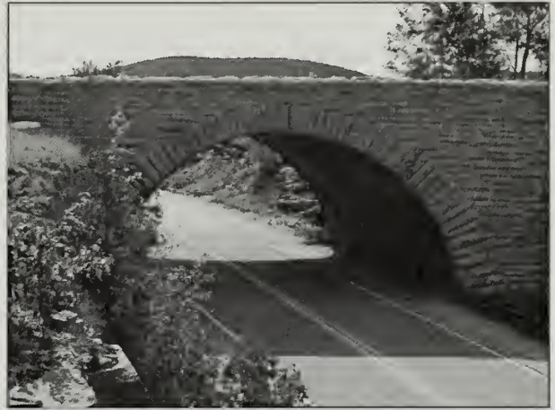
Figure 2.4. This reinforced concrete bridge features masonry facing. It carries Paradise Hill Road over State Route 233. (Acad0010_2.647(2), OCLP 2005)
