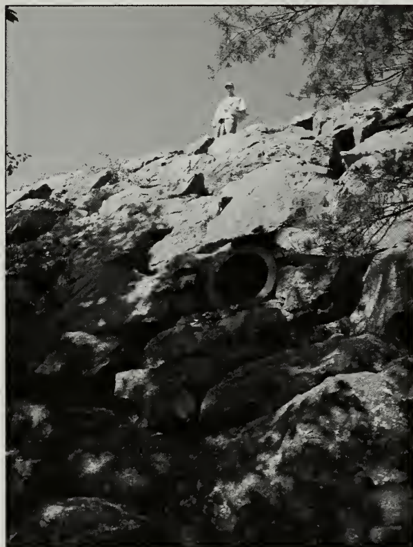
Figure 2.102. Some of the culvert pipe outlets are incorporated into retaining walls. (Acad0010_0.616, OCLP 2005)
