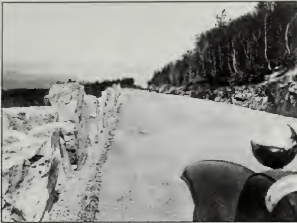
Figure 1.13. Good view of the guardwall stones on Cadillac Mountain Road after completion, in 1932. View looking north. (Acadia National Park archives)
