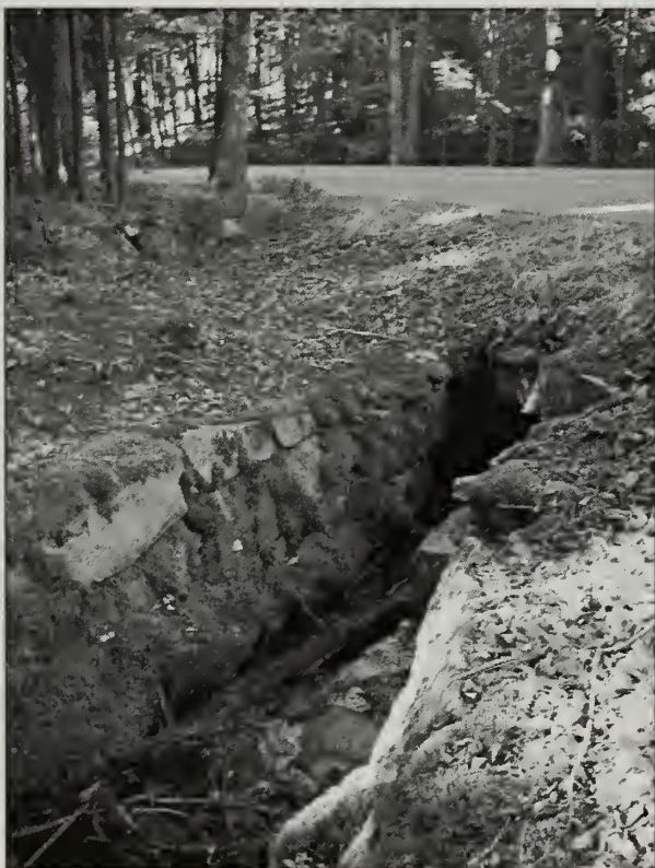
Figure 2.85. There are fifteen stone box culverts along Stanley Brook Road, and some feature stone-lined gutters. (Acad0014_0.162_In, OCLP 2005)
