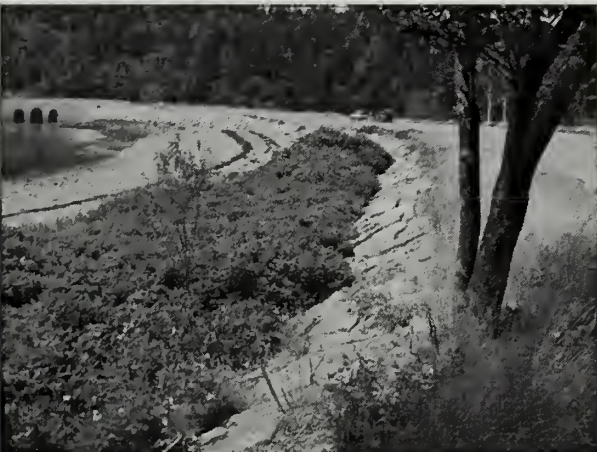
Figure 2.55. The loss of past structures at Otter Cove were the impetus to construct this formidable causeway with riprap embankments. (Acad0300_8.618(3), OCLP 2005)
