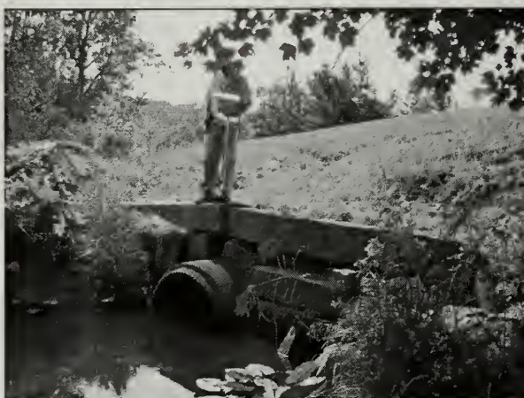
Figure 2.18. Outlet of the 48-inch diameter reinforced concrete pipe culvert along Cromwell Brook that drains Great Meadows and The Tarn. Note the poor condition of the headwall. (Acad0300_2.159_Out(2), OCLP 2005)
