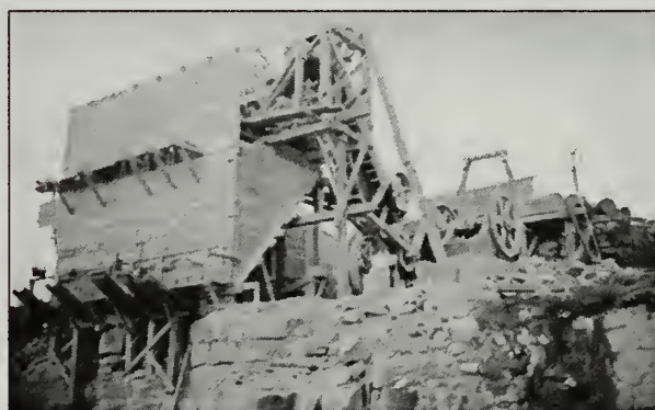
Figure 3.12. Crushing plant and bins used on the construction of Cadillac Mountain Road, July 1931. (Courtesy Leo Grossman Personal Collection, #62-2)
