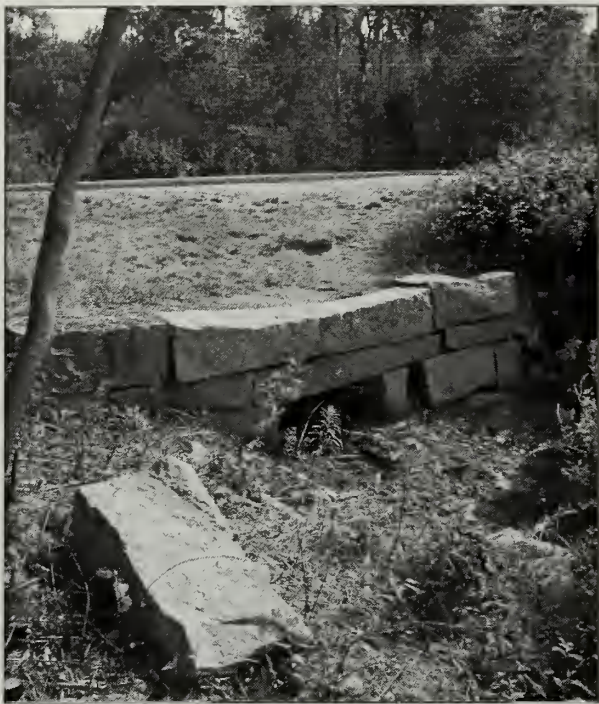
Figure 4.5. The culvert that drains Great Meadow is undersized and often blocked by debris from beaver dams. (Acad0300_2.159_In, OCLP 2005)
