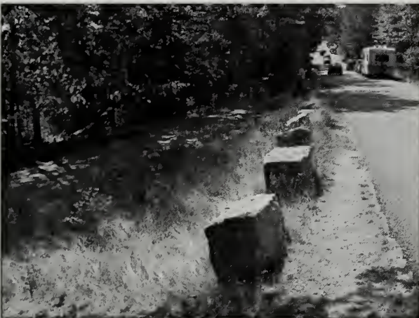
Figure 2.28. At the popular Sand Beach area, this guardwall of rectilinear stone blocks help protect the adjacent path. (Acad0300_5.843, OCLP 2005)
