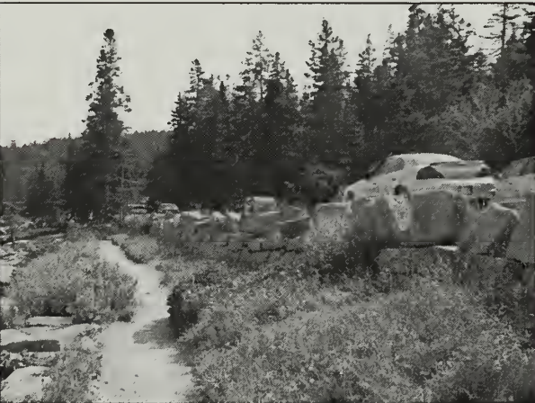
Figure 2.42. This guardwall/retaining wall separates road traffic from foot traffic on the Ocean Path. (Acad0300_7.024, OCLP, 2005)
