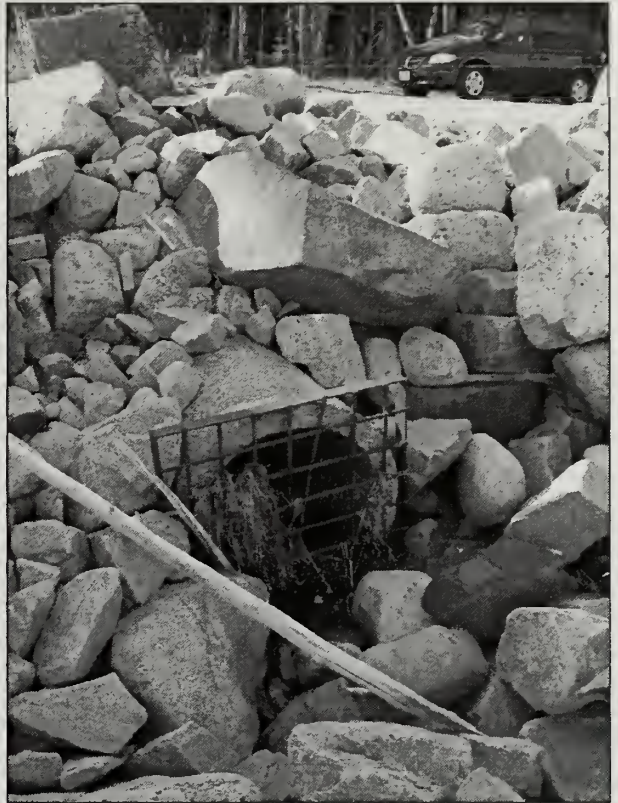
Figure 2.118 Many culvert pipes outlet into the embankment on Schoodic Point Road. (Acad0249_0.176_Out, OCLP 2005)
