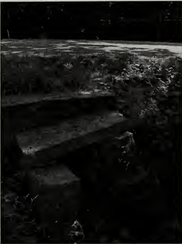
Figure 2.19. One of two dry-laid stone box culverts along the Kebo Mountain Road Extension. (Acad0300_2.306_Out, OCLP 2005)
