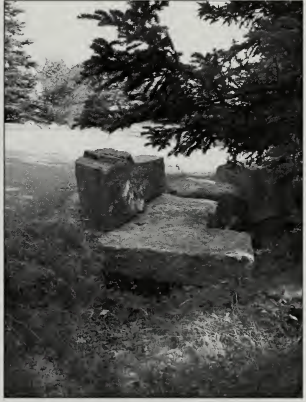
Figure 2.39. View of a dry-laid stone drop-inlet topped by a large coping stone. (Acad0300_6.972_In(2), OCLP 2005)
