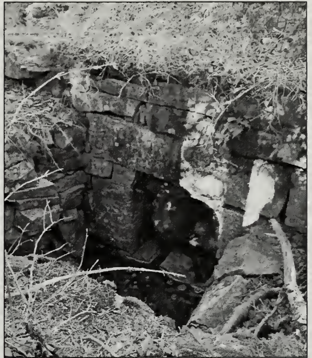
Figure 2.109. View of a large dry-laid stone drop-inlet headwall structure. (Acad0301_4.787_In, OCLP 2005)
