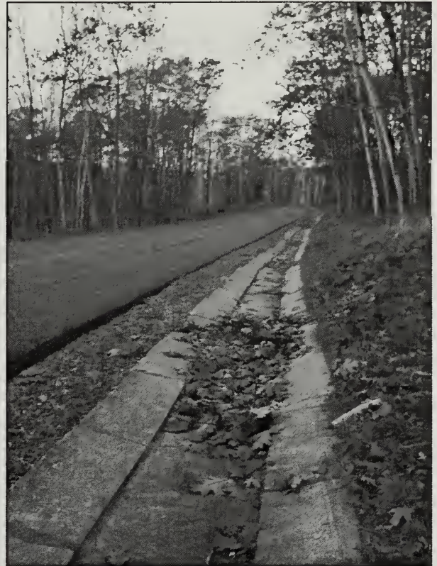
Figure 4.10. A demonstration section of a new mortared rubble waterway was installed off of Schooner Head Overlook Access Road in the mid-1990s. (IMG 0237, OCLP 2005)
