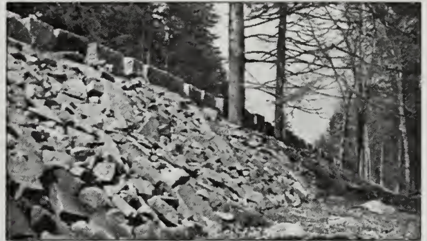
Figure 1.32. Hand-laid stone embankment and rectilinear guardwall stones on Kebo Mountain Road, 1936-1938. Note the preserved trees within the structure. (U.S. Department of Agriculture, Bureau of Public Roads, "Progress Views: Kebo Mountain Project 6A1.")
