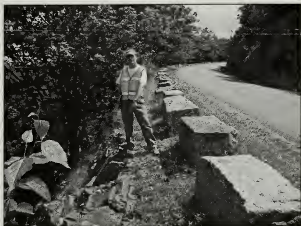
Figure 2.101. On Paradise Hill Road, all of the guardwalls are made of rectilinear quarried block and all of the retaining walls are dry-laid stones. (Acad0010_2.018, OCLP 2005)
