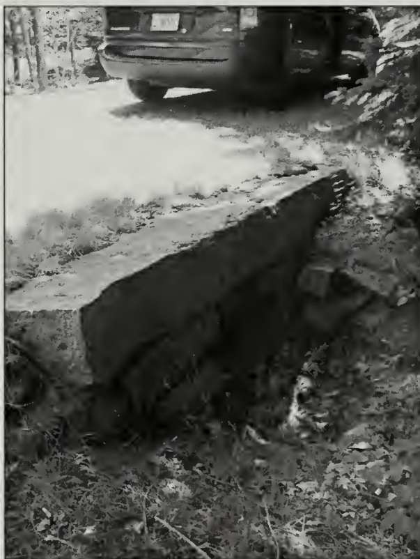
Figure 2.100. Dry-laid stone headwalls are the most common type of inlet on the road's culverts. (Acad0010_1.512_In, OCLP 2005)
