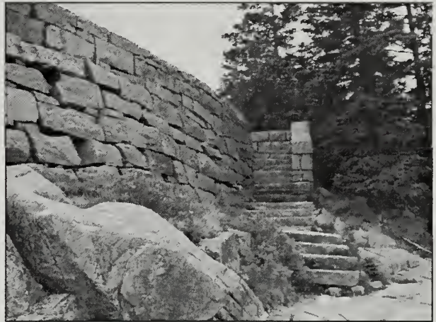
Figure 2.48. View of the outermost guardwall/retaining wall at the grade separation and a set of granite steps. (Acad Otter Cliff Ret Wall, OCLP 1998)
