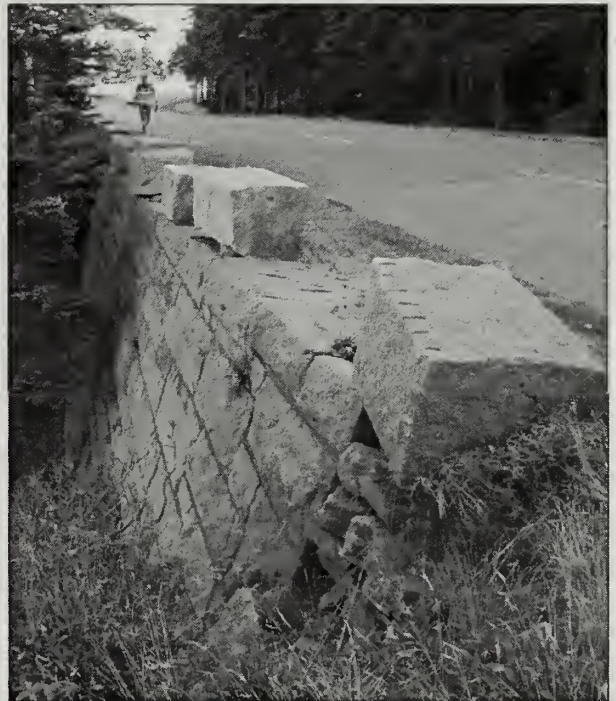
Figure 4.11. Some of the guardwall stones have fallen down the embankments or have become skewed, as seen in this photograph near Western Point on the Otter Cove Causeway and Blackwoods Road. (Acad0300_9.701(2), OCLP 2006)
