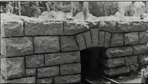
Figure 3.22. View of a headwall under construction on Day Mountain Road, 1941. Notice the tracks used to haul materials through the culvert. (Federal Works Agency, Public Roads Administration, "Progress Views of Structures: Day Mountain Road, Project 9A1.")
