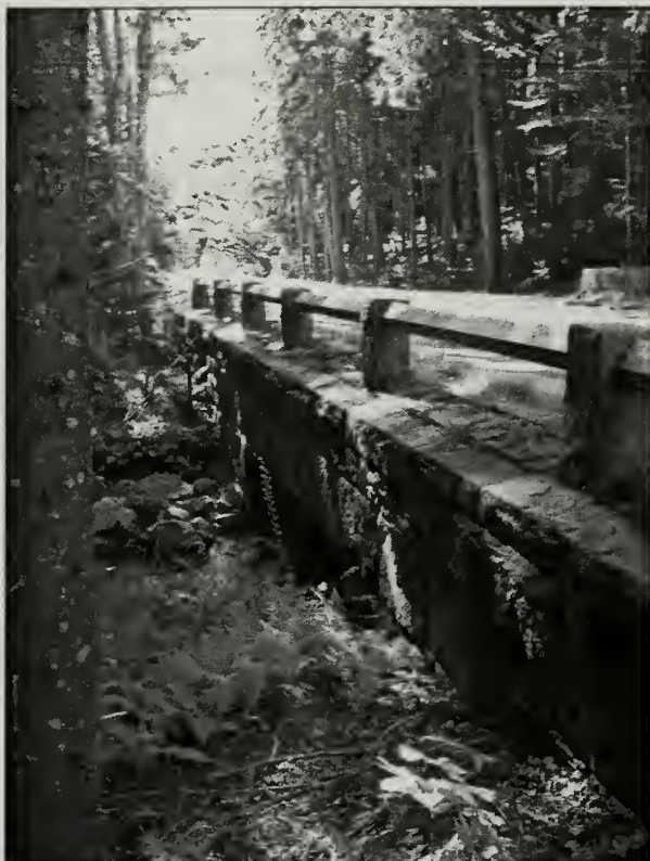
Figure 2.84. Four of the bridges on Stanley Brook Road feature wood guardrails supported by stone piers. (Acad0014_0.940(4), OCLP 2005)
