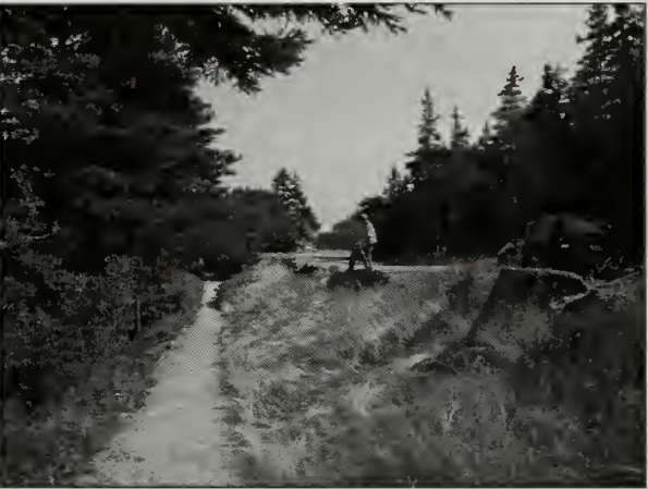
Figure 2.41. A run of angular ledge guardwall stones separates this section of road from the Ocean Path. (Acad0300_6.945(1), OCLP 2005)
