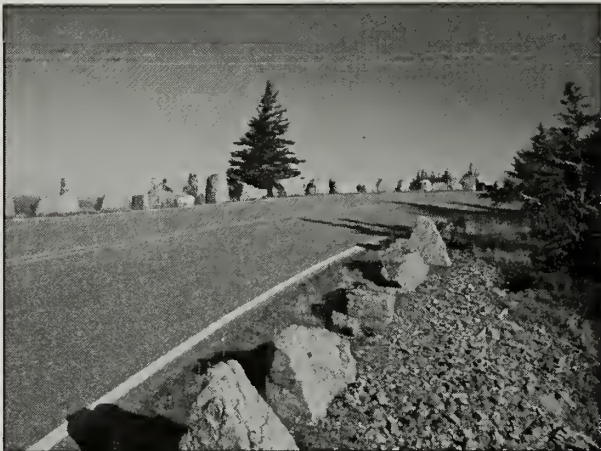
Figure 2.94. The guardwalls along Cadillac Mountain Road feature massive angular stones of pink granite. (Acad0013_1.864(2), OCLP 2005)
