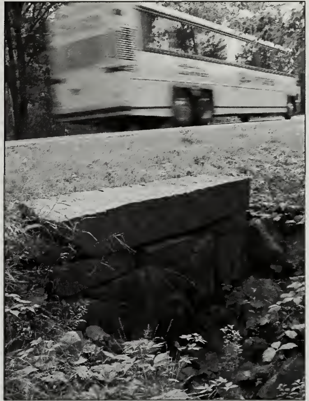
Figure 2.13. Many culvert inlets feature long granite lintel stones. (Acad0300_1.687_In(1), OCLP 2005)
