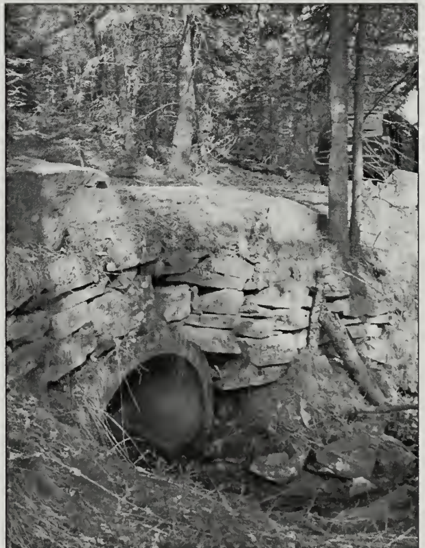
Figure 2.110. The outlet of this 48" pipe features an impressive dry-laid stone headwall. (Acad0301_2.360_Out, OCLP 2005)
