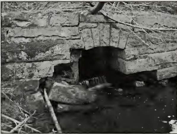
Figure 2.59. The outlet headwall of this concrete box culvert is impressive but is failing. (Acad0300_11.356_Out(2), OCLP 2005)
