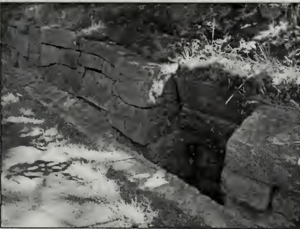
Figure 2.12. Some of the dry-laid stone drop-inlets and mortared waterways are incorporated into dry-laid stone retaining walls. (Acad0300_10.484_In(2), OCLP 2005)
