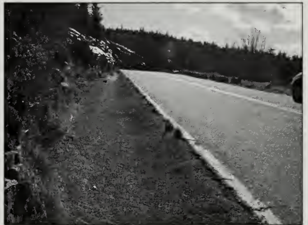
Figure 2.5. Paved waterways on Cadillac Mountain Road have widened its paved cross-section. (Acad0013_2.327, OCLP 2005)
