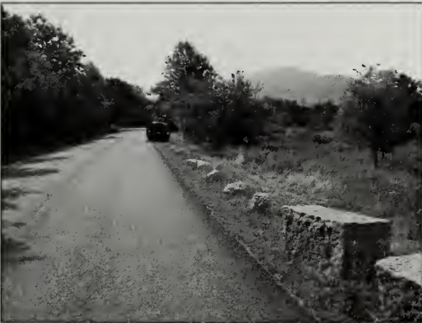
Figure 4.9. View of round parking management stones installed after a run of historic guardwall stones on Kebo Mountain Road Extension. The parking management stones are compatible with the rustic character, yet distinguishable from the historic stones. (Acad0300_1.760, OCLP 2005)
