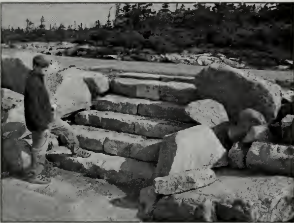
Figure 2.116. One of six sets of tooled stone steps that connect the three parking levels at the end of Schoodic Point Road. (Acad0249_0.513, OCLP 2005)
