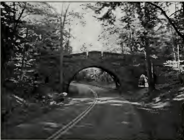
Figure 2.80. Stanley Brook Road passes under the Stanley Brook Bridge, a three portal structure built in 1933 to accommodate, the road, stream, a carriage road, and a trail. (IMG0010, OCLP 2005)
