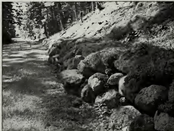
Figure 2.86. The retaining walls along Stanley Brook Road feature dry-laid uncoursed stone. (Acad0014_0.711(3), OCLP 2005)
