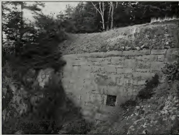
Figure 2.63. Mortared stone retaining wall along Blackwoods Road. (Acad0300_10.175(1), OCLP 2005)
