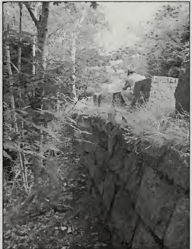
Figure 2.14. Of the four retaining walls along the road, only this one is mortared stone. (Acad0300_1.130, OCLP 2005)
