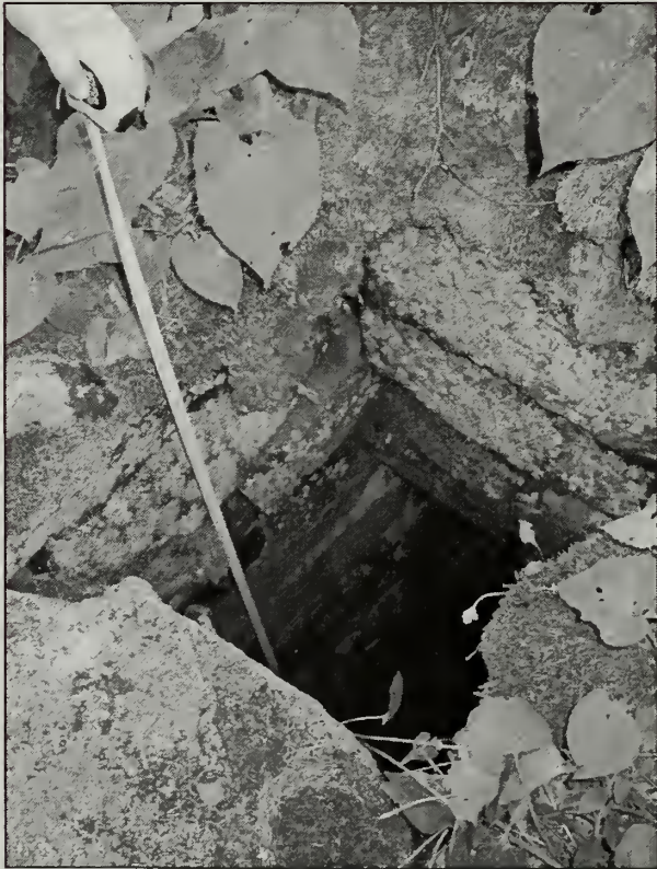
Figure 2.44. This dry-laid stone drop-inlet near the former Naval Station is over eight feet deep. (Acad0300_8.130_In(3), OCLP 2005)
