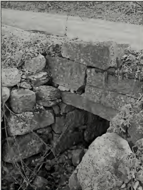
Figure 2.90. Outlet headwalls of a dry-laid stone box culvert at the bottom of the road. (Acad0013_0.160_Out(2), OCLP 2005)
