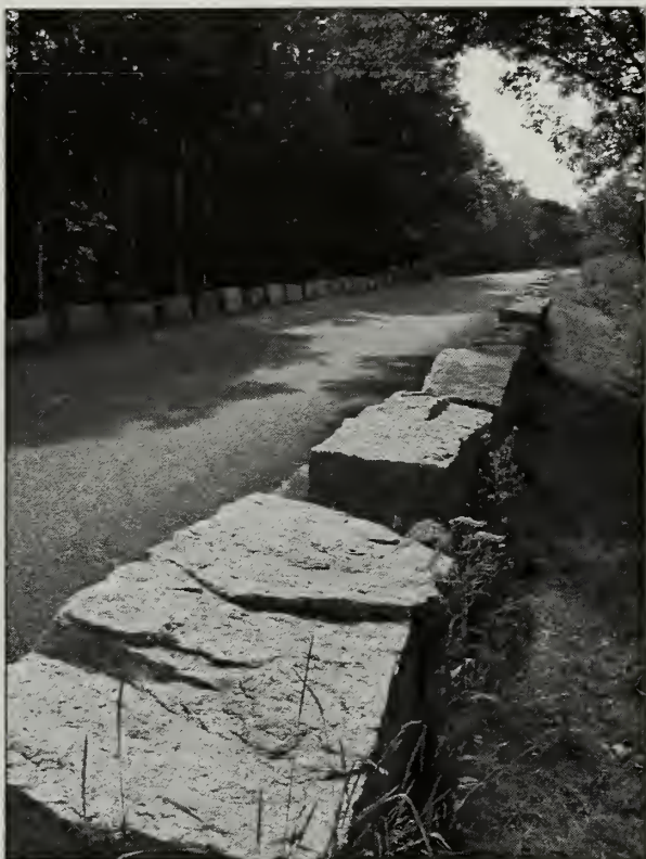
Figure 2.15. Guardwalls along Kebo Mountain Road feature rectilinear quarried blocks similar to those on Cadillac Mountain Road. (Acad0300_1.723(2), OCLP 2005)
