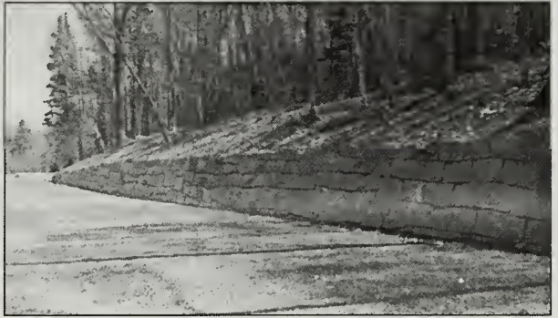
Figure 1.31. Dry-laid retaining wall on Kebo Mountain Road, 1936-1938. (U.S. Department of Agriculture, Bureau of Public Roads, "Progress Views: Kebo Mountain Project 6A1.")
