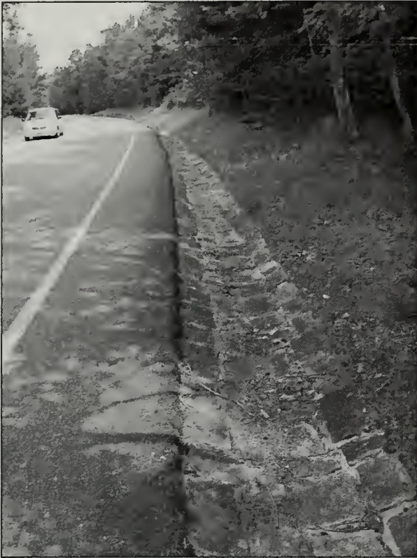
Figure 2.79. Mortared rubble waterways along the Jordan Pond/Eagle Lake Road can be found in the section that was completed in 1924. (Acad0012_4.801, OCLP 2005)
