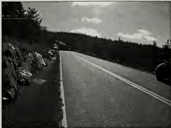
Figure 4.6. A wider cross-section, caused by paved shoulders or by paved waterways, as shown here on Cadillac Mountain Road, is a psychological cue for motorists to drive faster. (Acad0013_2.290, OCLP 2005)
