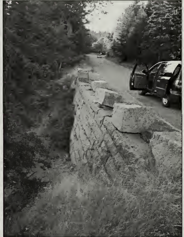
Figure 2.61. Guardwall/retaining wall employing mortared stonework. Note the skewed and missing blocks on top. (Acad0300_10.203(2), OCLP 2005)
