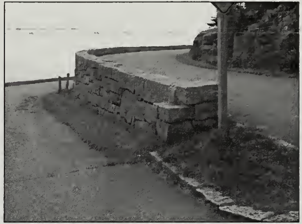
Figure 2.47. The pink granite guardwall/retaining walls at the grade separation blend into the surrounding rock outcrops. (Acad0300_7.452, OCLP 2005)
