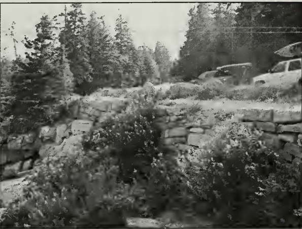
Figure 2.40. This dry-laid stone retaining wall supports both the motor road and the Ocean Path. (Acad0300_7.117, OCLP 2005)
