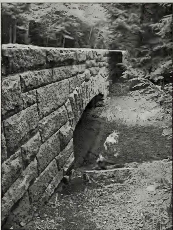
Figure 2.67. This small mortared and stone bridge spans Hunters Brook. (Acad0300_11.500(2), OCLP 2005)
