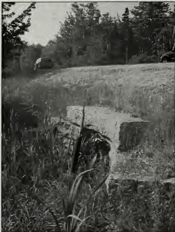
Figure 2.23. Route 4 also features culverts with mortared stone headwalls. This outlet has an interesting curved design. (Acad0300_5.008_Out, OCLP 2005)
