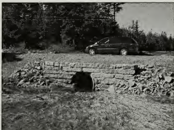
Figure 2.111. This culvert features a mortared stone inlet headwall that drains a perennial stream to West Pond. (Acad0301_2.808_In, OCLP 2005)
