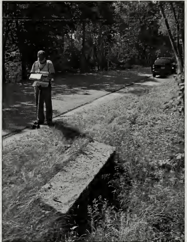
Figure 2.30. Numerous culvert headwalls feature long lintel stones. (Acad0300_5.414_In, OCLP 2005)
