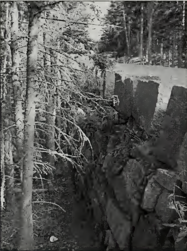
Figure 2.46. Topographic conditions in the Otter Cliff area warranted the construction of numerous guardwalls/retaining walls like this one. (Acad0300_7.301, OCLP 2005)
