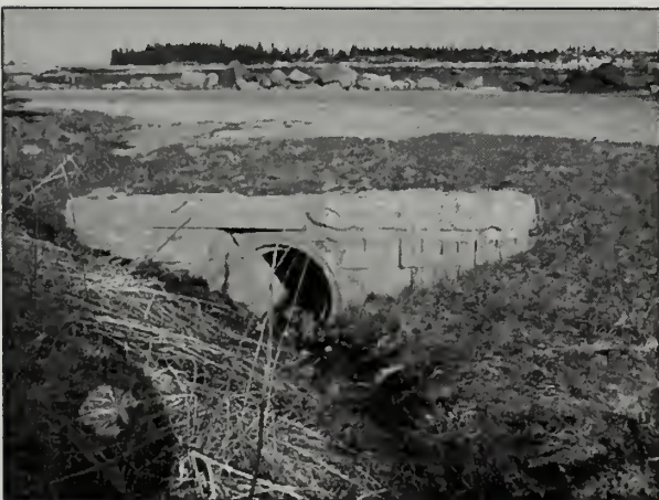
Figure 2.117. Mortared stone inlet headwall on Schoodic Point Road. (Acad0249_0.176_In, OCLP 2005)
