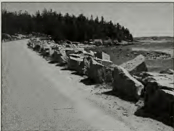
Figure 2.112. Most of the guardwalls along Schoodic Loop Road feature angular ledge stones. (Acad0301_3.333, OCLP 2005)
