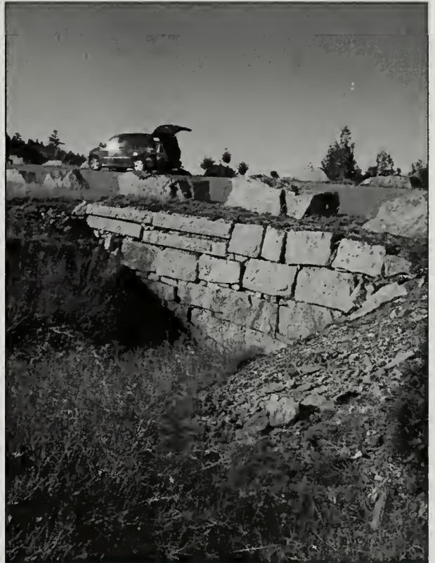
Figure 2.91. Interesting dry-laid stone inlet headwall with two colors of granite. (Acad0013_1.563_In(1), OCLP 2005)
