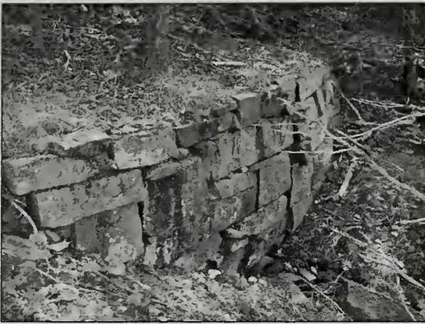
Figure 2.45. The dry-laid stone outlet headwall of the culvert shown in Figure 8.2 is in poor condition because of a severe lean. (Acad0300_8.310_Out(2), OCLP 2005)
