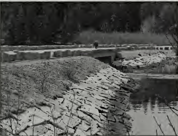
Figure 2.107. Schoodic Loop Road begins as a causeway and bridge. Unlike other guardwalls on the road, these feature rectilinear quarried blocks. (Acad0301_0.008, OCLP 2005)
