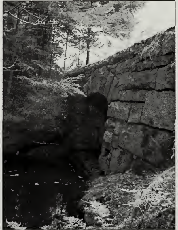
Figure 4.3. The culvert that conveys a perennial stream near the junction of Day Mountain Road Extension, Jordan Pond/Eagle Lake Road, and Stanley Brook Road has been identified by park staff as a possible impediment to fish. (Acad0300_13.227_Out(2), OCLP 2005)
