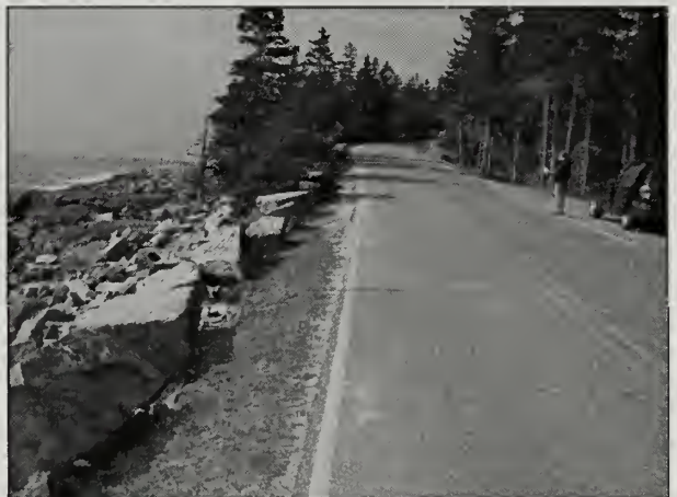
Figure 2.119. View of the embankment and an angular ledge stone guardwall. (Acad0249_0.367, OCLP 2005)
