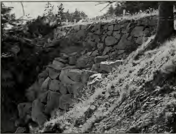
Figure 2.62. Several of the riprap embankments at Western Point have carefully been rebuilt. Note the longer retaining wall above it. (Acad0300_9.799, OCLP 2005)
