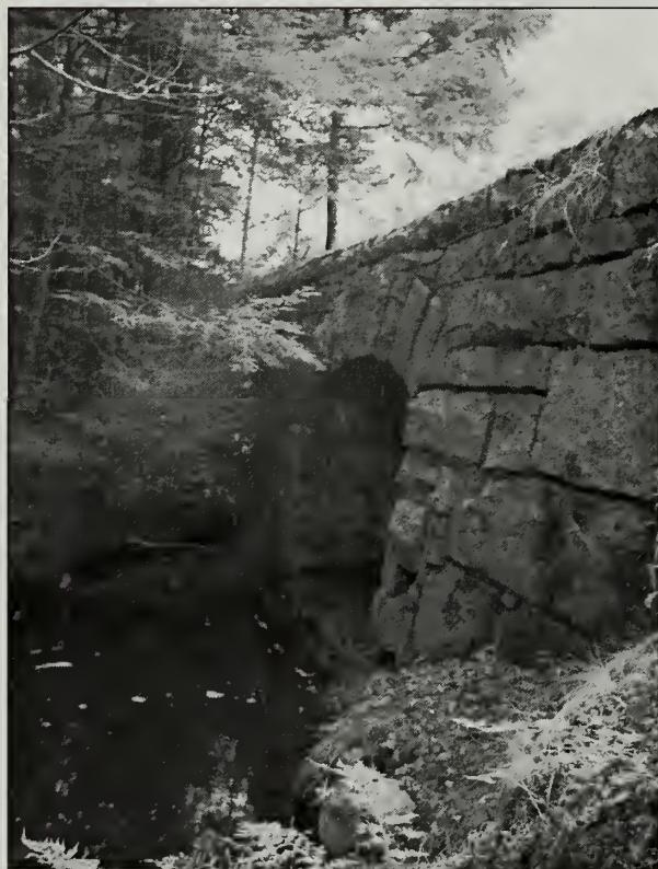
Figure 2.69. Impressive mortared stone outlet headwall of a concrete box culvert on Day Mountain Road. (Acad0300_13.227_Out(2), OCLP 2005)
