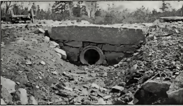
Figure 3.21. View of a dry-laid stone headwall on Cadillac Mountain Road, c.1930. (Courtesy Leo Grossman Personal Collection, #60-1)
