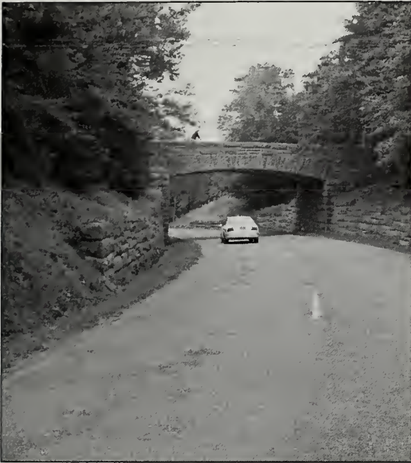
Figure 2.70. Mortared stone retaining walls segue to the carriage road bridge over Day Mountain Road. (Acad0300_12.448, OCLP 2005)
