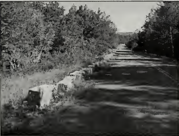
Figure 2.126. View east at rectilinear quarried block guardwalls on the West Street Extension off of Paradise Hill Road. (Acad0100_0.113, OCLP 2005)
