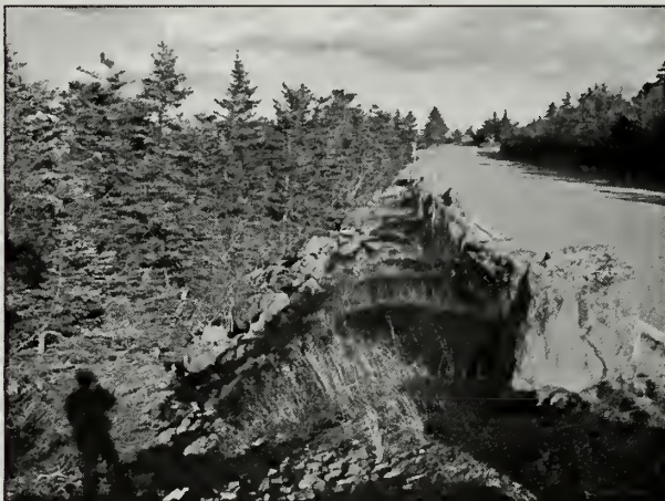
Figure 2.95. View of a guardwall and riprap embankment near the summit. (Acad0013_3.272, OCLP 2005)
