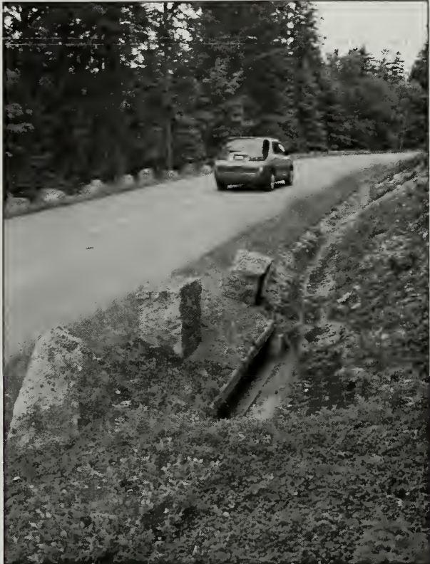
Figure 2.77. Many culvert inlets are marked by large coping stones because of the road's narrow shoulders. Most inlets and waterways are on the east side of the road while most guardwalls are on the west side. (Acad0012_1.077, OCLP 2005)
