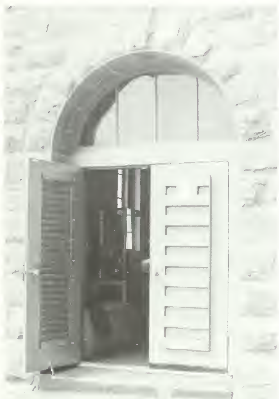
Figure 11. These louvered doors have been installed at Point Sur Light Station for security and ventilation. Note the baffles on the exterior and the screened louvers on the interior.
