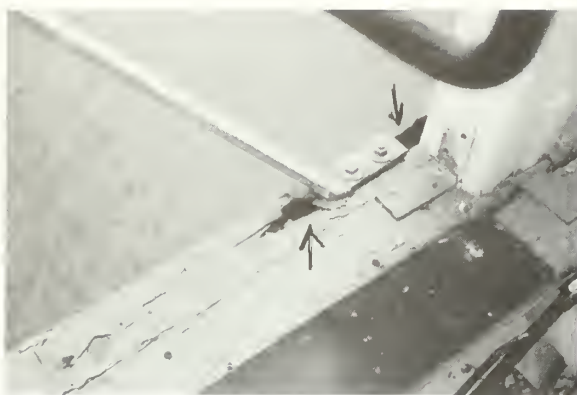
Figure 18. The wooden structural member that this bracket is attached to is extensively deteriorated. This condition is a prime example of deterioration that can be repaired by cutting back the rotted wood to a sound substrate, then fitting the void created with a wooden 'dutchman' or infill that matches as closely as possible the grain orientation and wood species as the existing member. Once the dutchman has been glued, and if needed, doweled in place, then the affected area should be properly primed and painted. This technique is affordable and incurs only minimal damage to the existing historic materials.
