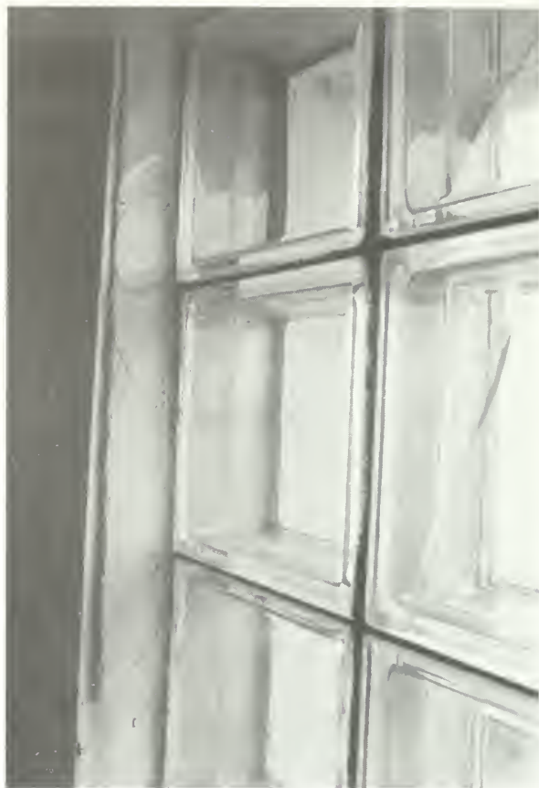
Figure 8. Close-up view of a glass-block window in a concrete lighthouse. The joint where the glass block meets the concrete wall should be caulked to prevent moisture infiltration.
