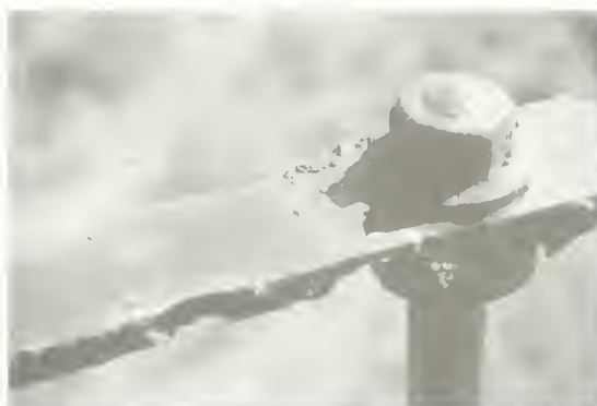
Figure 15. As corrosion attacked this steel handrail, wind and airborne sand eroded the loose and flaking surface rust.
