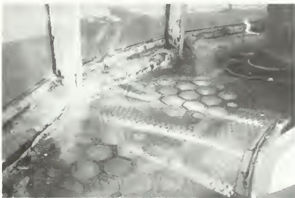
Figure 47. Lantern room before rehabilitation. Note the lower sill channels filled with concrete. This shortsighted 'repair' method blocked the ventilators and caused condensation to spill out on the deck, effecting rust and further damages below.
