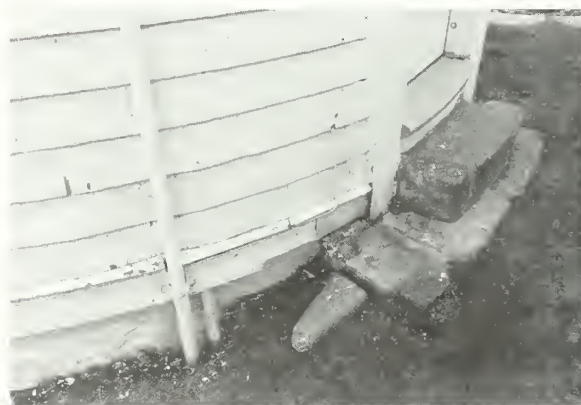
Figure 10. This door sill has a positive slope to ensure proper drainage; the joint where the door surround meets the shingles should be checked for gaps and recaulked if necessary.
