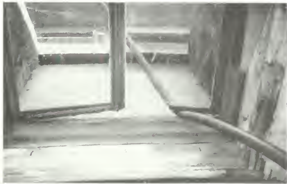
Figure 12. Close-up of severely deteriorated bottom rail of the same window in Figure 11. This condition can be repaired by splicing a new piece of sash
