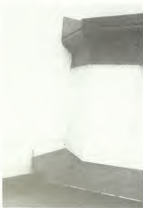
Figure 41 (left). This masonry lighthouse has been detailed with a two-tier cast-iron water table (the iron portions are painted black). Rust-bleed is occurring along lower edge of the upper tier.
