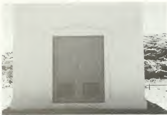
Figure 11. These replacement lighthouse doors have screened louvers that cover approximately 25% of the door opening to maximize air exchange.
