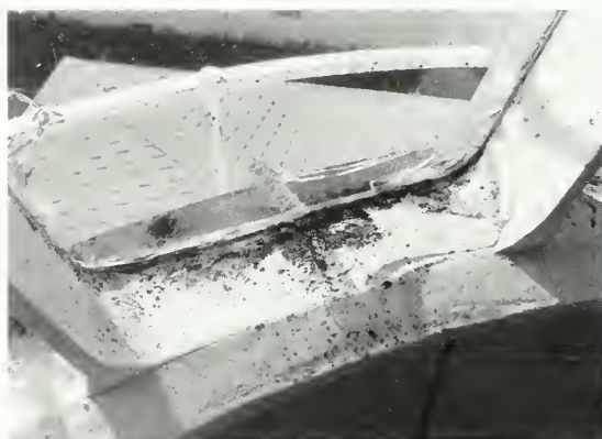
Figure 12. The glass in this lantern has been cracked by the rust-jacking that is occurring along the iron frame.
