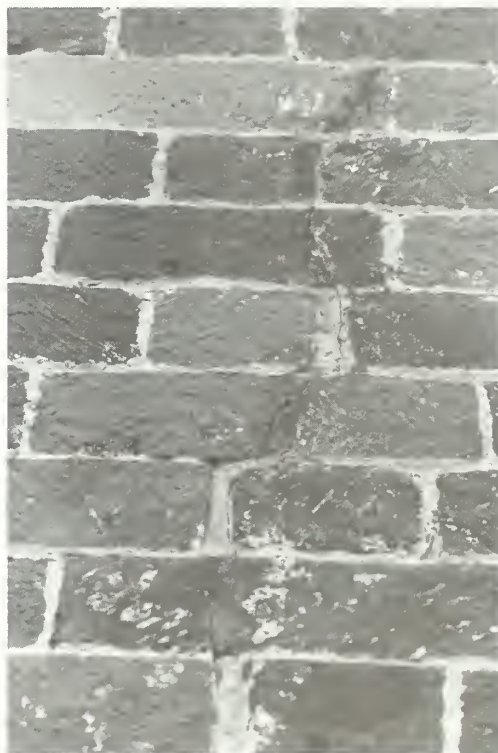
Figure 15. Cracks such these in a sandstone lighthouse should be monitored for movement prior to treatment.
