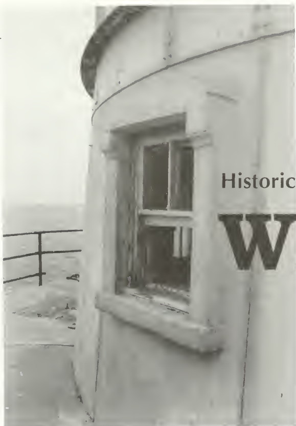
Figure 1. Close-up of a window found in a Chesapeake Bay "spark plug" lighthouse. The integral cast-iron trim is a typical character-defining feature of this lighthouse type from the late 19th century
