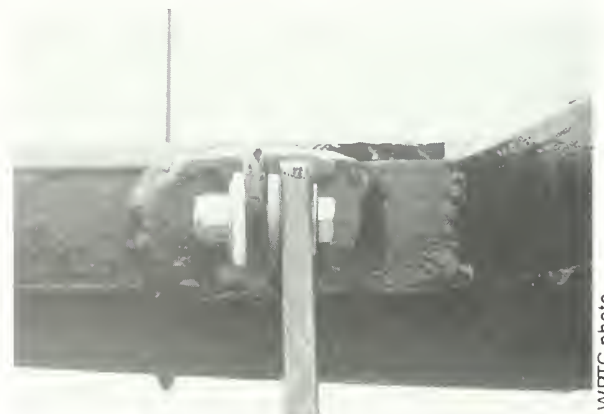
Figure 25. This is a view of a typical dissimilar metal isolation solution; the steel ladder post (vertical member in the center of the image) is isolated from the aluminum lantern gallery deck with nylon washers. The bolt chosen for this application is made from Type 316 stainless steel.
