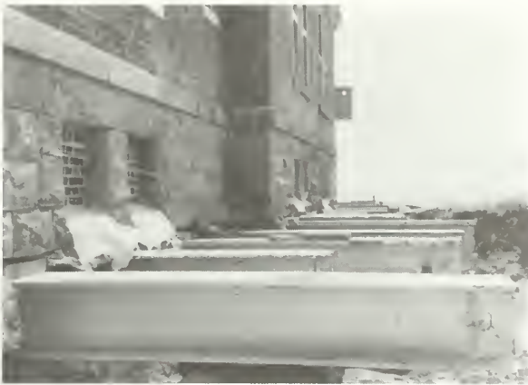
Figure 18. Large cross steel beams are inserted into the cut opening to form part of the grid that will carry the building.
