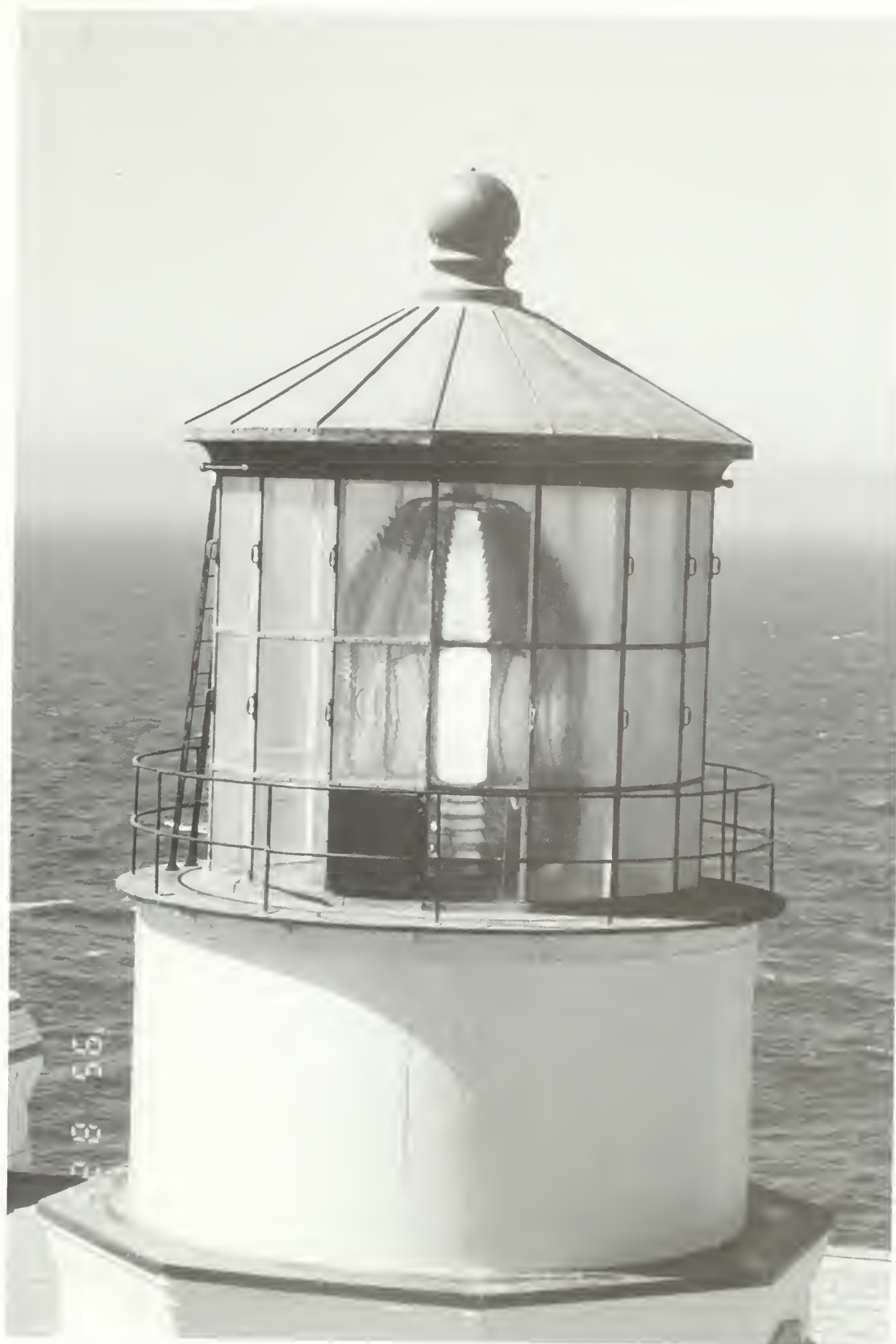
Figure 52. Light tower lantern after rehabilitation. The nonferrous metalwork at the lantern room is left unpainted and allowed to naturally patina, thus saving maintenance costs.
