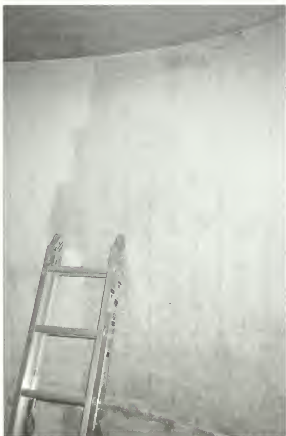
Figure 24. The interior paint was effectively removed using needle gun scalers, without damaging the concrete as evidenced by the visible impressions of the formwork boards.
