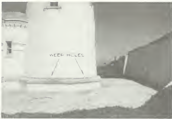
Figure 12. Typical masonry lighthouse weep hole locations. Each weep hole provides drainage for each individual cavity within the masonry wall.
