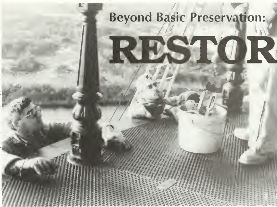
Figure 1. New ornate cast-iron handrail posts were recast and installed on the new gallery deck as part of a restoration at Cape Hatteras Lighthouse, Buxton, North Carolina.
