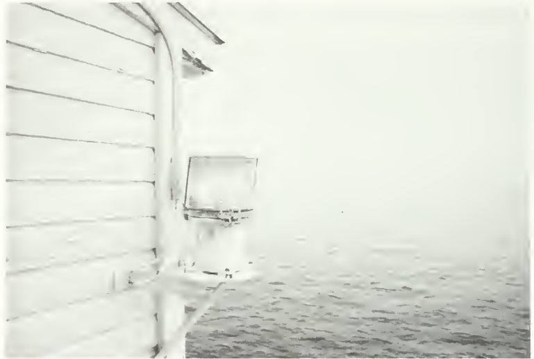
Figure 14. View of Class II paint condition: this example happens to be on the same lighthouse as the Class I condition shown in the previous image; multiple paint conditions can exist on the same lighthouse. In this example, only spot paint removal and repainting will be required to remedy the condition.
