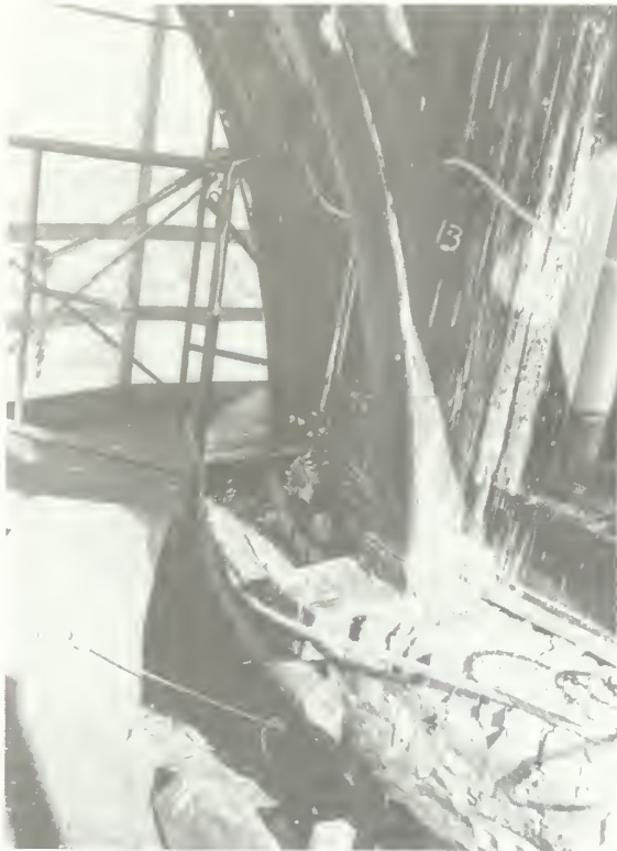
Figure 16. At the base of the brackets, the cast-iron belt course is removed, exposing deteriorated masonry below.
