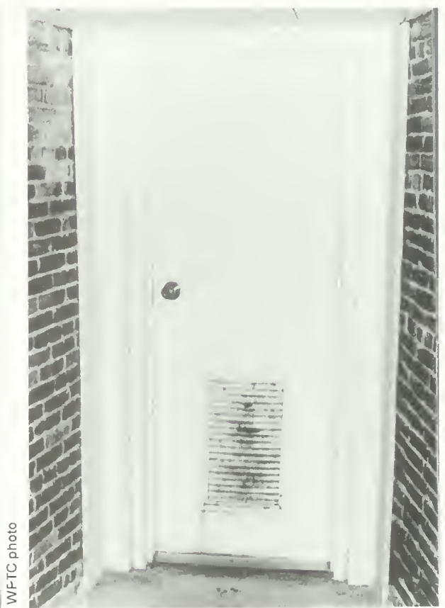
Figure 10. Interior view of the modern metal door at the Ocracoke Lighthouse before its replacement; corrosion like this should be removed and the affected areas treated with a rust-inhibiting coating system.
