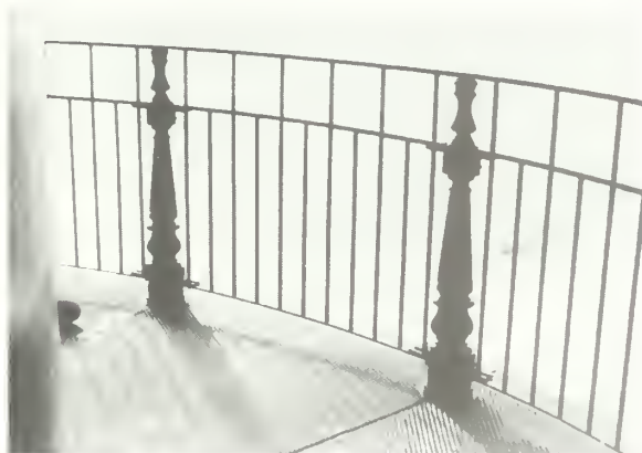
Figure 15. A replica handrail is installed.
