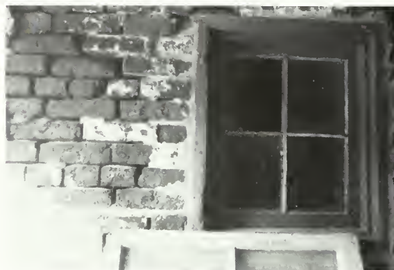
Figure 11. Detail of severely eroded brick and painting.
