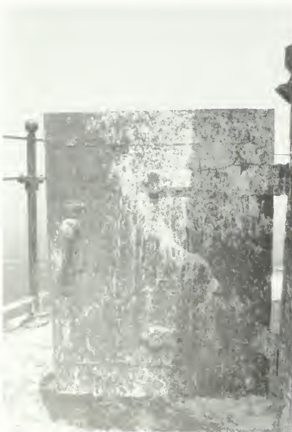
Figure 28. Surfaces such as this sheet-steel-covered parapet door that are covered with seagull guano should be thoroughly cleaned before mothballing and should be checked and cleaned once a year during the mothballing period.
