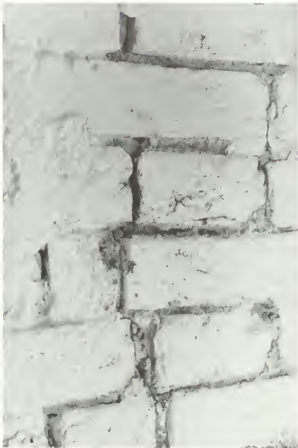
Figure 21. Detail of eroded pointing.
