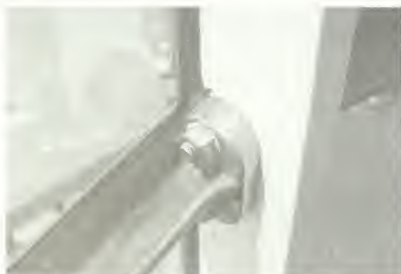
Figure 24. The stainless steel through bolts used to join this bronze sash bar to the vertical lantern post is isolated from the bronze using a nylon washer as a barrier.
