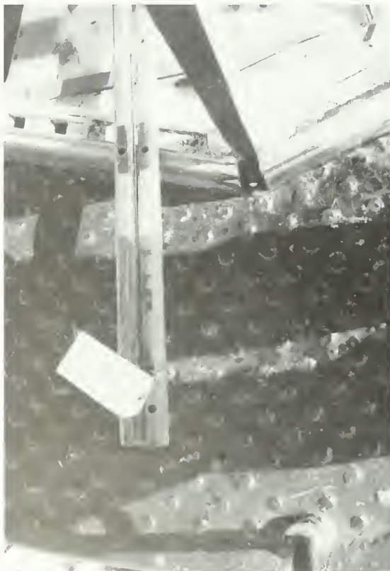
Figure 13. This detail of the bronze sill shows the location of the new lower fastener before its removal and resetting with the lower bronze mullion.
