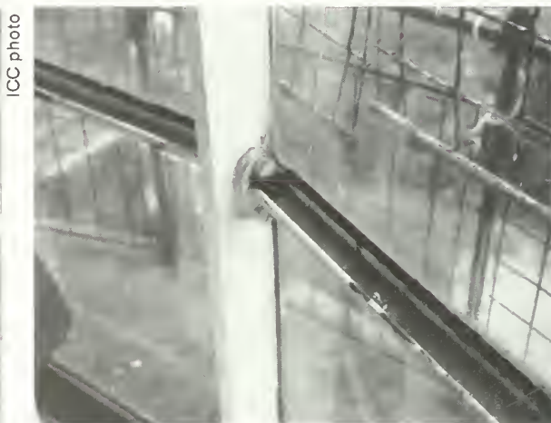
Figure 2 (left). Condition of the bronze sill sitting on the lantern deck inside the lantern room. The sill is wedged between two vertical cast-iron stiles, which are anchored into the masonry below.
