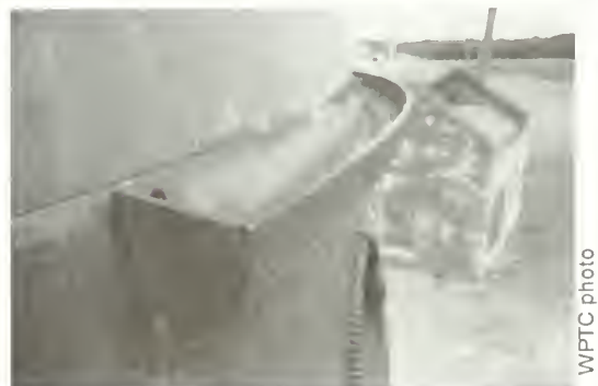
Figures 23 and 24. Two types of gutters found on iron lighthouses; the gutters must be in proper working order and checked regularly during the mothballing period.
