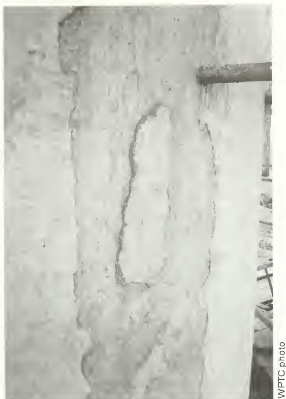
Figure 9. Patches of spalled concrete: familiar with lighthouse preservation the one pictured here should be repaired to protect the underlying concrete structure.
