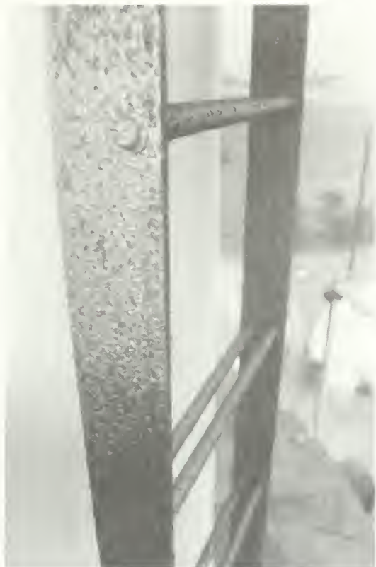
Figure 11. Detail view of a steel ladder that has been uniformly attacked by corrosion.
