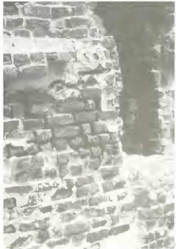
Figure 5. The coating that once protected the soft bricks of this lighthouse was not maintained; the severe deterioration required the replacement of nearly 25,000 bricks.
