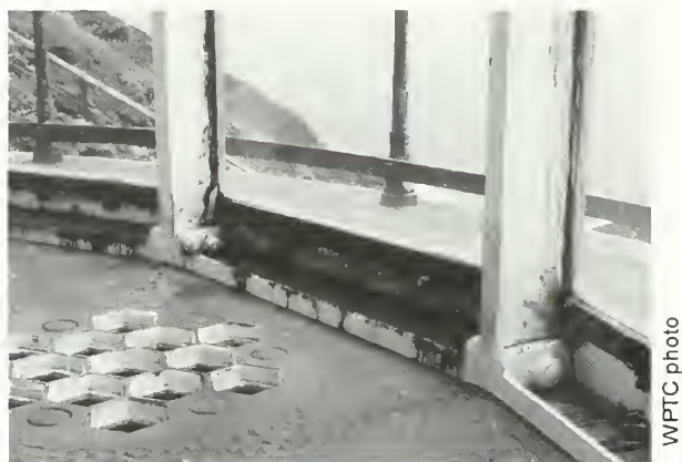
Figure 22. Close-up of sill vents in a first-order lantern. The vents should be kept open during the mothballing period to maximize lantern and tower ventilation.
