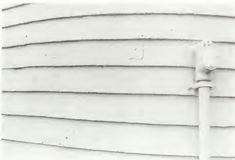
Figure 15. View of Class III paint condition: in this case the cracking, peeling, and alligatoring have been caused by excessive paint layer build up.
