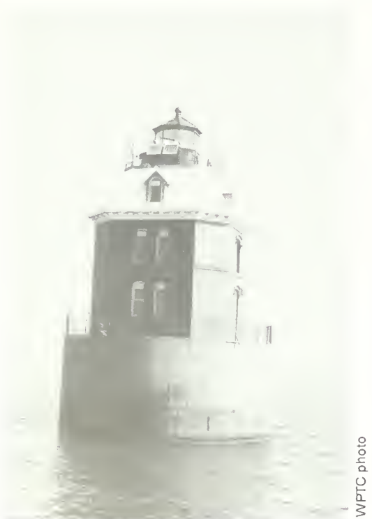
Figure 3. For the construction of this caisson-style lighthouse, unreinforced concrete was used as ballast to sink the cast-iron caisson foundation deep into the mud on the bottom of the Chesapeake Bay in Maryland.
