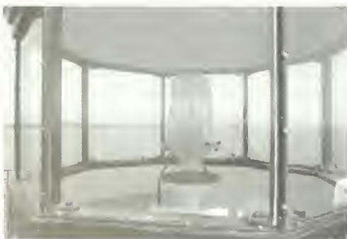
Figure 10. Close-up of a lantern glass frame: note the use of stainless steel bolts; the lower clamps are also stainless steel that have been painted black.
