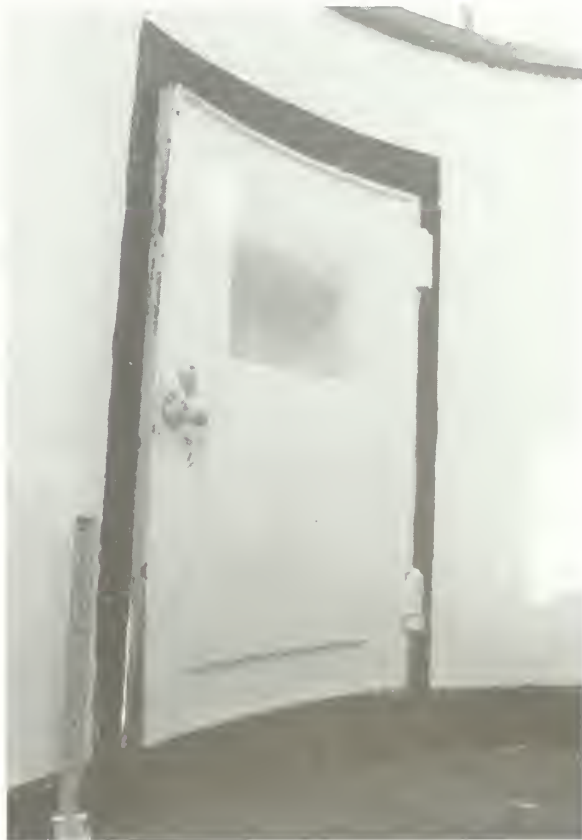
Figure 20. Close-up of a vented parapet hatch in a fourth-order lantern. The hatch should have a good seal and still remain operable. The built-in vent should also be kept open to maximize ventilation of the lantern and tower.
