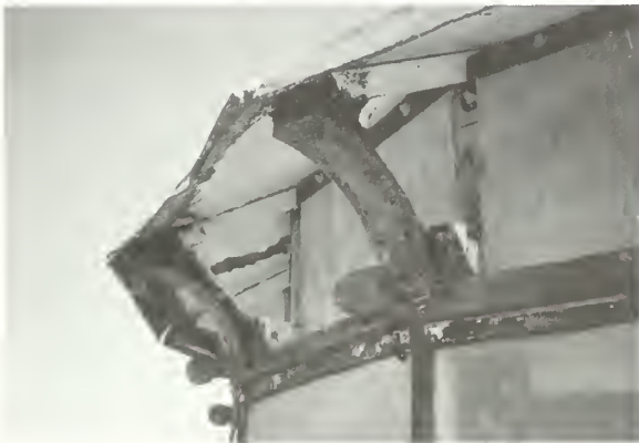
Figure 48. Reconstructing the cornice. The cornice plates were removed to expose the corroded cast-iron brackets and top channels. New brackets were cast in bronze, and the top sill channels were fabricated in stainless steel. Note the plywood 'curtain' erected for weather protection and shoring the lantern roof during reconstruction.
