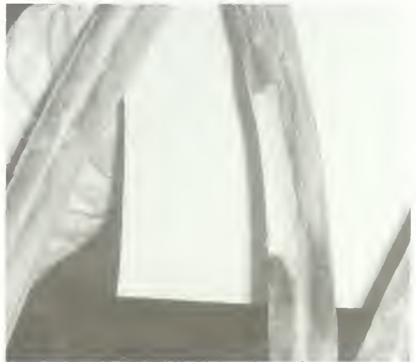
Figure 13. Close-up of a dutchman repair (light-colored wood used to mend a window muntin).
