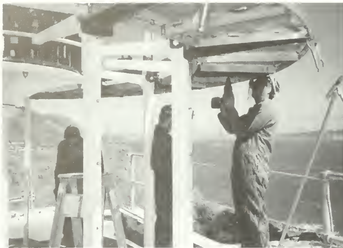
Figure 41. Final fitting and installation of the new aluminum deck plate.
