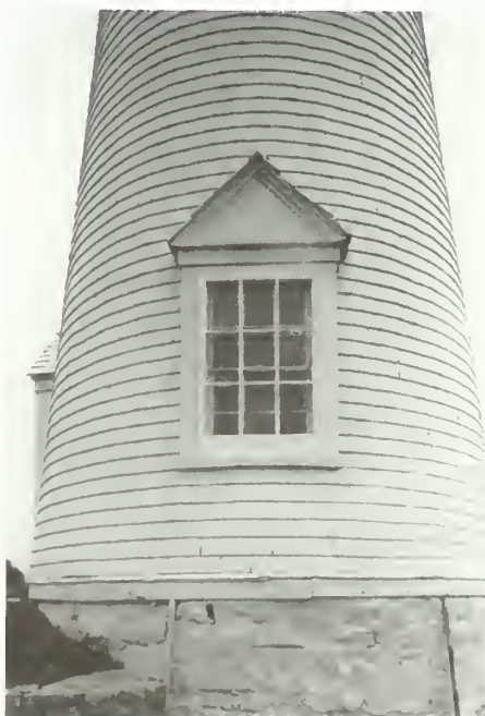
Figure 2. Stone masonry foundation in a 38-foot-tall wood-frame lighthouse in Maine.
