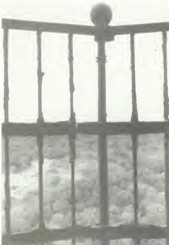
Figure 13. View of a steel railing where corrosion has occurred in distinct locations either because of variations in composition or localized failure of the coating system.
