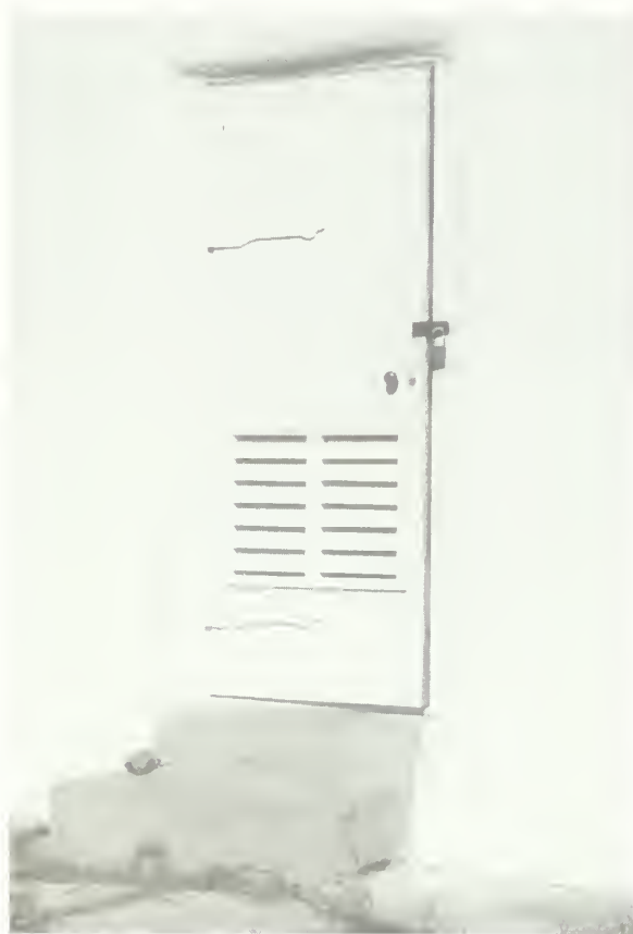
Figure 9. View of the Ocracoke Lighthouse five years after replacement; note rust streaks from nails. This condition indicates the paint coating has degraded to the point where moisture has permeated the surface.
