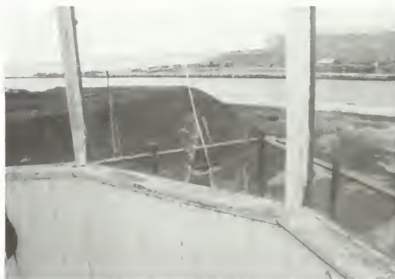
Figure 5. Storm glass with holes should be replaced as soon as possible to minimize water infiltration. If immediate replacement is not an option, the storm glass can be temporarily patched.
