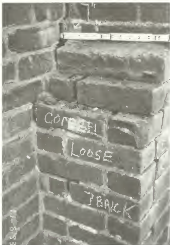
Figure 13. A complete structural survey of the building was performed and documented in order to perform the structural repairs necessary to move the building intact. All loose or eroded mortar joints were cut out and carefully pointed with a new mortar mix designed to closely resemble the original. All chimneys were braced and cabling installed around the perimeter to catch problem areas.
