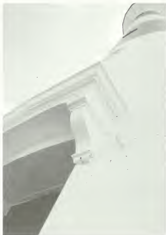
Figure 45. Within three months after painting, the rust began to bleed through this weep hole on the bottom of this pediment bracket. Two lessons are to be learned from this condition: 1) keep weep holes open to allow any water that may have entered the casting to escape, and 2) keep joints around applied castings sealed; apparently this was not done and water has entered the hollow cavity of the pediment, causing rust to form inside.
