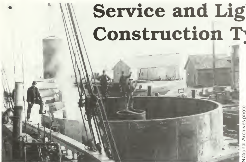
Figure 1. Assembly of Point No Point Lighthouse caisson at Solomons, Maryland, before being transported to site in Chesapeake Bay.
