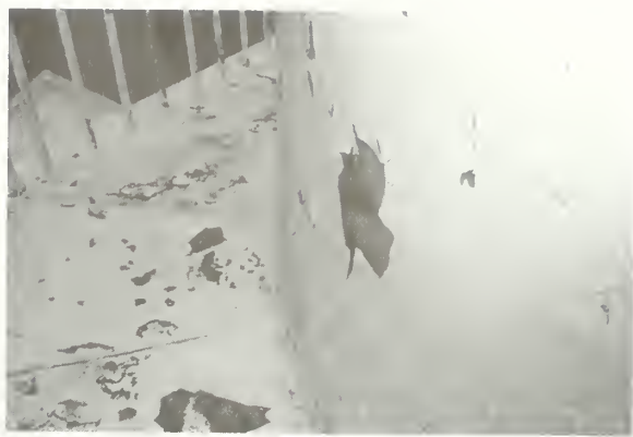
Figure 14. Detail of failing paint, a problem which should be addressed during stabilization and protection. In this particular case, spot painting may be all that is required to maintain a weatherproof protective coating.
