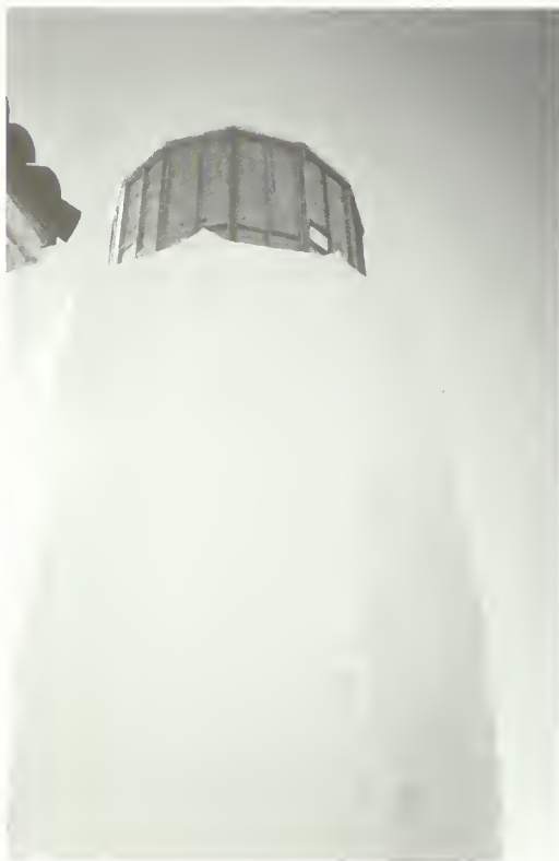
Figure 22. View of the lighthouse scaffolding covered with shrink wrap to contain all hazardous materials and protect workers from severe weather.
