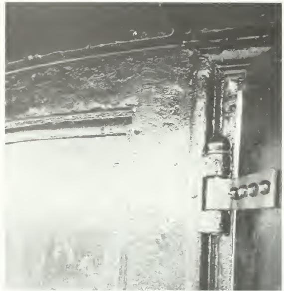
Figures 36 and 37. The left image shows the condition of the iron exterior service room wall before rehabilitation. The right image shows the same area after power hand tool cleaning and coating. The crescent shaped scars in the iron are from the arc of a grinding wheel.
