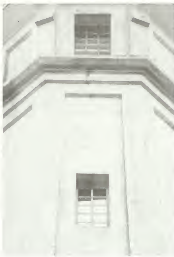
Figure 10. Cracks like the one here, extending down from the belt course of this concrete lighthouse, should be monitored for movement before any patching is performed.
