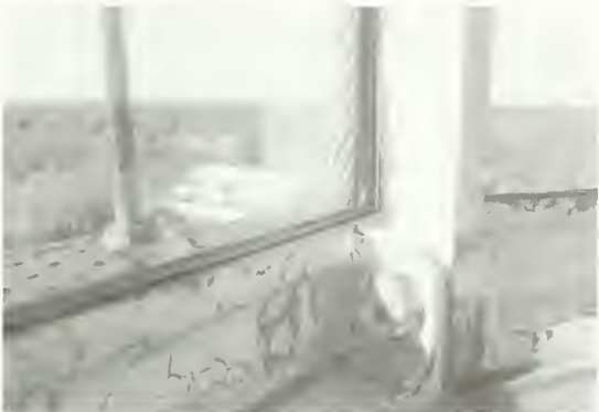
Figure 16. This detail shows the new glazing system in place with associated cast-iron post and bronze sill available to receive additional cleaning and paint removal.
