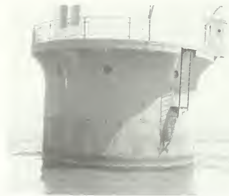
Figure 17. The cyclic pressure of the different rates of expansion and contraction of the exterior cast-iron plates and the interior brick lining of the caisson-style lighthouse has caused the cast-iron plates to fatigue and crack.
