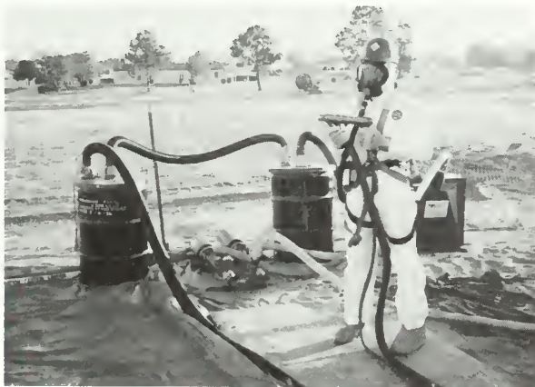
Figure 29. Worker dressed in full personal protective gear. The full-face-shield self-contained respirator provides both respiratory and eye protection. The worker is wearing protective coveralls, gloves, and boot covers to prevent lead dust contact. The harness is part of a full protection system. He is holding a pneumatic needle gun that is hooked to a two-stage HEPA (High Efficiency Particulate Air) filtered vacuum system.
