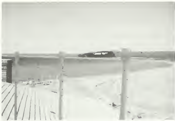
Figure 26. Detail of handrail that is being deformed by rust-jacking.
