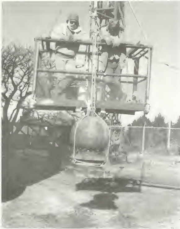
Figure 4. The first step in removing the roof was to take off the vent ball. The vent ball not only serves as a lightning rod but also provides ventilation to the glass in the lantern room, limiting condensation.
