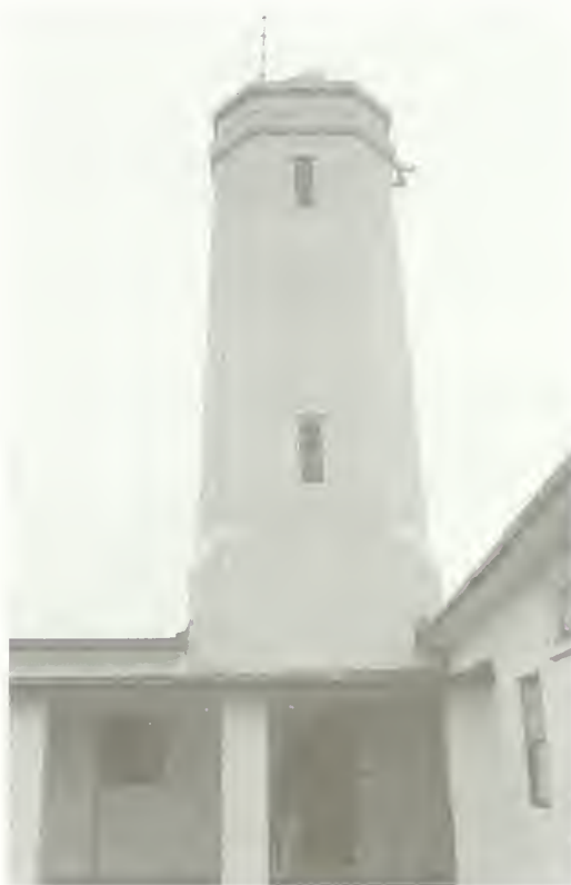
Figure 5. St. John's River Lighthouse, Mayport, Florida, was constructed of reinforced concrete for its economy and low maintenance.
