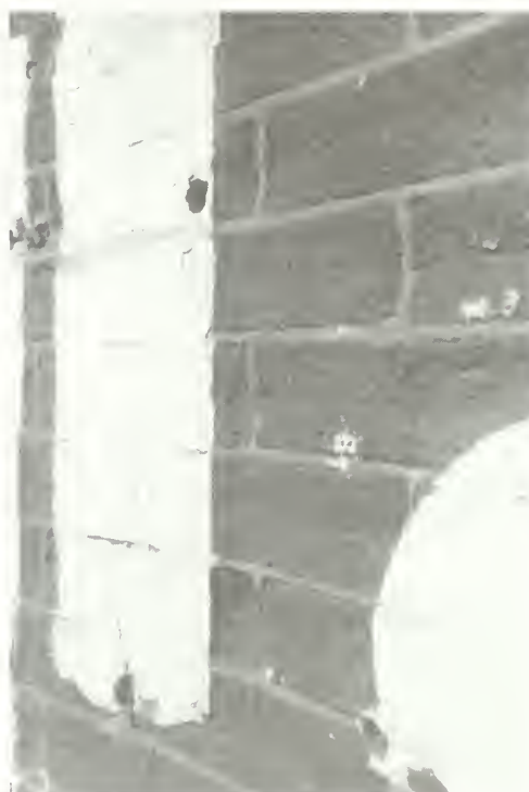
Figure 17. Deeply eroded brick as a result of sandblasting. The white areas are where electrical components were attached to the wall at the time of sandblasting.
