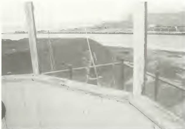
Figure 16. This lantern glass has been damaged by rock-throwing vandals. The resulting hole is allowing rain and insects to enter the lantern.
