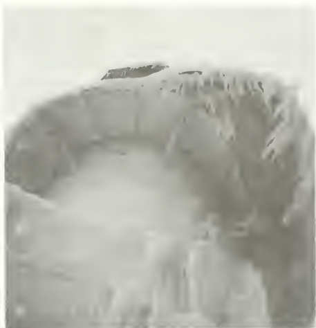
Figure 15. Close-up of ice on St. Joseph North Pier Lighthouse causing damage to gallery deck and handrail.
