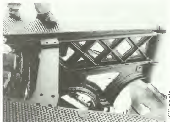
Figure 13. After the most severely deteriorated portion of the brackets were removed, new cast-iron pieces were made and installed; and new deck plates installed.
