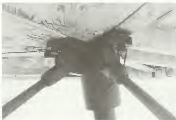
Figure 12. View of underside of a screwpile lighthouse. Although these bare wood surfaces are not directly exposed to rain, they are susceptible to mist and condensation moisture; and because there is no exposure to direct sunlight, the surfaces are seldom dry. For adequate protection during the mothballing period, these surfaces should be painted.
