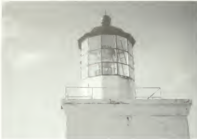
Figure 33. Point Bonita Lighthouse before rehabilitation; note missing gallery deck and holes below between the bottom of the lantern glass and top of the service room wall.
