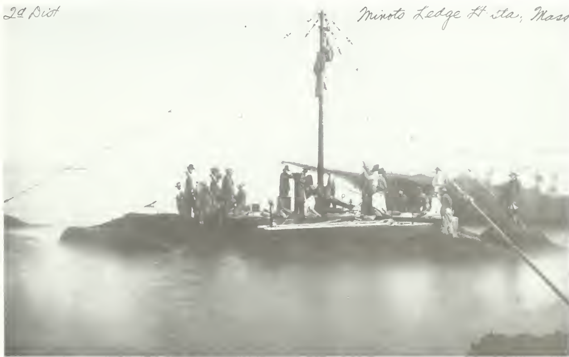
Figure 30. Workers on a calm day, completing the first course of granite block for the foundation of Minots Ledge Lighthouse, 1858
