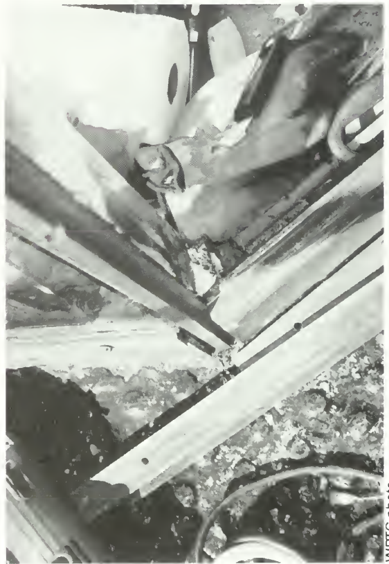
Figure 14. Following placement of the restored bronze mullion, the fenestration is ready to receive the new glazing system.
