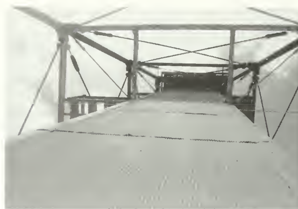
Figure 9. If the exterior of the wooden tower has been covered with another sheathing material like this corrugated metal, all joints in the exterior sheathing should be made completely weathertight; at this particular lighthouse, deterioration of interior wood framing members was caused by moisture infiltration.
