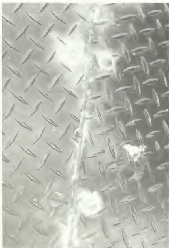
Figure 7. The white chalky residue around the steel bolt heads on this aluminum deck is the by-product of the corrosion occurring at these connections.
