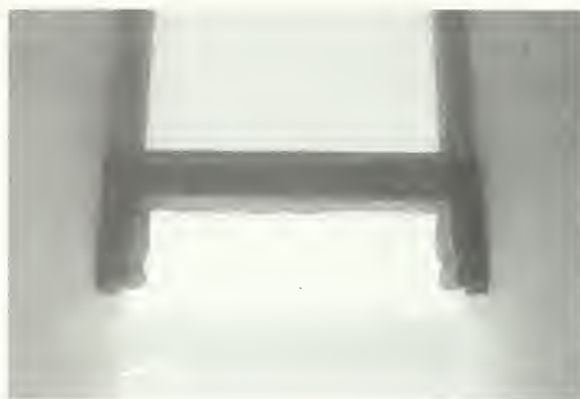
Figure 6. The once crisp edges of this decorative granite lintel have been eroded by constant high winds and airborne sand.
