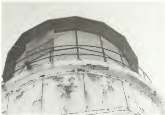
Figure 46. Lighthouse lantern before rehabilitation. Note the missing ladder rails and the severe rust on the lantern cornice and lower watch room panels. The badly spalled concrete gallery deck was installed in 1947 and is not original.
