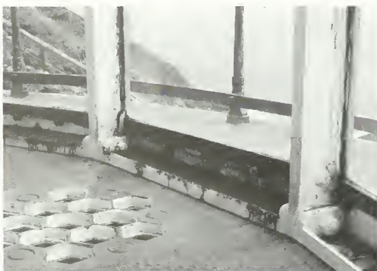
Figure 11. The water that has collected in this lantern sill is causing the iron lantern glass frame (the vertical members in the center of the photo) to rust and corrode.
