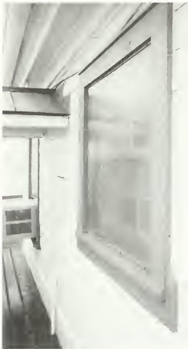
Figure 13. This image shows a Class I paint condition: virtually no deterioration, only some soiling and possible salt buildup resulting from the open-water location of the lighthouse.
