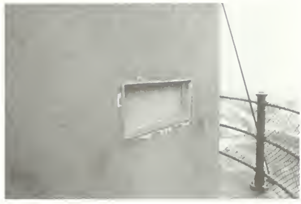
Figure 27. This lantern vent opening has been covered with a fine stainless steel screen that prevents insect infiltration while maximizing air movement through the vent and into the lantern.
