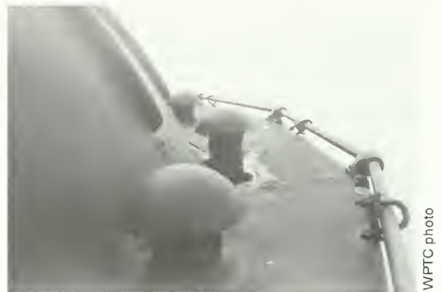
Figure 17. Roof vents such as these should be inspected for leaks and maintained during the mothballing period. This shroud-style vent allows air to pass while preventing rain from entering.
