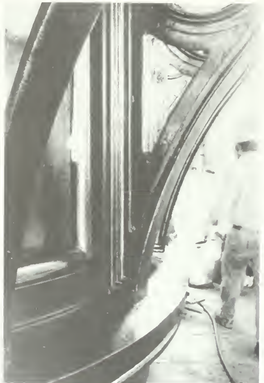
Figure 17. The cast-iron belt courses are repinned to new masonry beneath.
