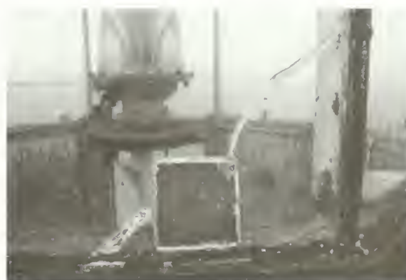
Figure 6. An acceptable temporary lantern glass repair made using a small piece of sheet metal and caulking.
