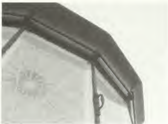
Figure 30. Close-up of a first-order lantern that retains its lantern glass; note the clarity.
