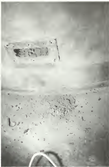
Figure 19 (left). Buildup of rust in parapet wall vents.
