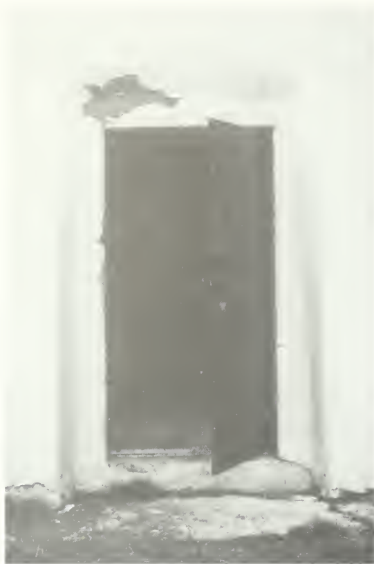
Figure 13. Site-built steel door at the Turkey Point Lighthouse; this solution was chosen because of the remote location and repeated break-ins. Note exterior stiffeners and shroud over the hasp and lock.
