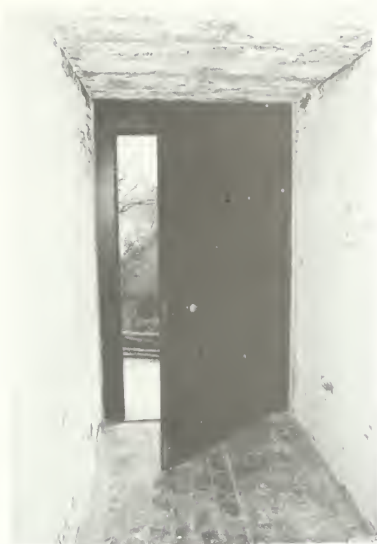
Figure 5. View of the large, single-leaf, wood-plank door at the Cape Henry Lighthouse (first tower), Fort Story, Virginia.
