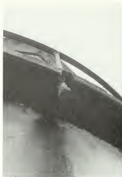
Figure 10. View of underside of gallery deck; the streaks on the stucco indicate that water is passing between the deck plates and possibly entering the masonry wall.
