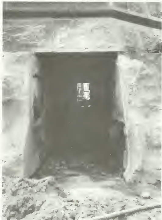
Figure 16. Close-up of the opening for the beam cut by the wire saw measuring 5 feet high by 3 feet, 6 inches wide. The depth of the cuts ranged from 18 inches to 16 feet for multiple wall cuts.
