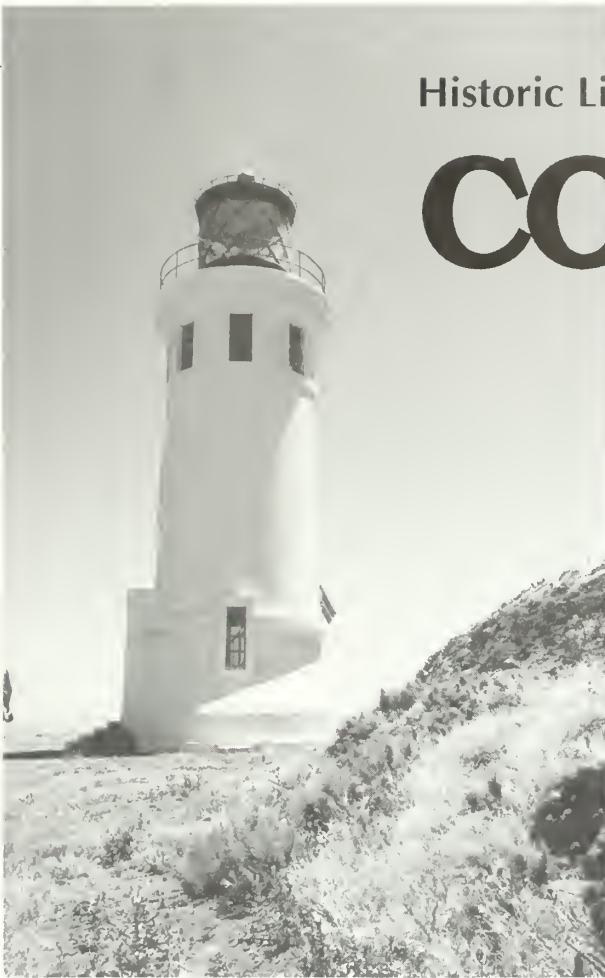
Figure 1. Anacapa Island Lighthouse is a reinforced concrete lighthouse located on a highly exposed island off the California coast. Concrete was chosen because of its ability to withstand the high winds, harsh climate, and seismic activity of this exposed location.
