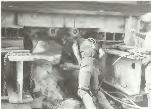
Figure 19. Once the initial lift was performed, the remaining foundation between the beams was removed.
