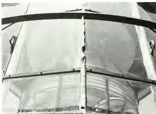
Figure 14. Wind and airborne sand have accelerated the deterioration of this lantern gallery deck handrail
