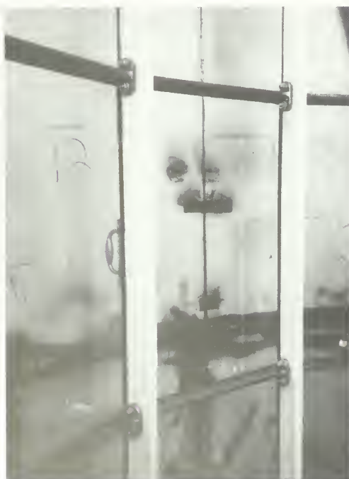
Figure 7. Inside the lantern room, the mullions have been reworked and reattached to the stiles. New stainless steel bolts have been used to prevent corrosion and teflon tape has been used as a gasket between the bronze and the cast iron. Teflon washers also separate the bronze from the stainless steel bolt.
