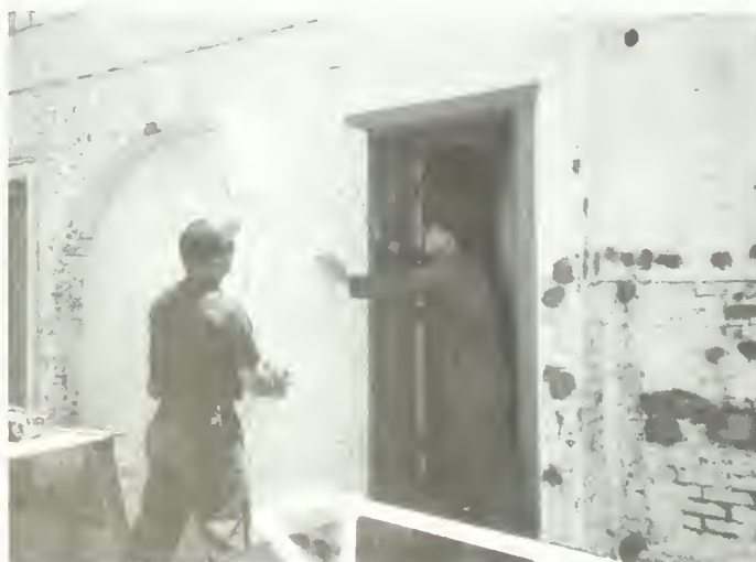
Figure 43. Installation of the new exterior wood storm door.
