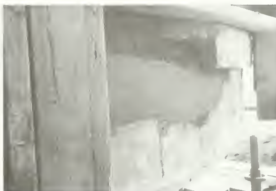
Figure 29. The first application of the mortar patch material to the damaged concrete.
