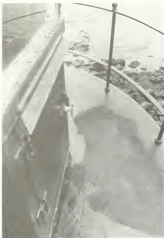
Figure 7. Ponding is occurring on this gallery deck near the base of the lantern parapet wall. This ponding has led to an active leak that occurs even during light rain conditions. A condition such as this should be remedied before the mothballing period.
