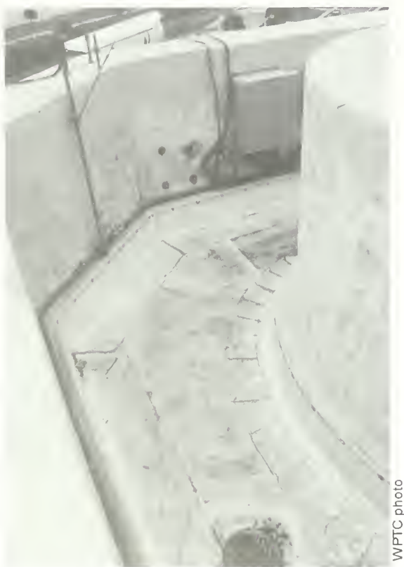
Figure 7. The concrete gallery deck on this concrete lighthouse has been covered with a rubber membrane. This covering should be checked regularly for leaks.
