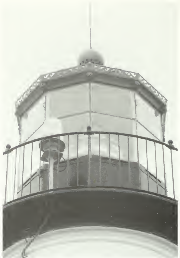
Figure 35. This is an acceptable auxiliary light installation. The light is mounted on an aluminum pedestal that has been bolted to the replacement aluminum deck.
