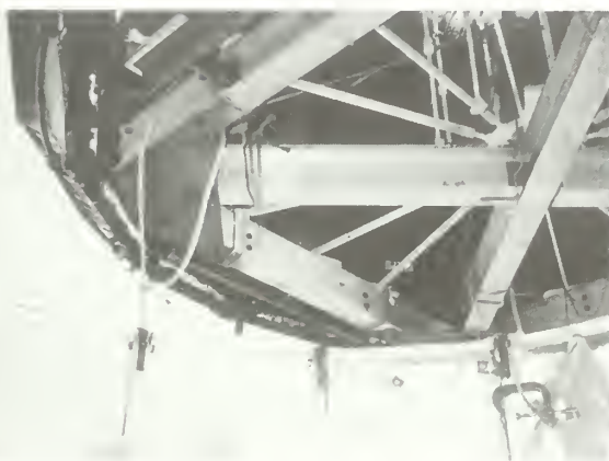
Figure 5. As the roof is being removed from the lighthouse, the tie rod system, supported by ICC's aluminum roofing frame, is visible. This frame was designed to fully support the roof and alleviate any stress or strain on the roof during the lift. Protruding down from the roof are the ends of the rafters which connect to the top of the stiles.
