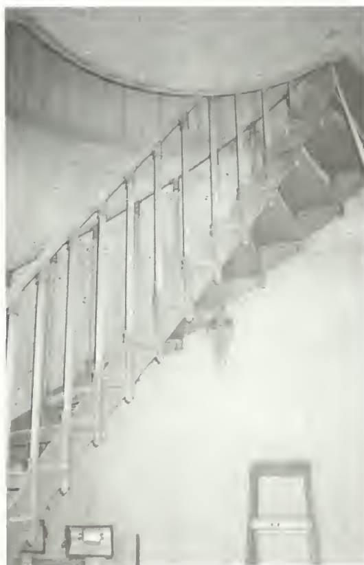
Figure 25. After the cast-iron stairs were blast-cleaned, they were rinsed to remove all traces of lead dust; flash rust immediately formed (as seen in this photo). Before painting, this light rust was removed with wire brushes.
