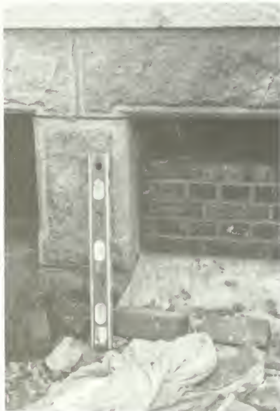
Figure 12. In preparation for the move, the cellar windows openings are temporarily bricked in to stabilize the masonry above the lift point.
