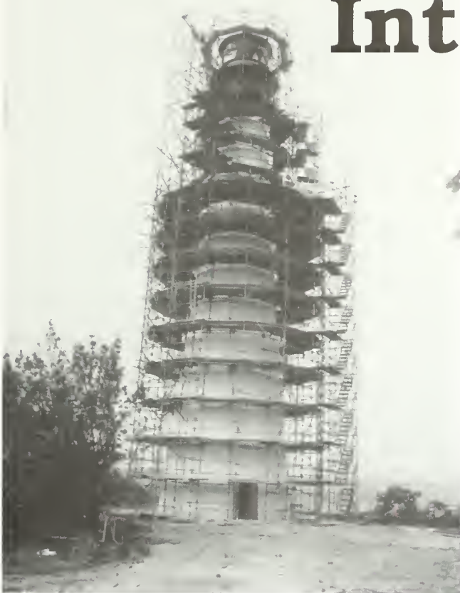
Figure 1. Brick replacement in 1996 restoration at Cape Florida Lighthouse on Key Biscayne, Florida.
