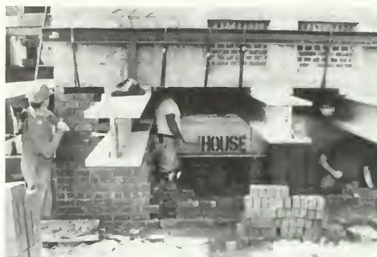
Figure 22. Construction of a new foundation around the support beams.
