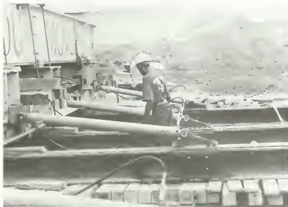
Figure 20. Four hydraulic rams set into the track steel pushed against the main steel to set the lighthouse in motion.
