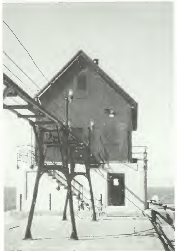
Figure 15. View of watertight 'ship' style door installation on the Grand Haven South Pierhead Front Range Light, Grand Haven, Michigan.
