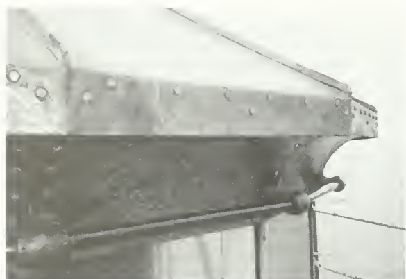
Figure 50. Lantern cornice after rehabilitation. Replacing the original steel cornice plates with copper eliminated the dissimilar metals problem.
