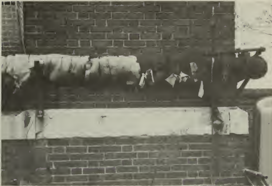
11. Spalling and loss of material at limestone water table due to rusting pipe anchors.
