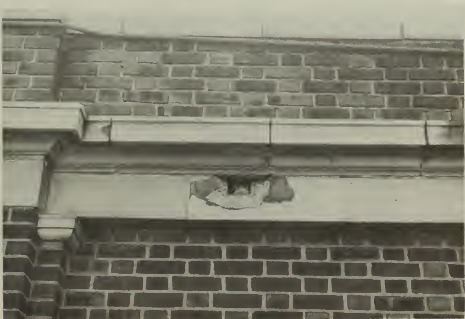
7. Hole and spalling, west elevation.
