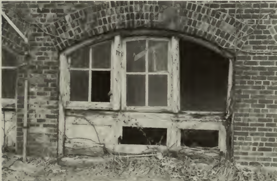
16. Rotting, broken, and missing window, west elevation.
