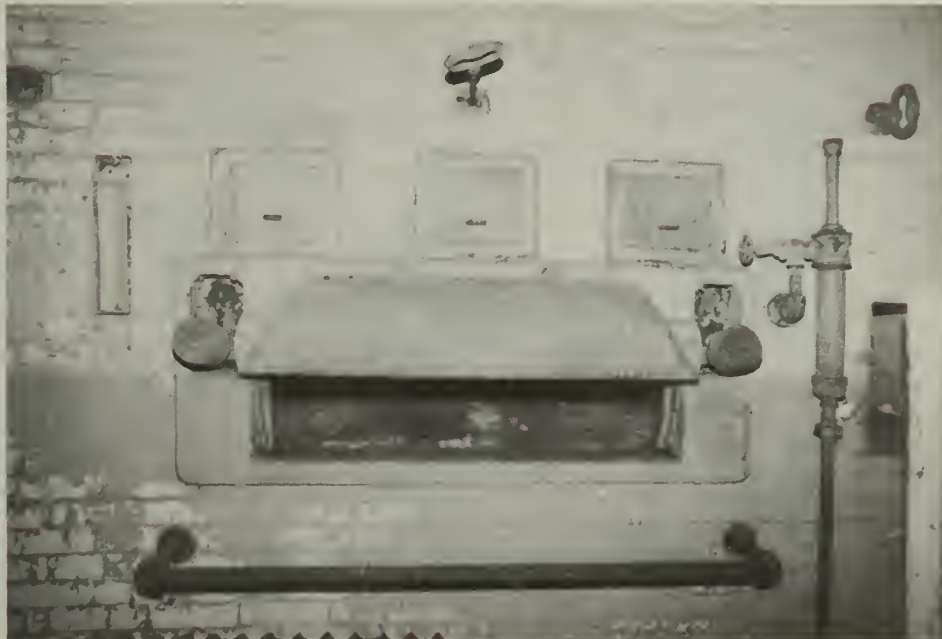
5. Room 101- south wall, one of three oven loading hoods- "Middleby Oven Co., N.Y."
