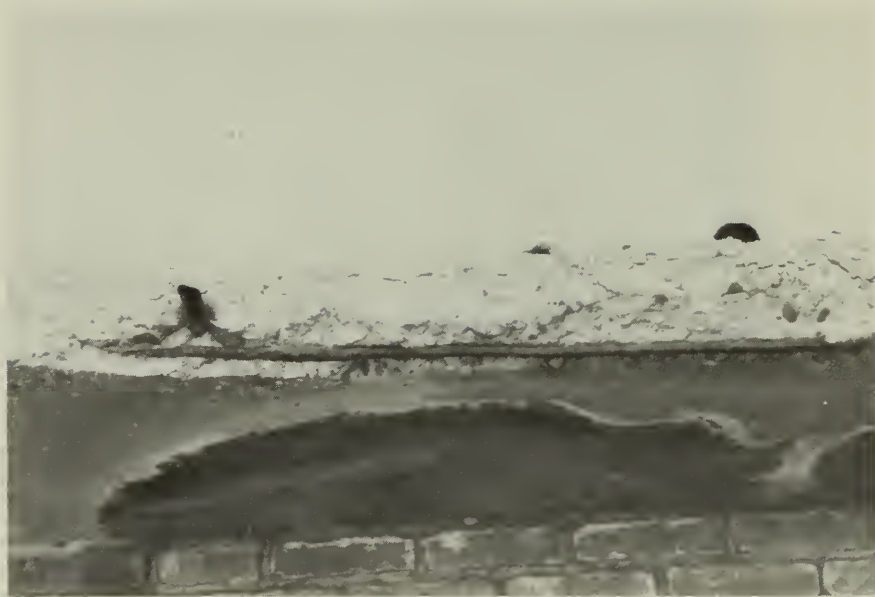
13. Exposed corroding beam causing concrete spalling, lintel on gabled projection.
