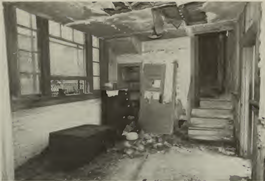
12. Room 104- lowered ceiling forming mezzanine level above. Deteriorated vinyl flooring revealing original hexagonal floor tile.
