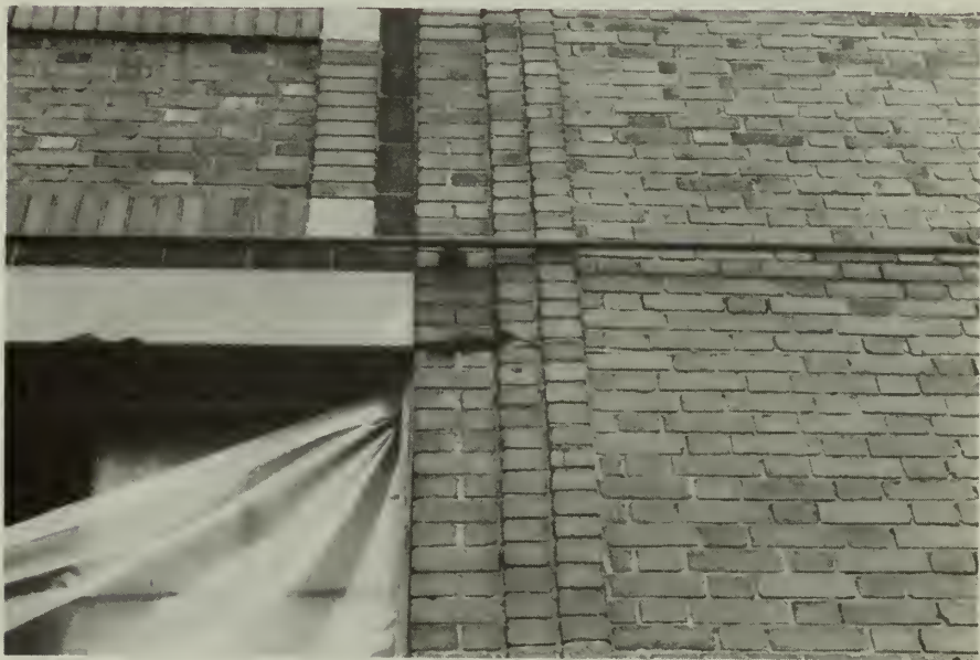
10. Spalling at lintel, west elevation.
