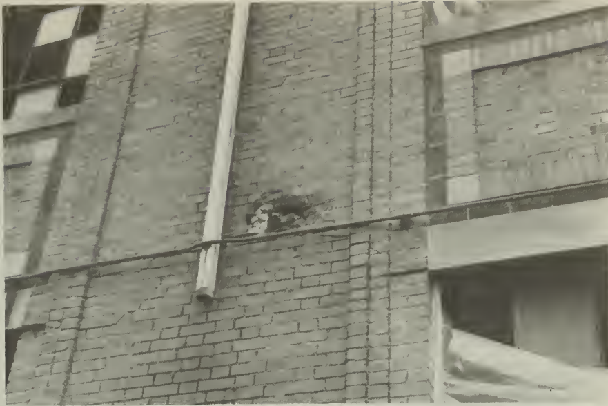
7. Missing downspout and missing brick, west elevation.
