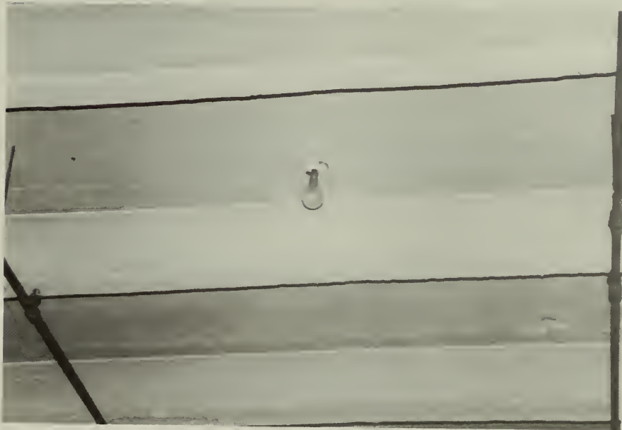
2. Porcelain socket ceiling mounted lamp, room 101.
