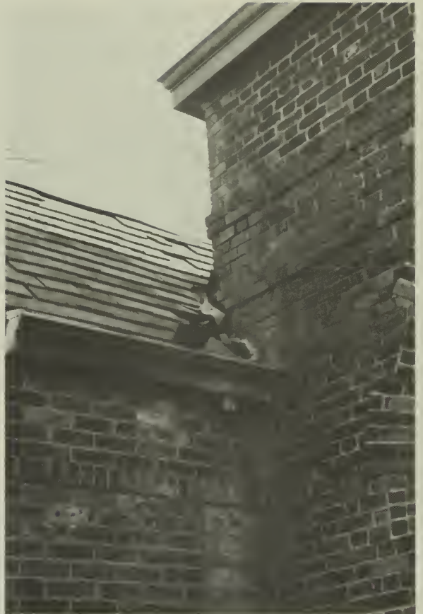
18. Torn flashing at juncture of gabled projection and pavilion, west elevation.
