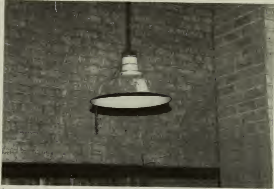
1. RLM-type fixture, c. 1935, room 103.
