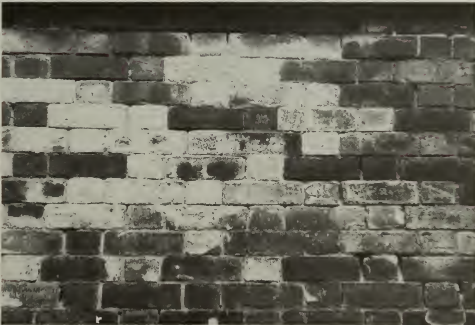
4. Efflorescence, south elevation.
