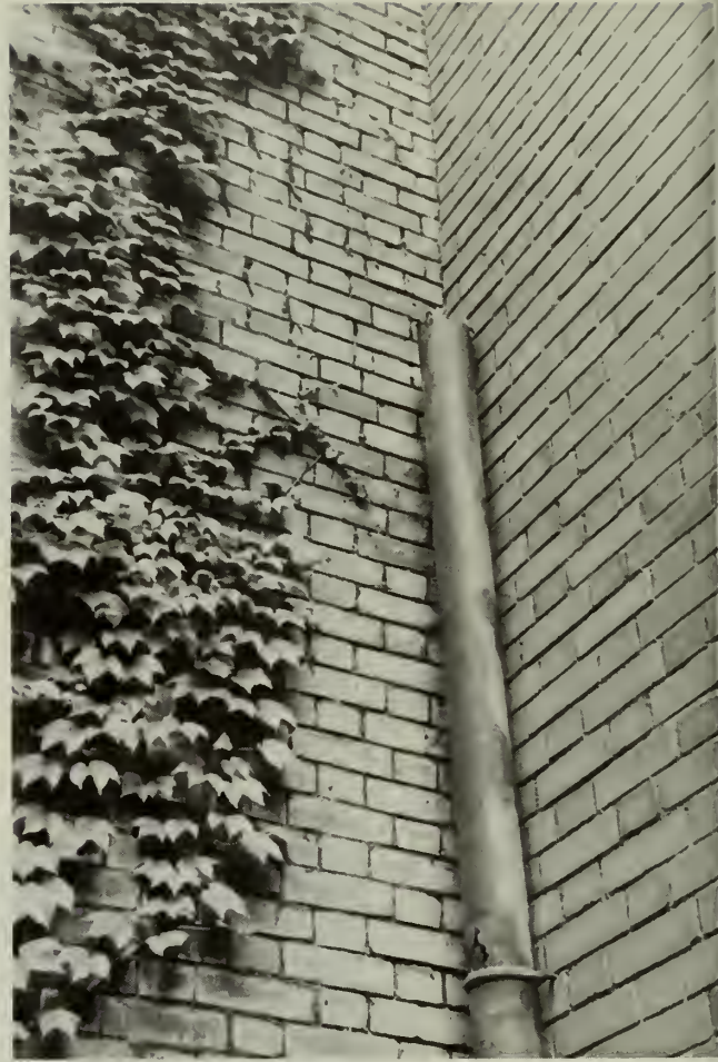
6. Biological staining, north elevation at juncture with corridor 2.
