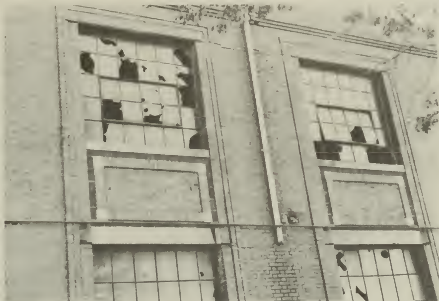
5. Brick pushed out at crack along second floor window tops, west elevation.
