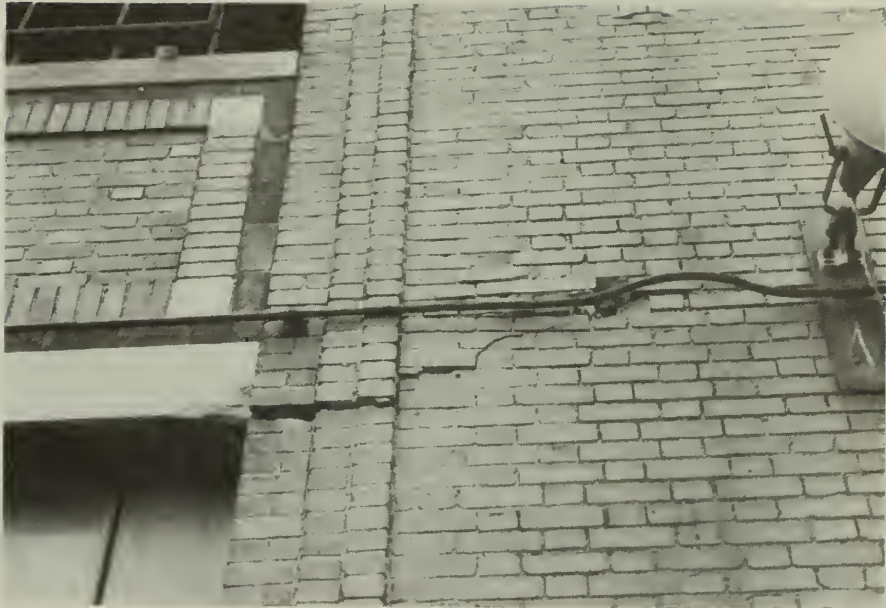
9. Severe cracking at lintel level, west elevation.
