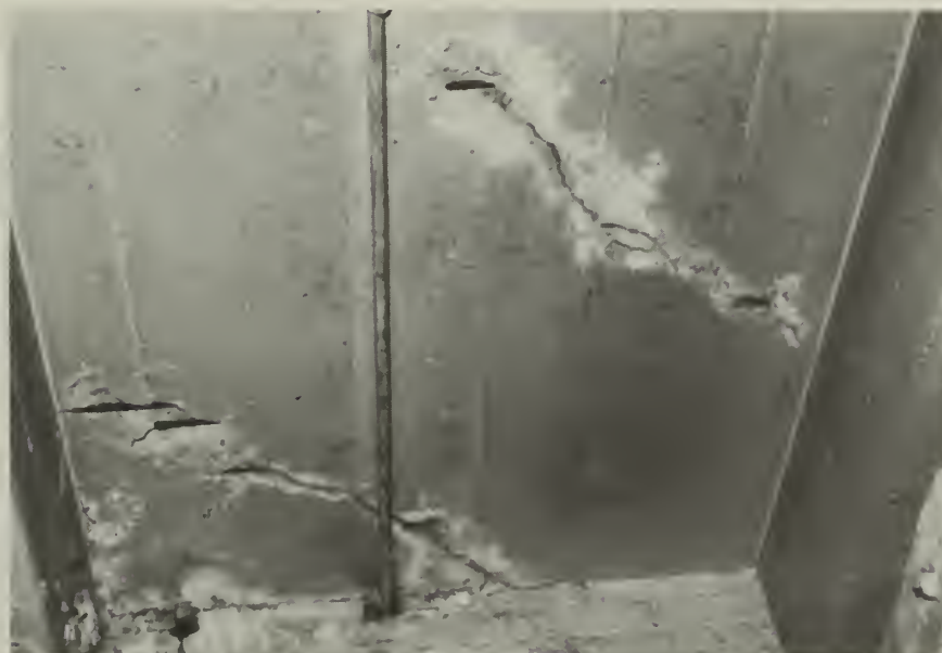
2. Crack at northwest corner of room 101.
