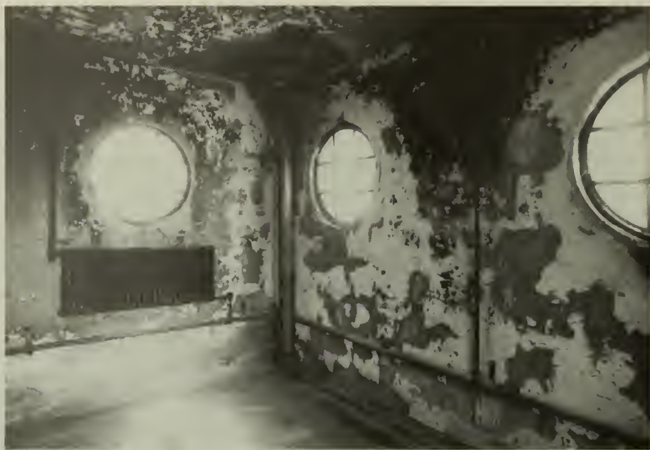
8. Room 103- view of northwest corner, exposed terra-cotta on walls and ceiling lath. 139
