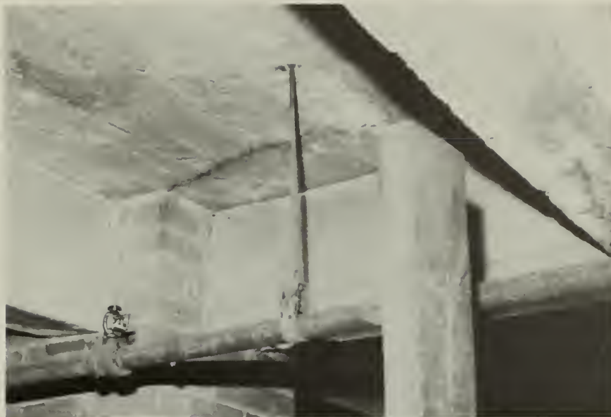
1. Crack in underside of second floor slab.
