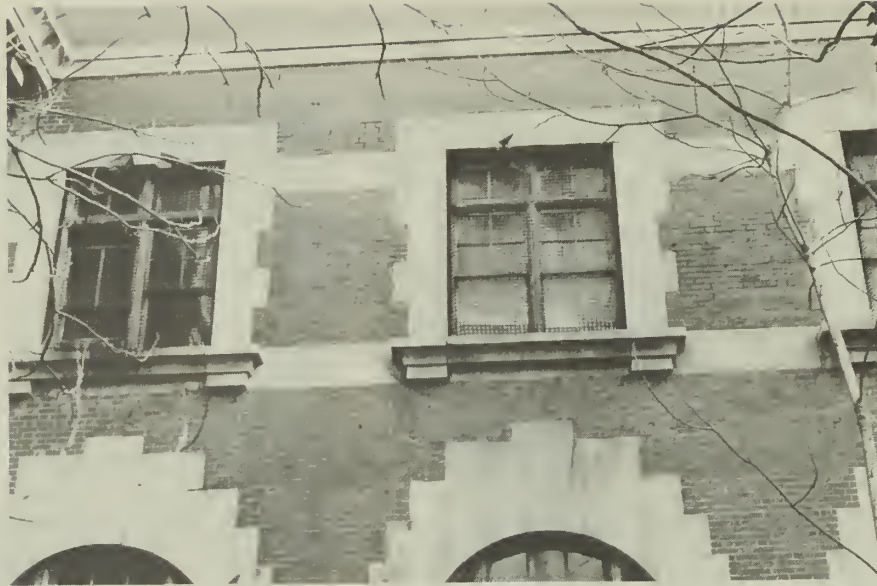
16. Cracking and spalling of stone on either side of keystones on the west facade of C-2.
