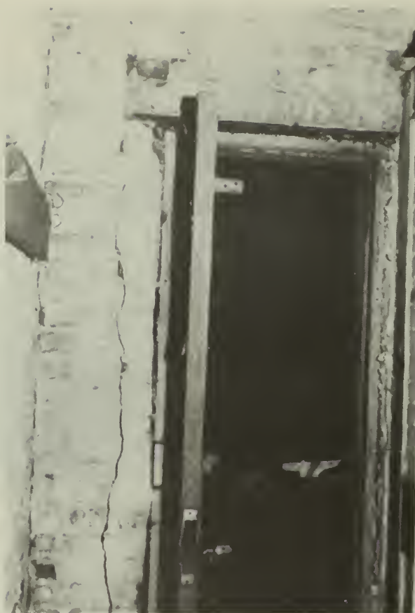
3. Crack along west side of door, north wall, room 101.
