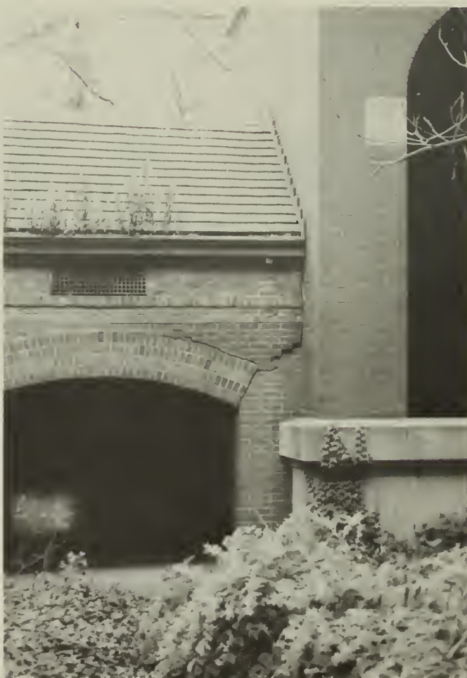
8. C-4- separation at mortar joints on east wall near arched pavilion to baggage and dormitory building.
