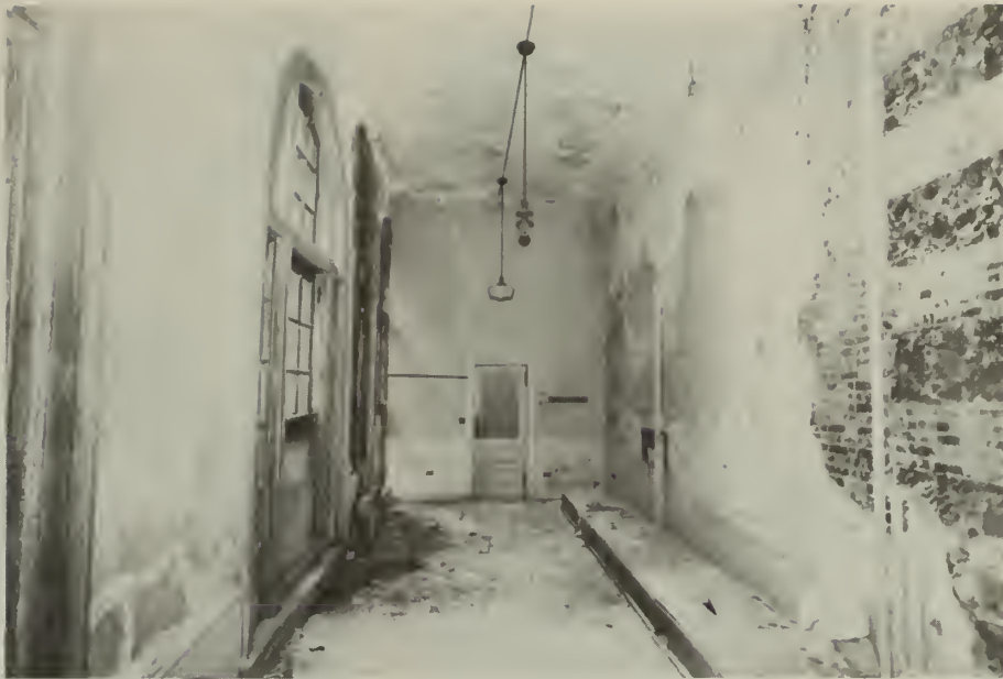
8. Room 105- looking south- raised platform floor over original ramped floor.
