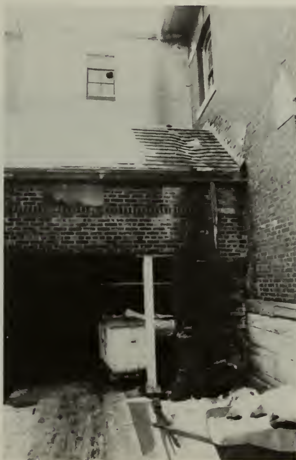
12. Crumbling brick and temporary wood support, east elevation of C-5 adjacent to powerhouse, view west.
