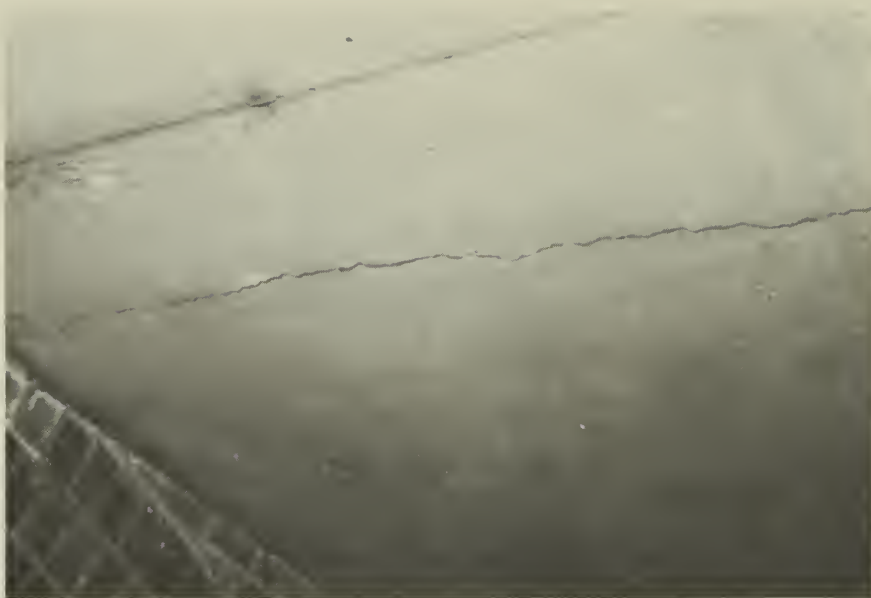
7. C-4- transverse cracks in the ceiling with evidence of water leakage.
