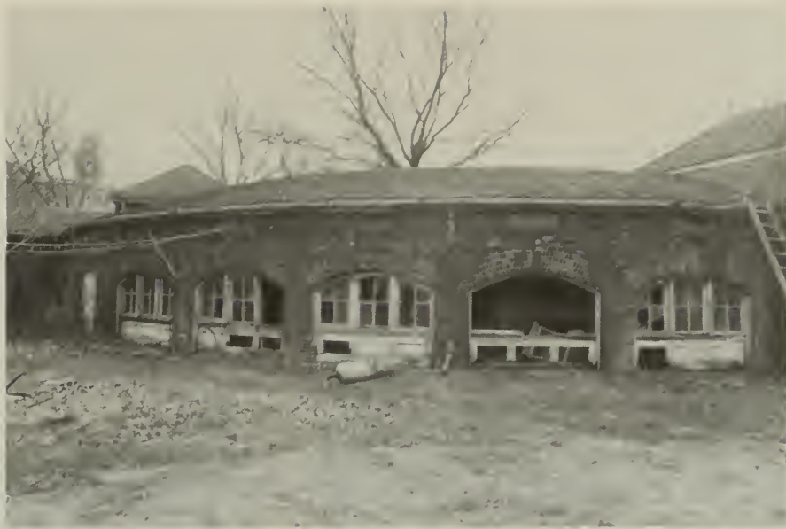
15. Rotting, broken, and missing windows and wood panels, west elevation.
