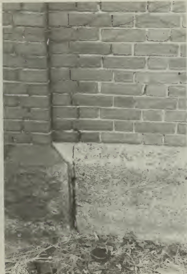
8. Foundation crack at juncture of two-story building with one-story oven room, west elevation.
