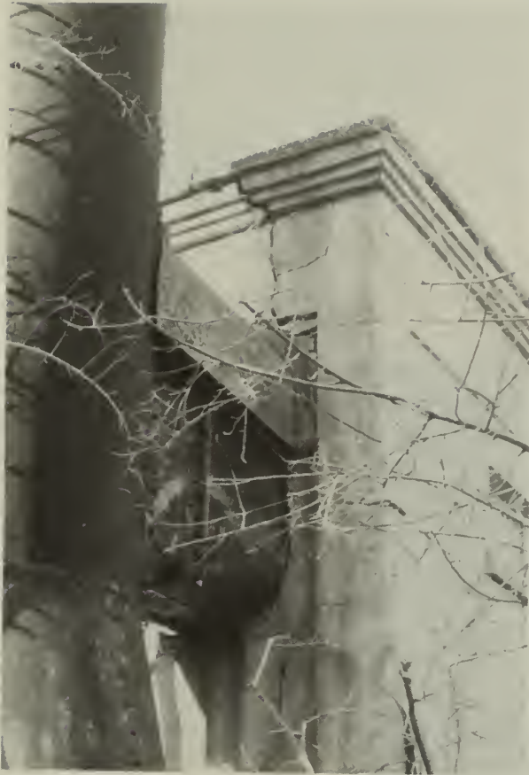
7. Cracking and spalling at east elevation, adjacent to smokestack.
