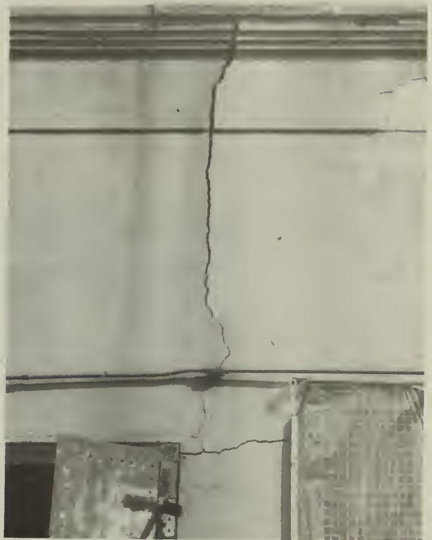
8. Severe cracking, south elevation.
