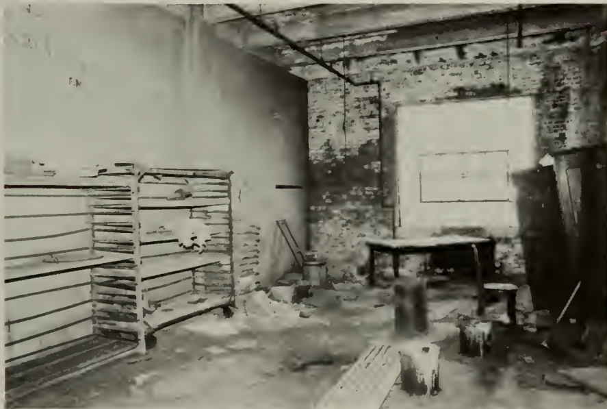
9. Room 202- Peeling paint on brick outside wall, plastered room wall at left, wood flooring.
