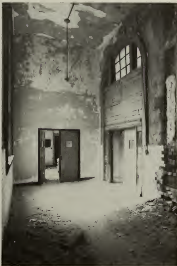
13. Room 101- deterioration of plaster on wall at right and of ceiling parging.
