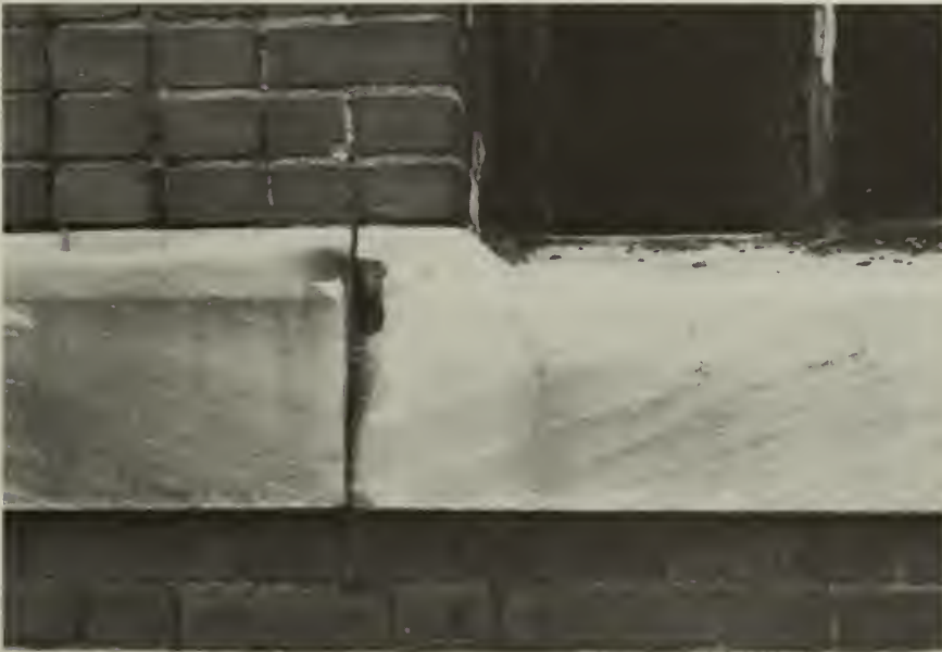
12. Spalling at limestone window sill joints.
