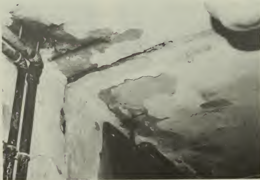
17. Severe transverse ceiling cracks and vertical wall cracks on second floor of C-2.
