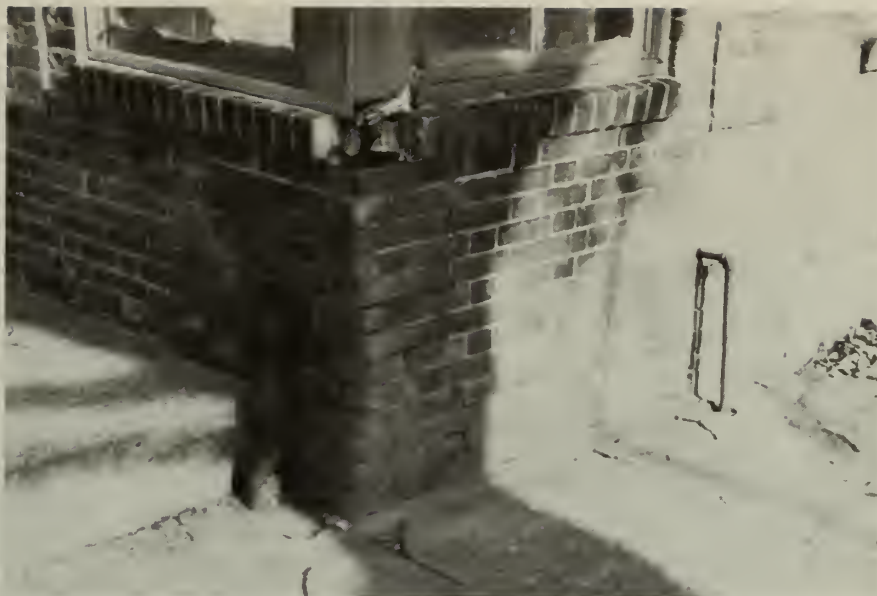
11. Missing brick at corner of window sill, northeast pavilion.
