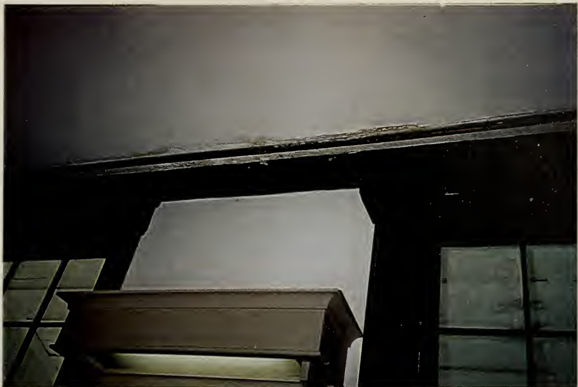
Photo shows damage (in the corner where the wall meets the ceiling) caused by penetration of rainwater from the corner of the middle dormer in the south into the roof and eventually to the ceiling.
