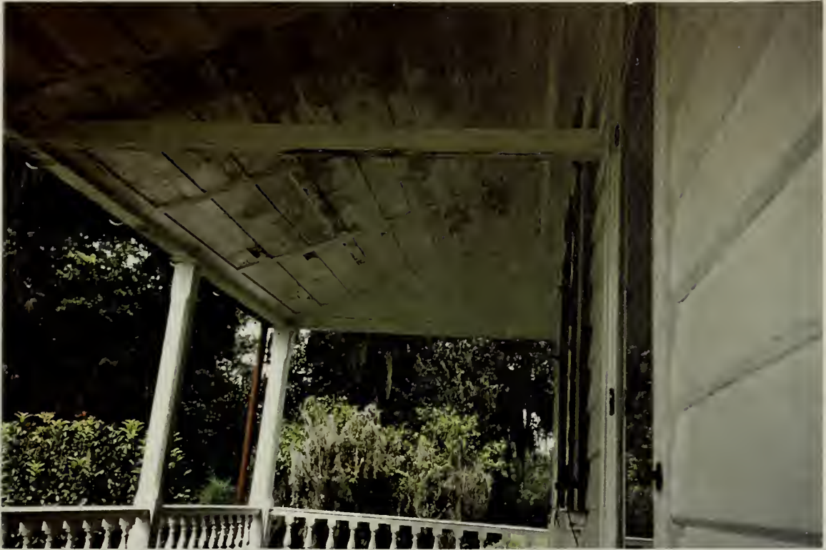
Mildew damage on the paint surface of the south porch ceiling , similar to this is on the surface of the gable in the east and west part of the main building.
