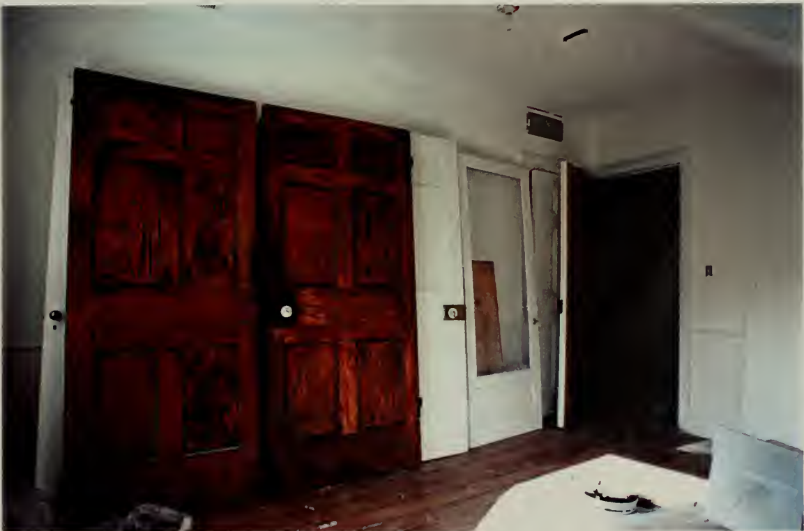
Photos show the original doors that belong to the southeast and southwest rooms on the first floor in the main building. Note the entrance door is painted on one side and the other side is varnished.
