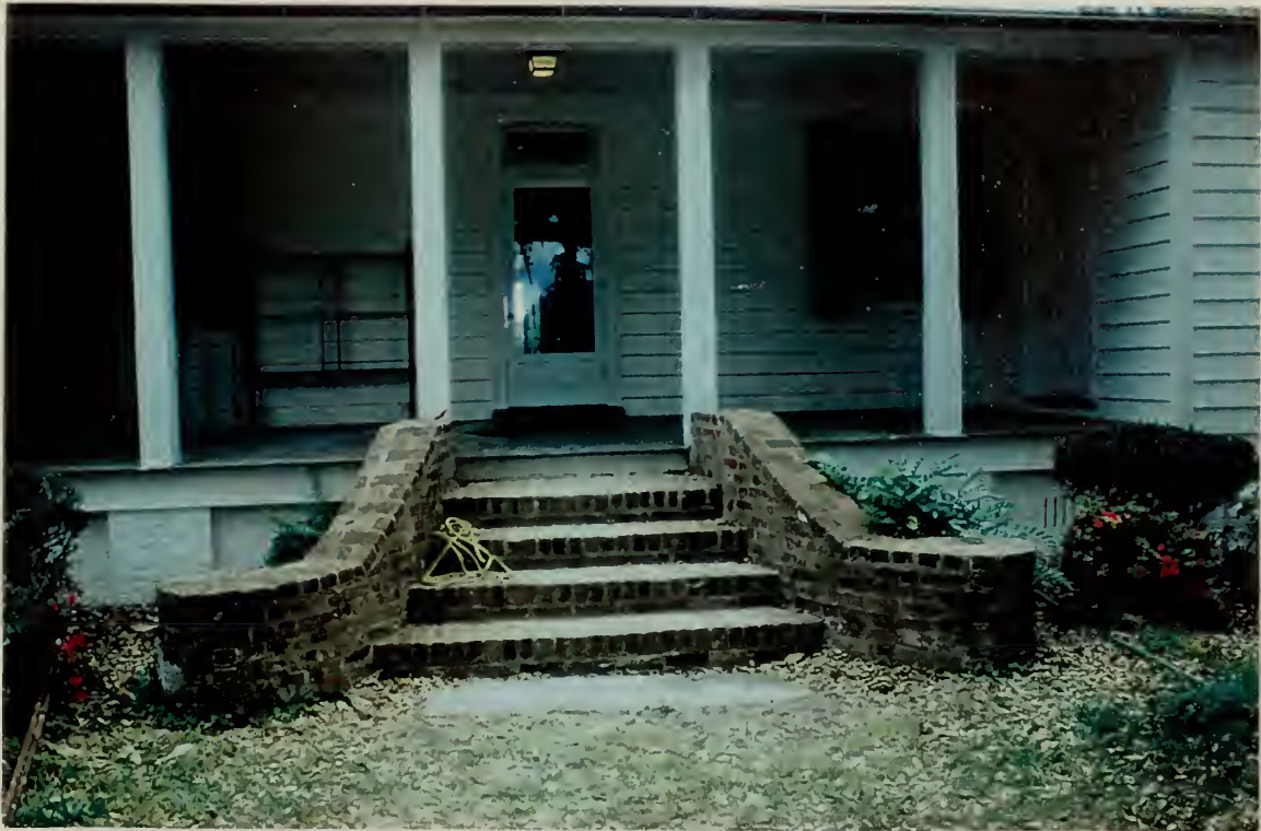
North porch with brick steps and stone treads. The steps at the base extending in a scroll to either side, lead to the porch. Posts are square and handrails and balustrades are removed to repair.
