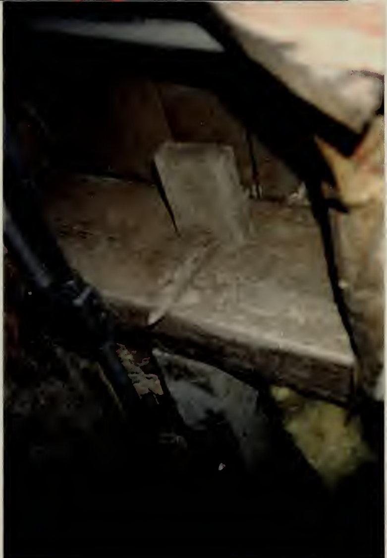
In this photo, note the connection of the floor joists with the girder in the main building. The connection of the floor structural members, as shown in the photo, are mortise and tenon with a wood peg.
