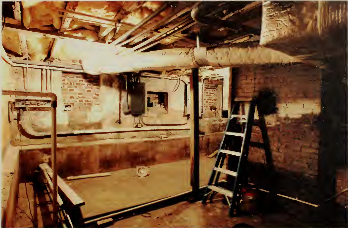
View toward the west of the basement under the west wing. Note basement windows are covered with bricks and the girder supported with a temporary 4"x4" wood post and a jack. Basement openings should be opened to promote air circulation, reduce moisture, and bring some light into the basement.
