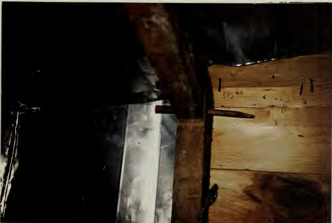
Photo shows the interior part of the main building attic. Note the original wood sheathing and the connection of the rafters. Rafters in the ridge are connected to each other by tenant and mortise with wood peg.
