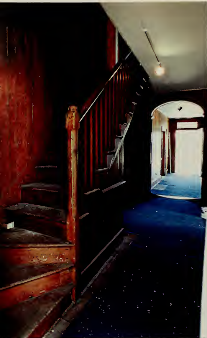
Lower level corridor and the stair in the main building. Note the open well cypress wood stair with plain rounded hand rail, plain square balusters (two per step); a single carved piece with chamfered edge and a round cap newel, and scroll-cut pieces along the sting. All of the woodwork in the corridor and stairs are cypress.
