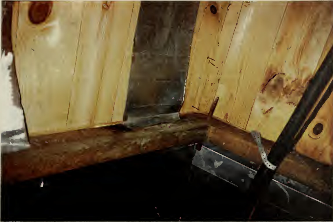
Photo shows the interior part of the main building attic. Note the original wood sheathing and the connection of the rafters. Rafters in the ridge are connected to each other by tenant and mortise with wood peg.
