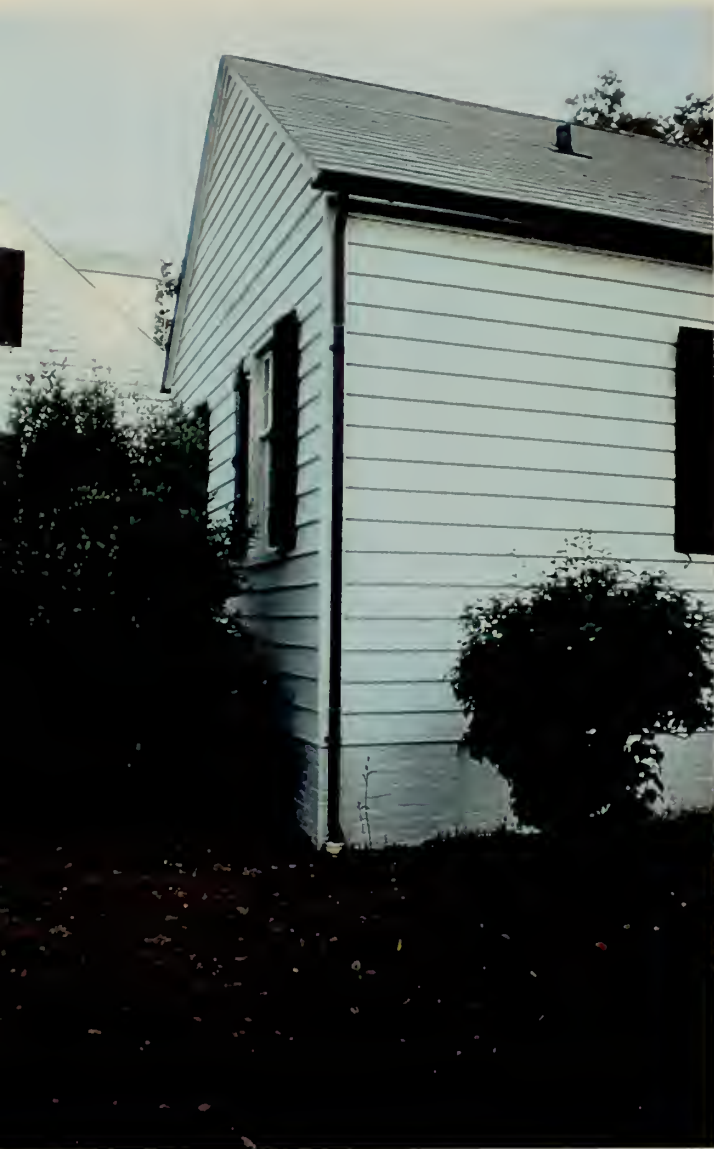
Photo shows the southeast corner of the east wing; note the downspout drains right in the ground adjacent to the brick wall foundation and causes damage.
