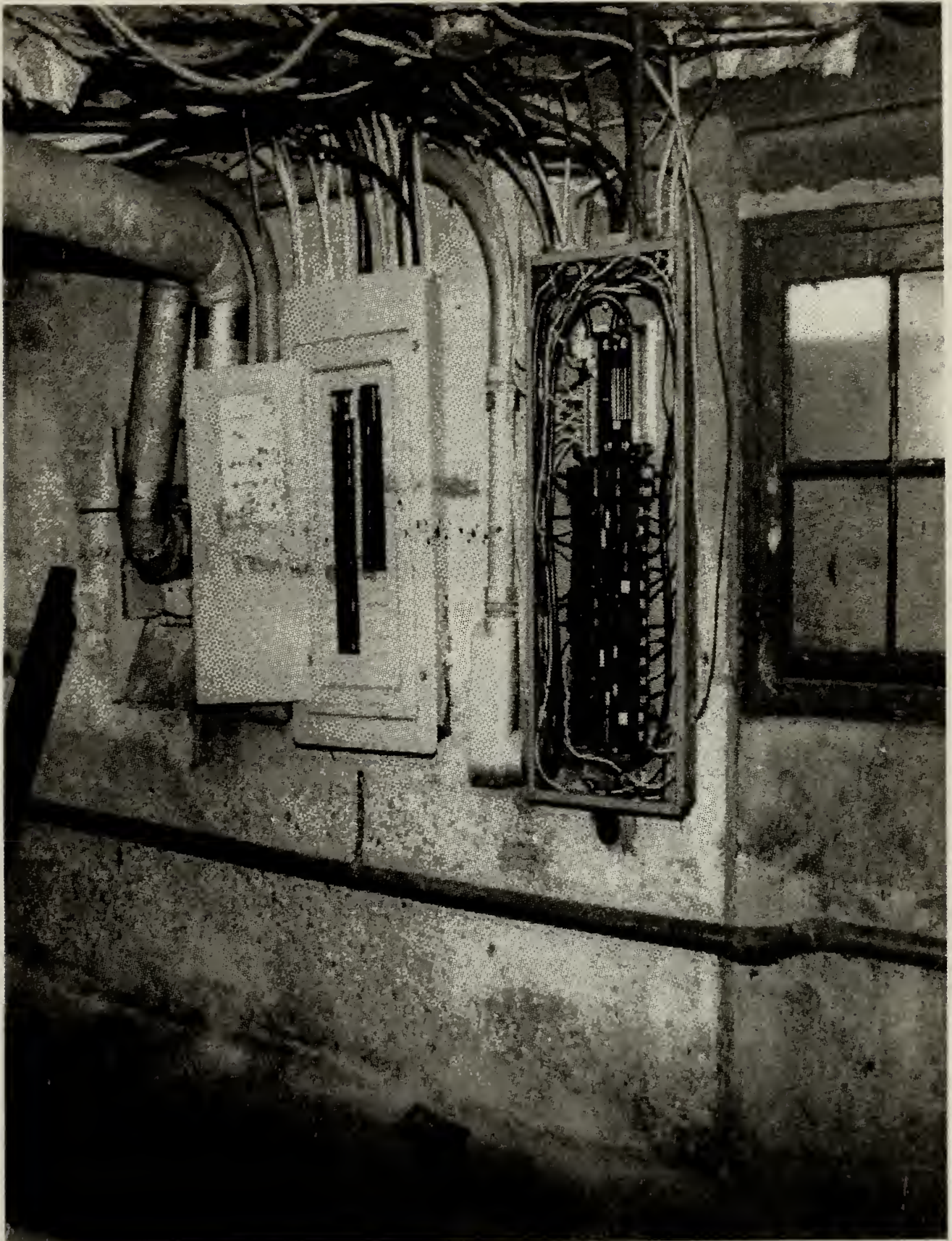
West wall of the basement under the west wing. Note the electric panels and the original window. Windows in this wall have been removed and their openings filled with brick.
