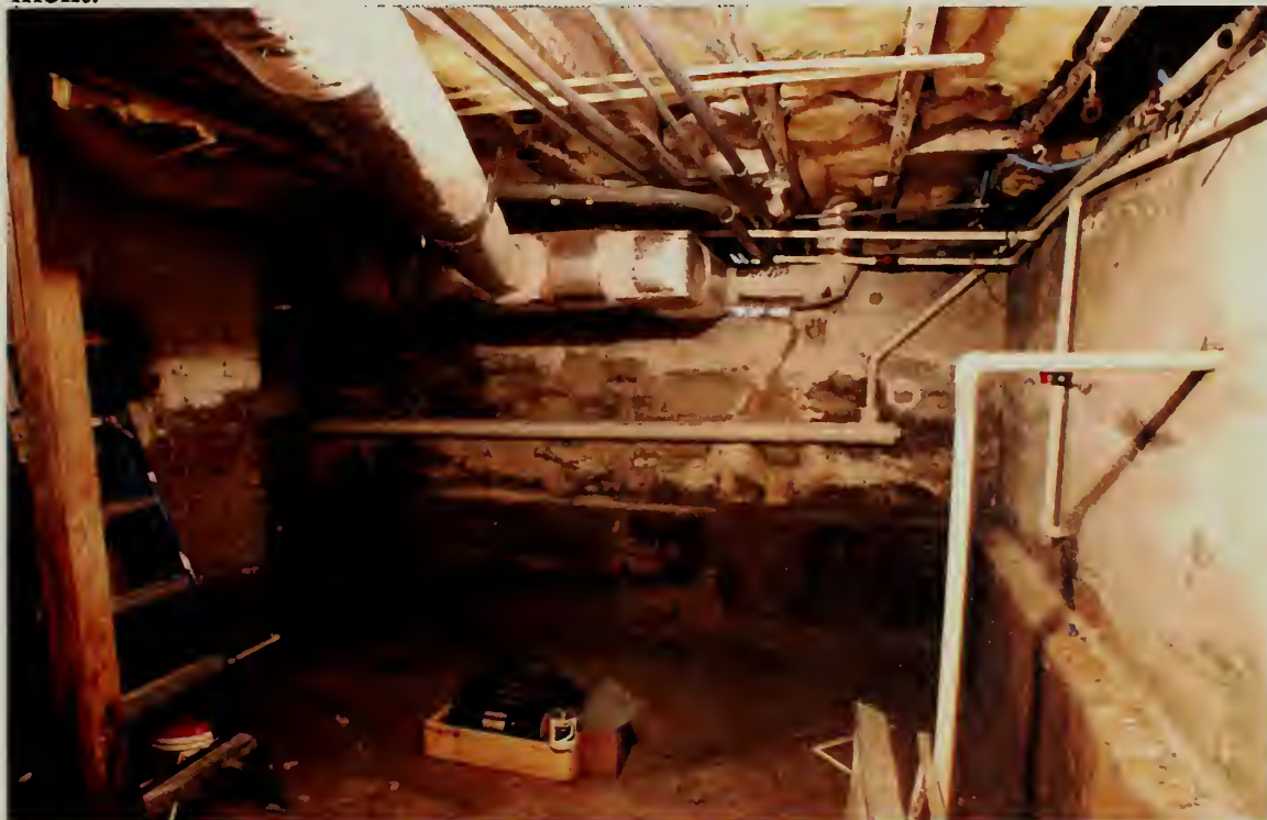
View toward the east wall of the basement under the west wing. Note the surface damage on the concrete wall caused by moisture.
