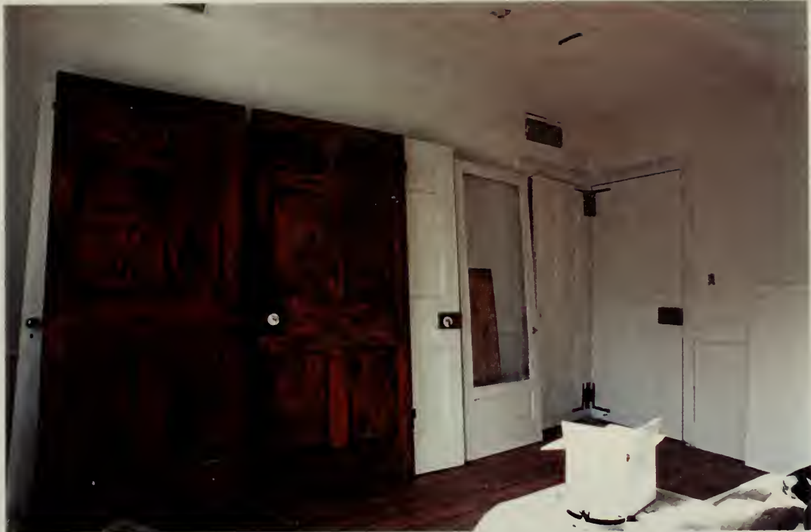
Photos show the original doors that belong to the southeast and southwest rooms on the first floor in the main building. Note the entrance door is painted on one side and the other side is varnished.
