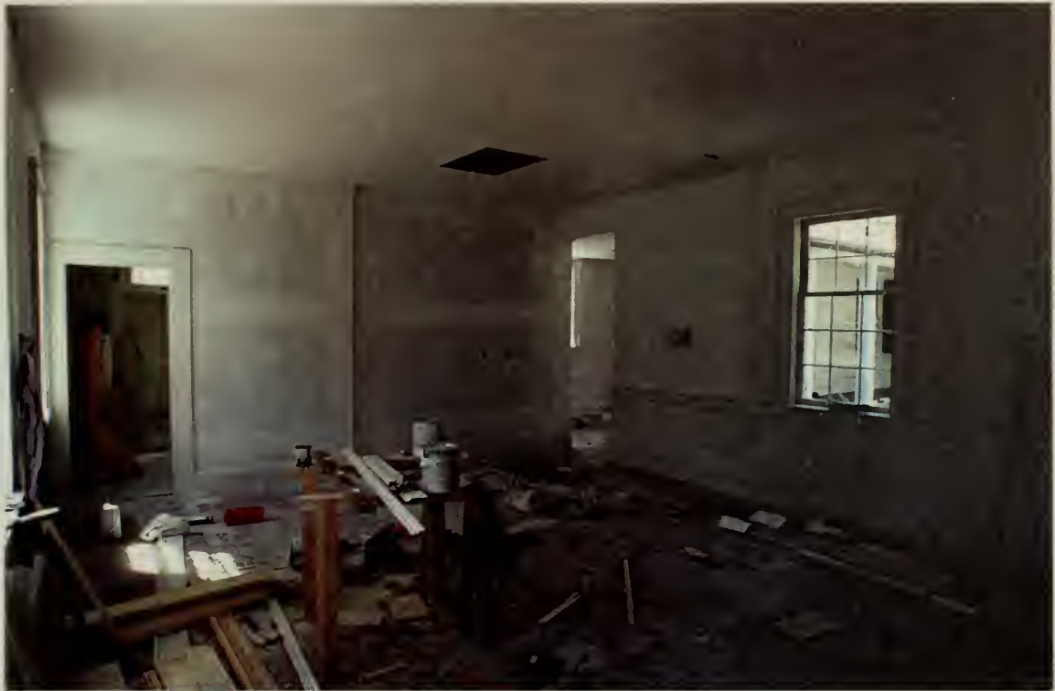
West wing room; Note the access on the left side of picture to the new handicap toilet. The toilet wall is a new sheetrock wall and the ceiling and wall on the right side of the picture are plaster.
