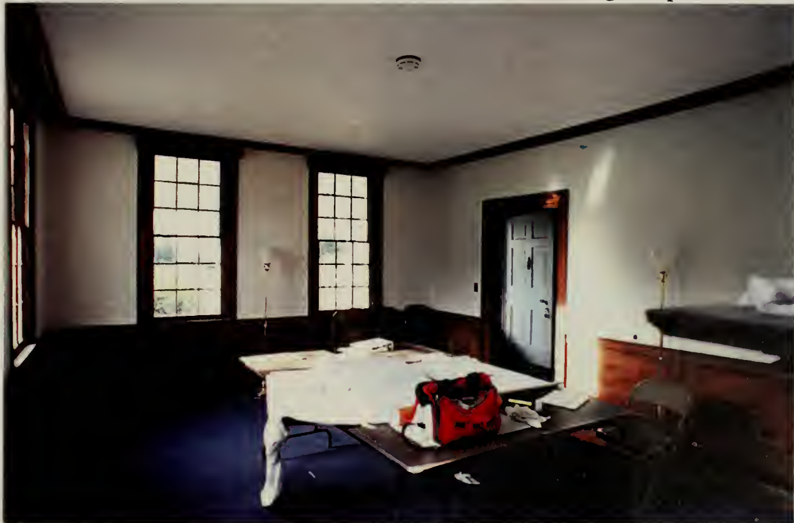
Interior view of the southeast room in the main building. Note the wainscoting, door and window trim with valances, and ceiling molding.
