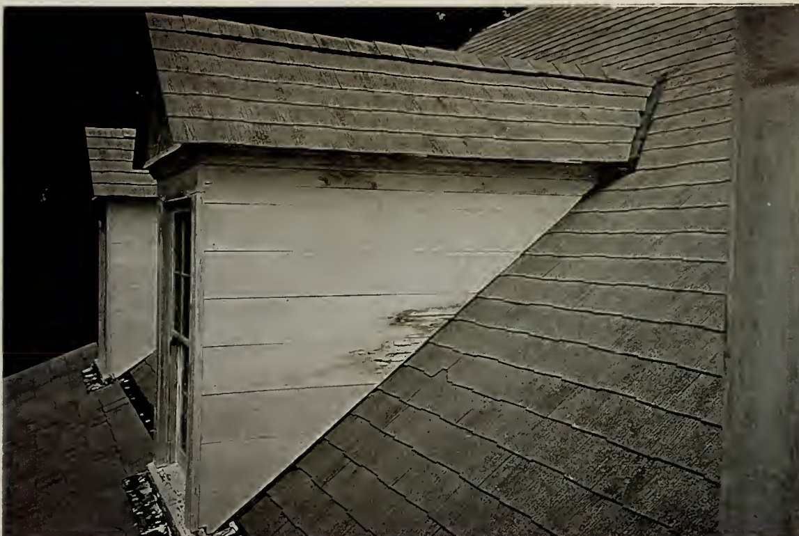
Damaged wood siding on the dormer walls in the south part of the main building.
