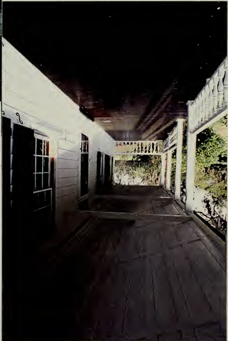
Photo shows the south porch area. Note the floor, ceiling, chamfered posts, handrailing, and balustrade with turned balusters. The wooden floor and it's structure rests on the brick piers.
