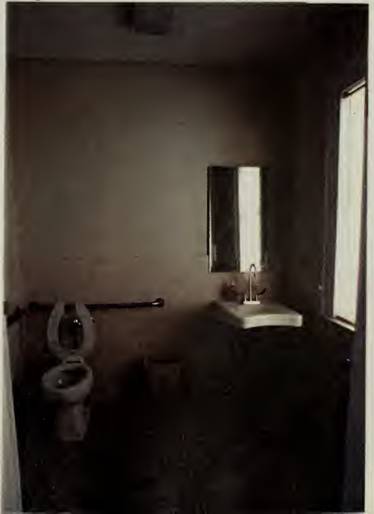
West wing room; Note the access on the left side of picture to the new handicap toilet. The toilet wall is a new sheetrock wall and the ceiling and wall on the right side of the picture are plaster.
