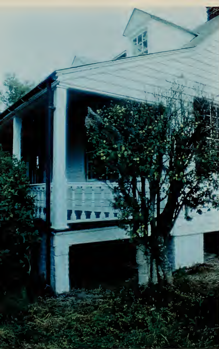
Southeast elevation of the porch. Note the size of the copper gutter and downspout. It appears the size of downspouts are not enough to drain all of the water from the roof. Downspout drains adjacent to the brick pier and causes damage.
