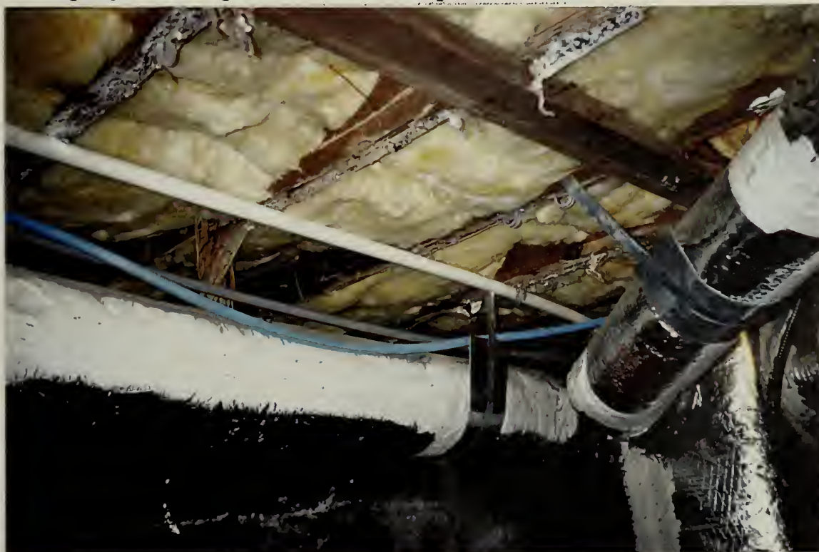
These photos show the termite damage in the joists and girders in the basement ceiling in the west wing in the north part of the brick chimney. These damaged joists and girders need to be replaced with new.
