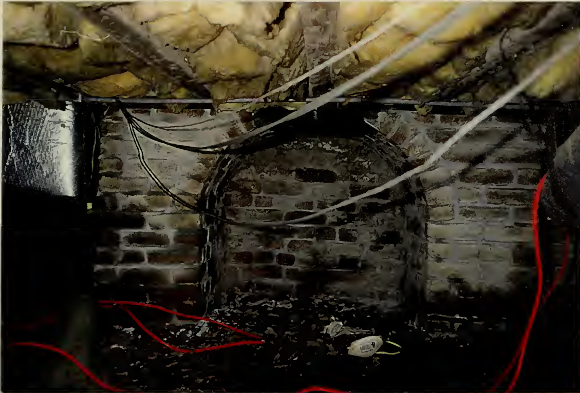
Photo indicates the fireplace foundation in the crawl space and the batt insulation inserted between the joists of the first floor in the main building.
