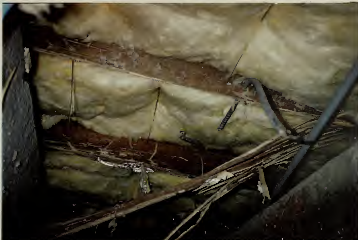
These photos show the termite damage in the joists and girders in the basement ceiling in the west wing in the north part of the brick chimney. These damaged joists and girders need to be replaced with new.
