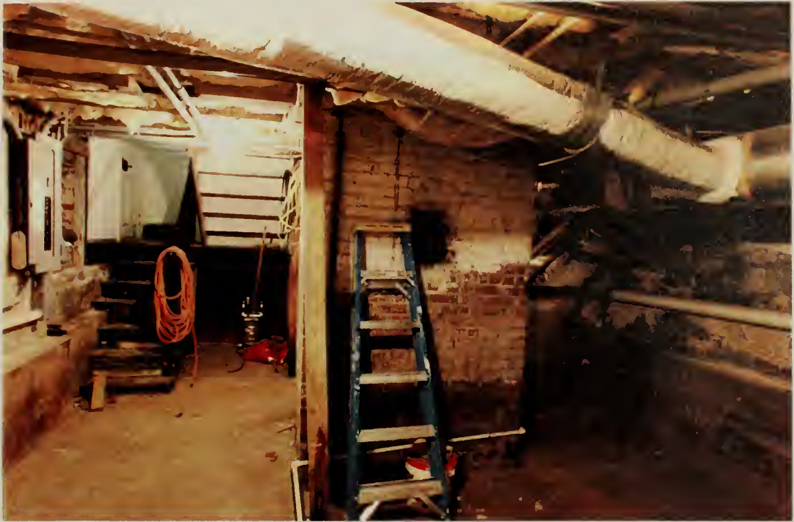
View of the basement toward the north. Note the basement stair on the left of the picture and the unaligned post under the girder adjacent to the brick chimney and ladder.
