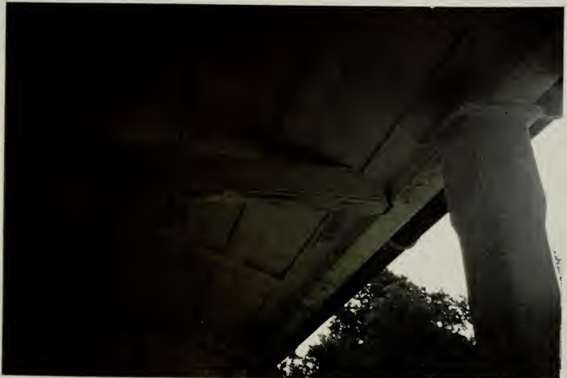
Mildew damage on the paint surface of the south porch ceiling , similar to this is on the surface of the gable in the east and west part of the main building.
