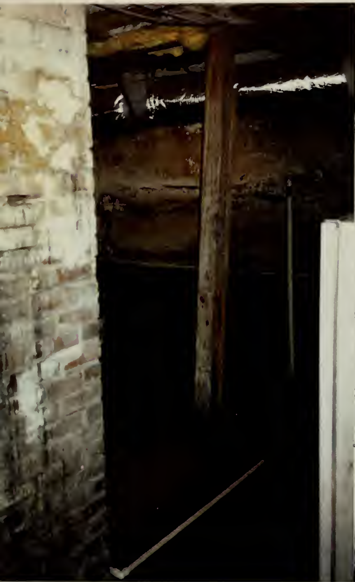
Photos show basement joists in the south part temporarily supported with an un-aligned post and a metal jack close to the brick chimney
