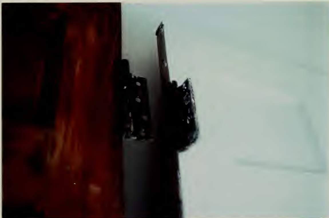
Photo shows the original metal swivel hinge on the room's entrance doors in the main building.
