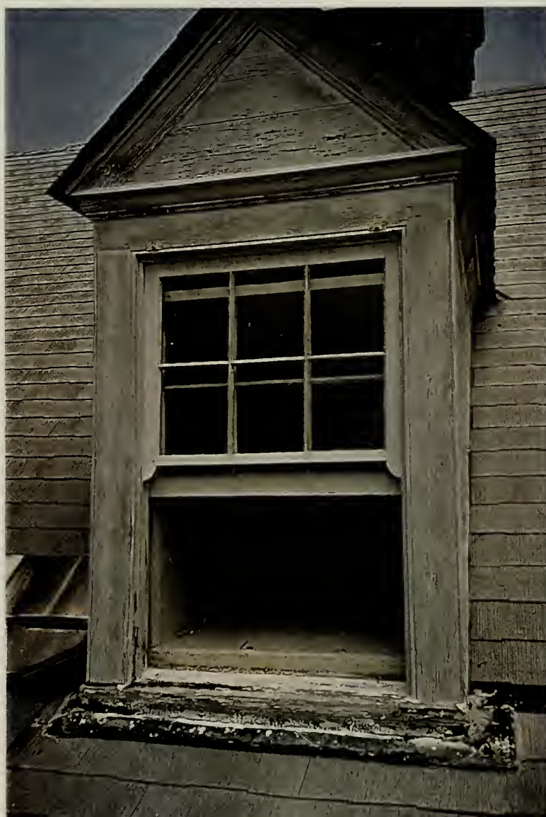
Damaged wood siding on the dormer walls in the south part of the main building.
