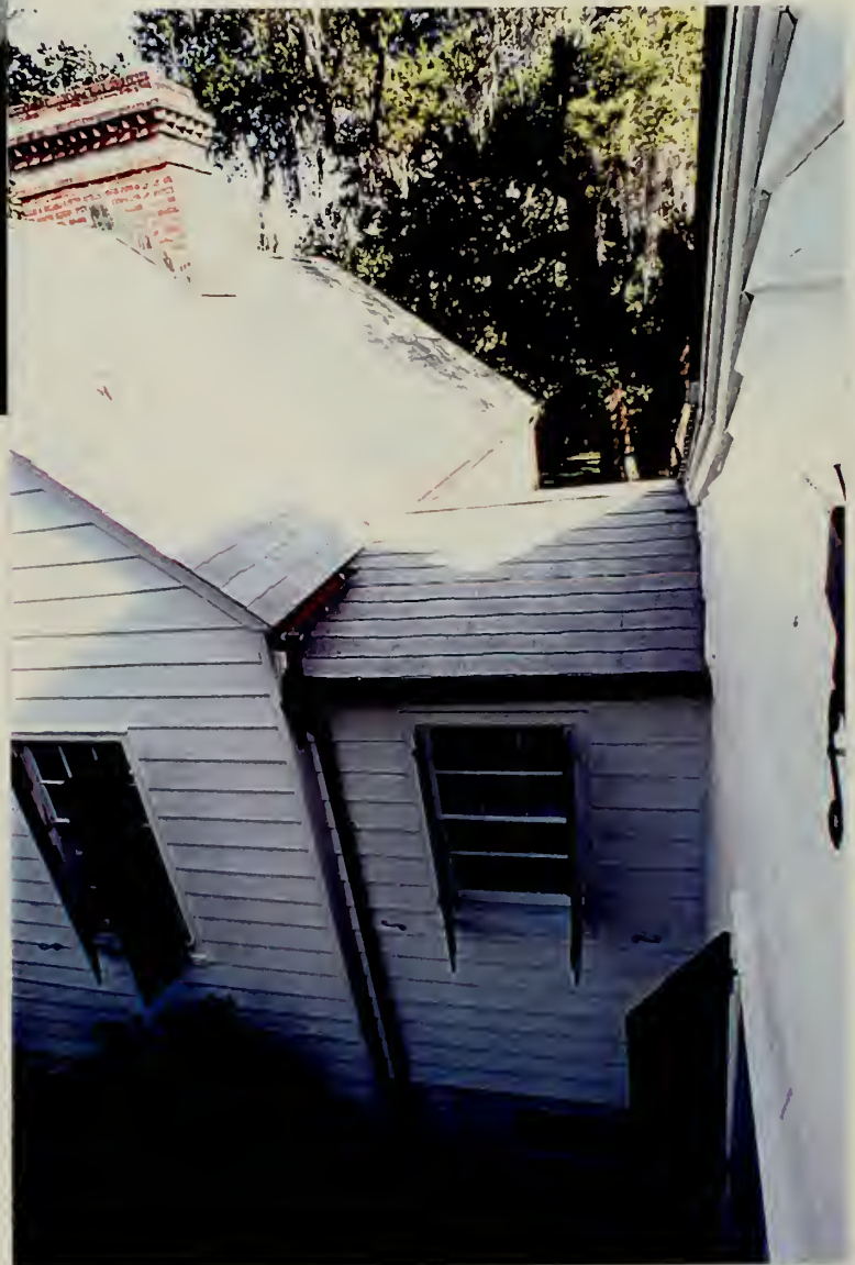
Photo shows the detail of the connection of the main house to the west wing. Note pitch of the roofs and the size of the downspout, which is typical for the main building and the wings.
