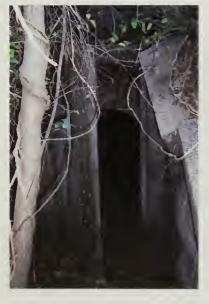
Figure 3.30: The exterior entry of the Battery Catlin parados (BS-8) built in c.1865, looking east showing granite cheek walls and overgrown conditions. SUNY ESF, 2007.
