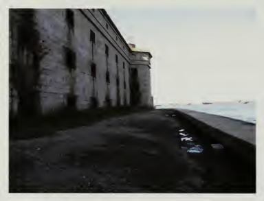
Figure 3.5: The moat space (SO-2), looking north, is filled with earth and rubble and top-dressed with gravel between the granite seawall (BS-2) and the fort walls. SUNY ESF, 2006.
