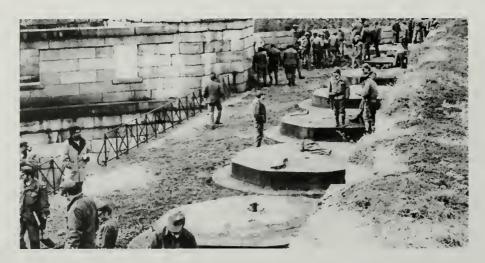
Figure 1.67: A 1970 photograph looking northwest across the barbette tier of Battery Weed showing a National Guard crew completing a landscape maintenance detail. Prior to this work, the barbette tier was overgrown with scrub and trees. Note shell of fort's magazine in the background. Unnumbered photograph, Gateway National Recreation Area Archives, Fort Wadsworth.
