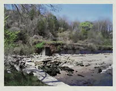
Figure 3.35: The partially vine-covered concrete seawall (BS-13) built in c.1938, view looking northwest with Battery Catlin in the background. In the foreground is a collapsed section of the granite seawall. SUNY ESF, 2007.
