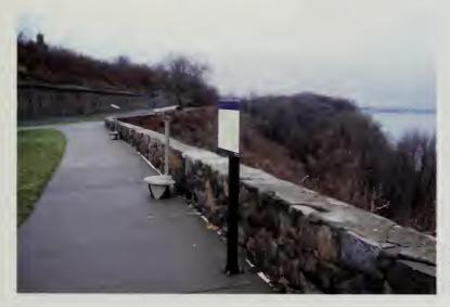
Figure 3.32: The overlook stone wall (BS-10) built in c.1938, view looking north along the overlook terrace. The wall measures approximately 2,000 feet in length. SUNY ESF, 2007.
