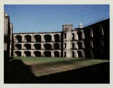
Figure 3.4: The parade ground (SO-1) view looking northeast, is enclosed by a half-hexagon of arched granite casemates with two four-story stair towers and guardhouse on the west side. SUNY ESF, 2006.
