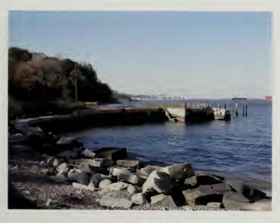
Figure 3.27: The north dock (BS-6), built in c.1859, looking northwest with remains of the 1907 timber extension. In the foreground is a collapsed section of the granite seawall. SUNY ESF, 2007.
