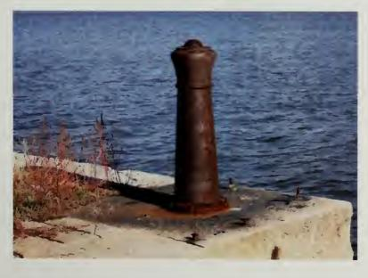
Figure 3.51: One of the two iron dock bollards (SS-11) that probably date to the original c.1859 construction of the north dock. SUNY ESF, 2007.
