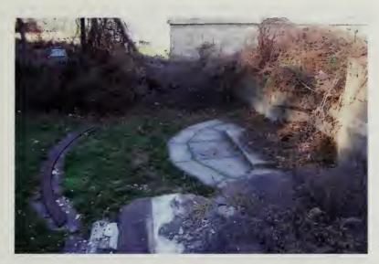
Figure 3.31: The gun emplacement (BS-9) at Battery Bacon (see T-3) built in c.1898 looking north showing concrete platform and parapet walls, iron pintle, and traverse circle. SUNY ESF, 2007.
