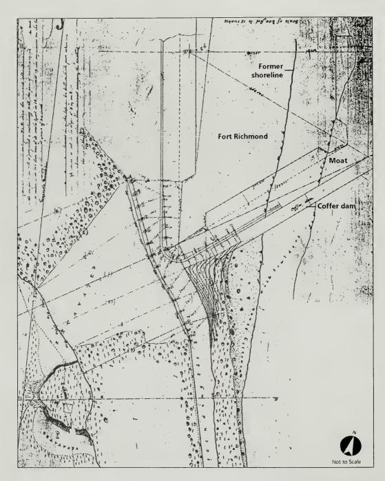
Figure 1.25: Plan titled "Sketch of the ground adjoining the south west salient of Fort Richmond (Staten Island) and the hill with a proposed wall to sustain the foot of the its slope," 1848. The plan shows the proposed graded portion of the bluff above the southwest bastion of the new Fort Richmond. RG 77, Dr 43, Sht. 12, Cartographic Division, National Archives II, College Park, Maryland, annotated by SUNY ESF
