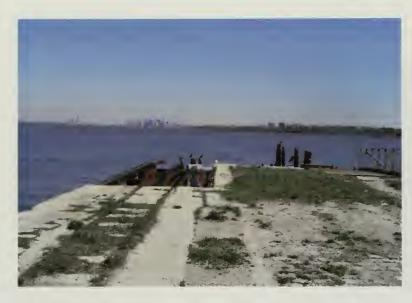
Figure 3.28: The north dock (BS-6), built in c.1859, view looking northeast showing granite and concrete surface, and remnants of the mine railway and timber extension dating to 1907. SUNY ESF, 2007.
