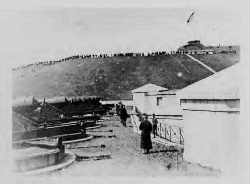
Figure 1.47: A photograph taken in 1890 looking southwest toward Fort Tompkins showing the barbette tier of Fort Wadsworth (Battery Weed) with its rotating guns still in place. The objects below the guns are rammers used to load munitions. Uncatalogued photograph, Gateway National Recreation Area Archives, Fort Wadsworth.
