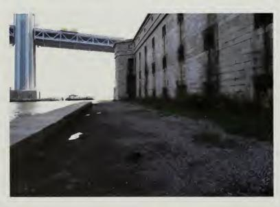
Figure 3.12: The route of the waterfront promenade (C-5), looking south along the granite seawall completed in c.1871 and moat that was partially filled in c.1904. SUNY ESF, 2007.
