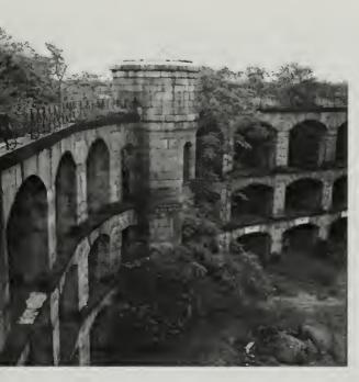
Figure 1.65: Photograph of Battery Weed in 1964 showing poorly maintained conditions that included piles of soil and ruts in the parade ground and volunteer vegetation growing up and over the building. Print 12C02F, Still Pictures Division, National Archives II, College Park, Maryland.
