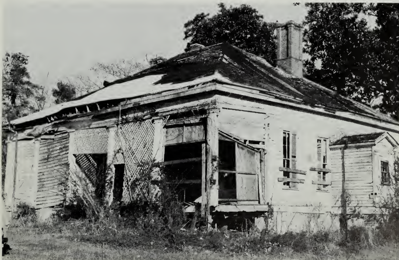
Coker House, Champion Hill Battlefield, Vicksburg vic., MS. This badly deteriorated Greek Revival house is one of the few remaining historic structures on Champion Hill Battlefield. The battle fought here was the precursor to the siege of Vicksburg. An NPS indepth inspection identified the need for major roof, foundation and porch repairs to save this Landmark. Photo by J. Travers.
