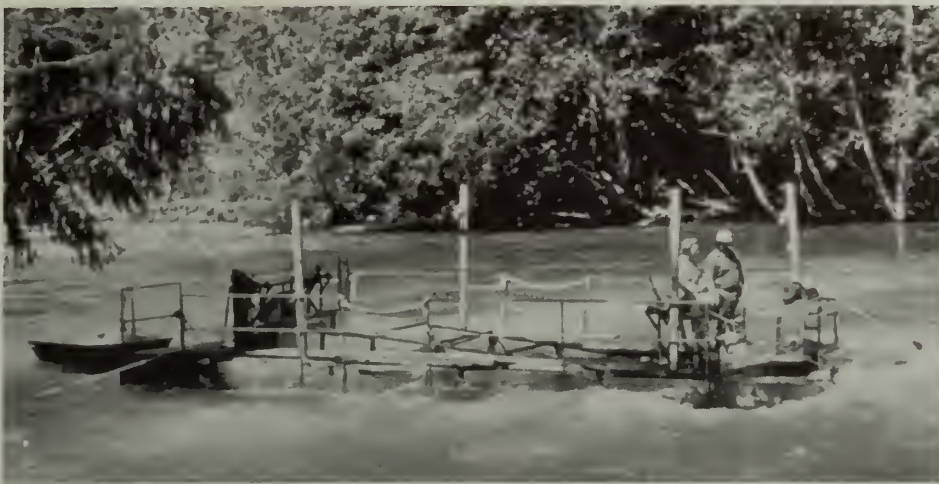
Inclined plane smolt trap operates below the Elwha dam to sample smolt survival.
