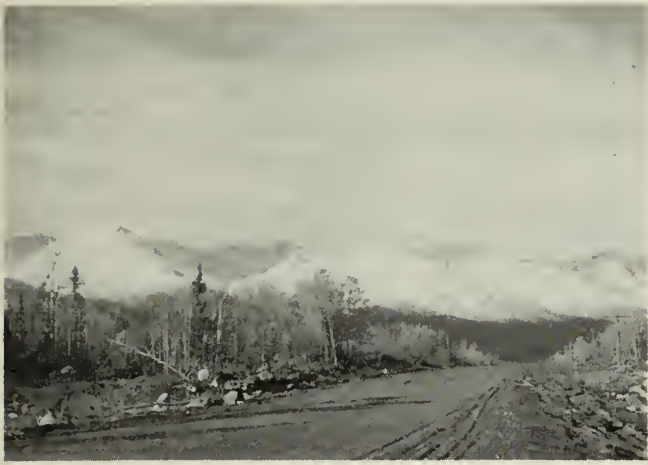
Figure 40.—Alaska Highway, ready for gravel surfacing.
