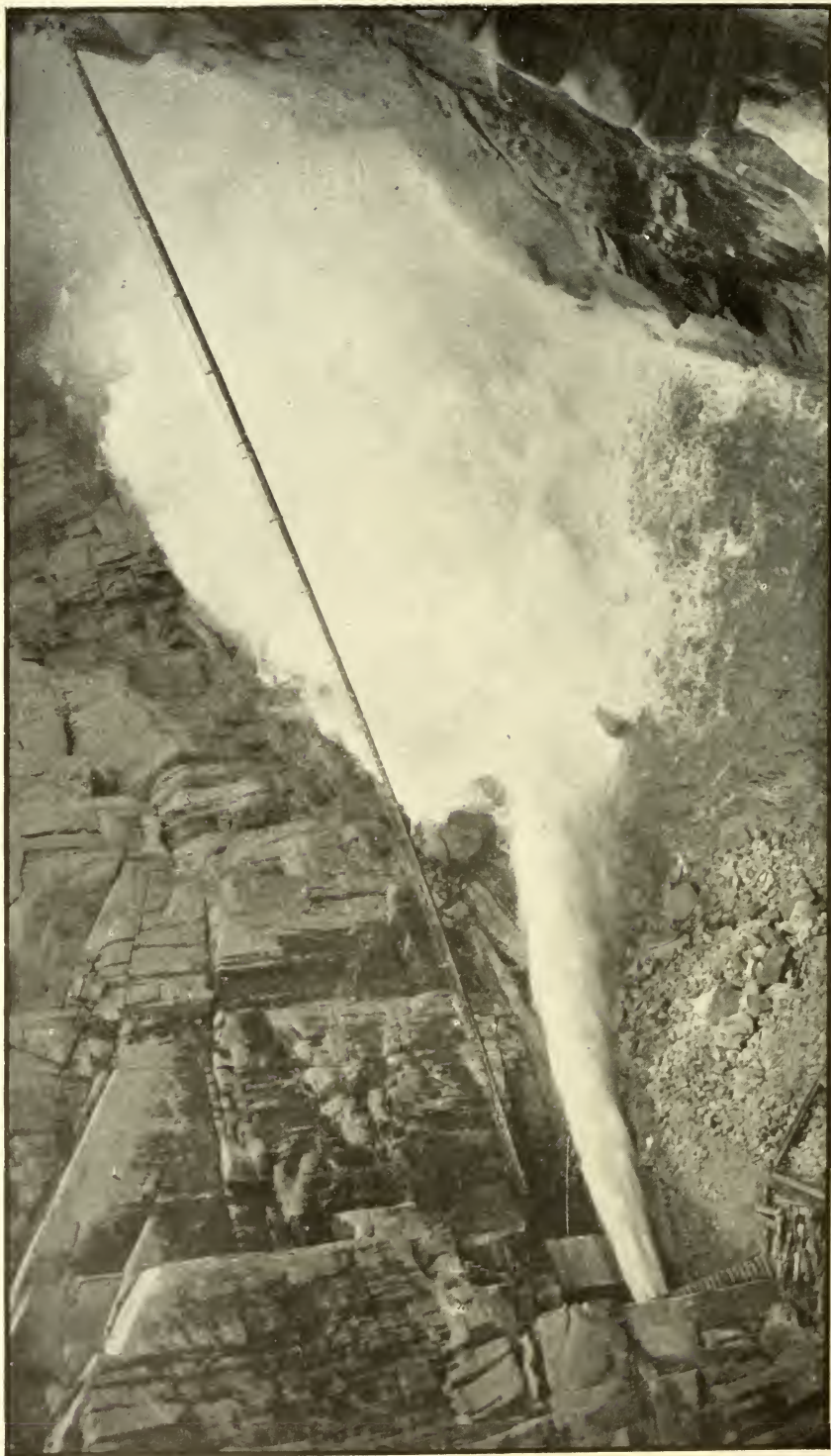
OPERATION OF 58-INCH BALANCED NEEDLE VALVE IN NORTH TUNNEL OUTLET, PATHFINDER DAM.
