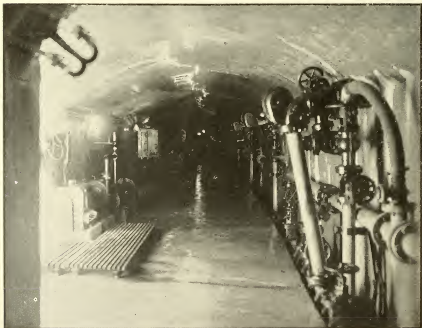
B, BALANCED VALVE CONTROL CHAMBER, ARROWROCK DAM.
