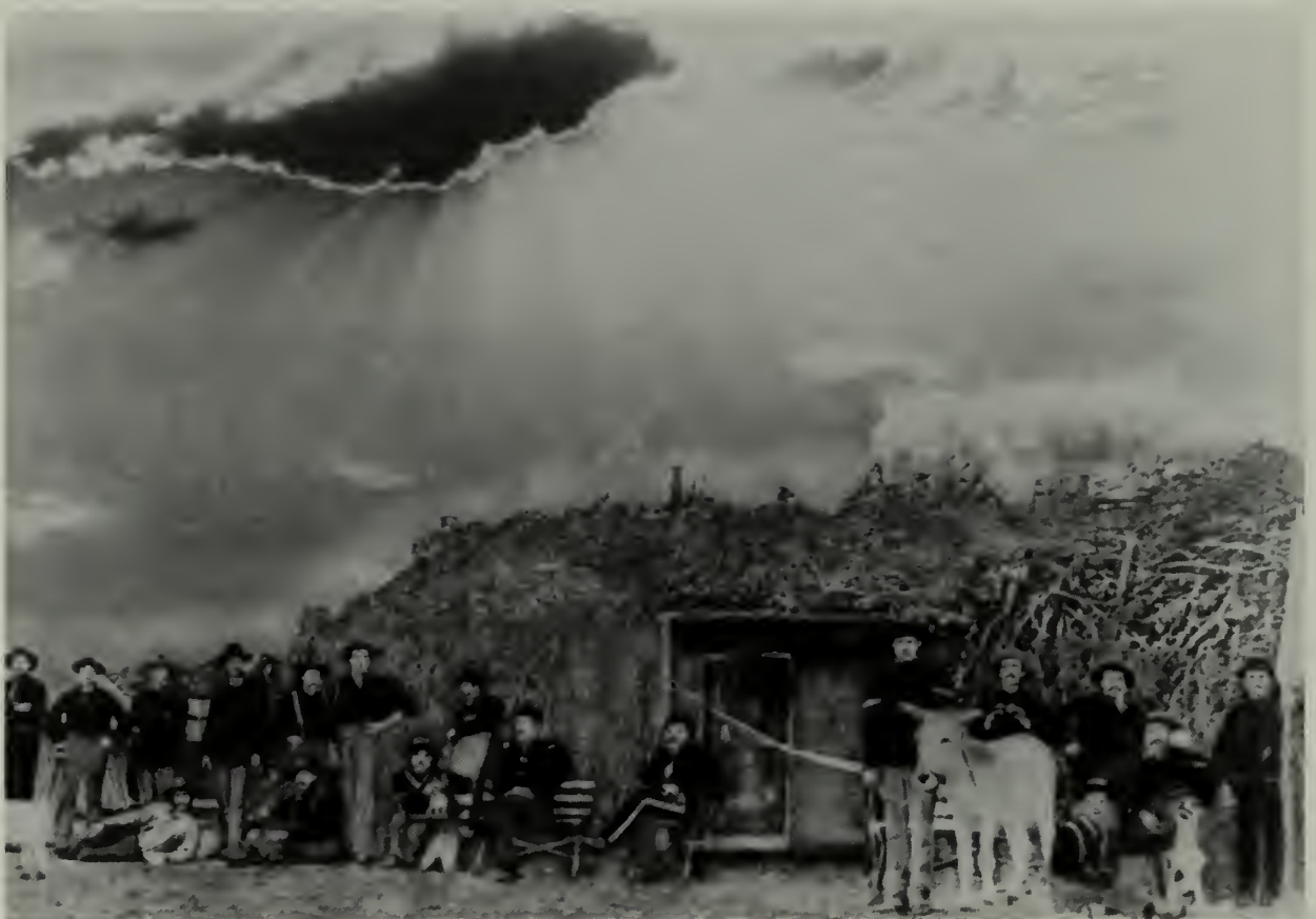
Figure 7. This photograph shows the approximate scale of the earthen fortification as well as some aspects of its construction. This is the south angle of either HS-206 or 207, the enlisted barracks in the redans. The branches overlying the parapet retarded erosion. Log framing outlined the entrance. Fort Union National Monument.
