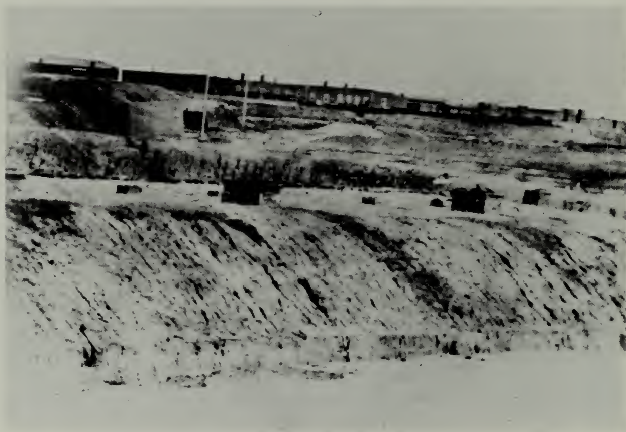
Figure 8. This photograph of the star fort shows the deterioration of the earthwork due to erosion. The brick chimneys pierce the roof of the redan, HS-205, at fairly regular intervals. The Third Fort Union is in the background. National Archives, Still Pictures Branch.
