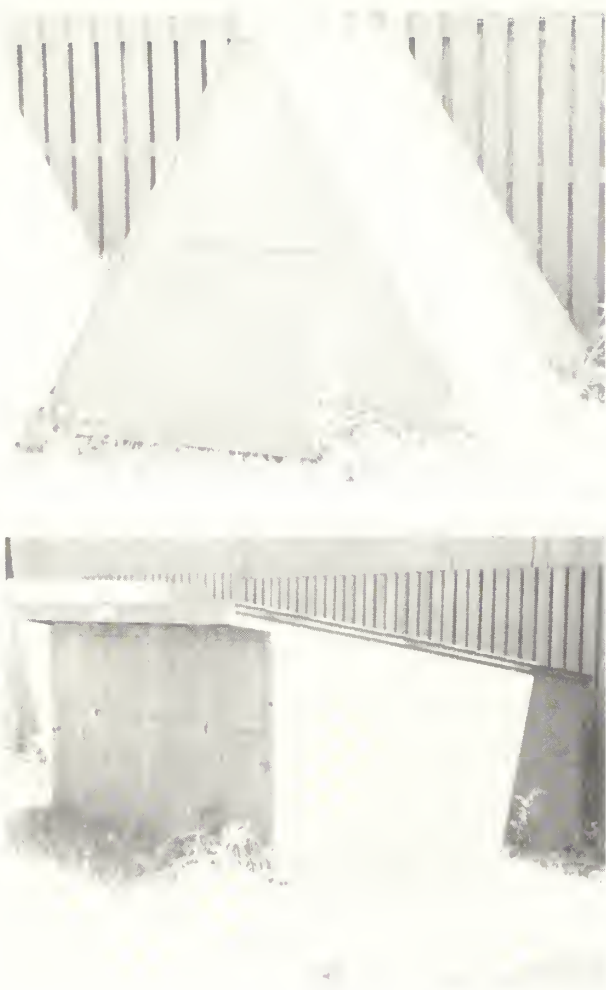
Figure 5.—“A” and shed-type portable hog houses. (Photo courtesy of University of Illinois, Department of Agricultural Engineering)
