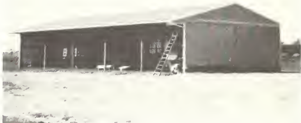
Figure 3.—Machine storage building with wood-pole frame and metal exterior walls. (Photo courtesy of University of Illinois, Department of Agricultural Engineering)
