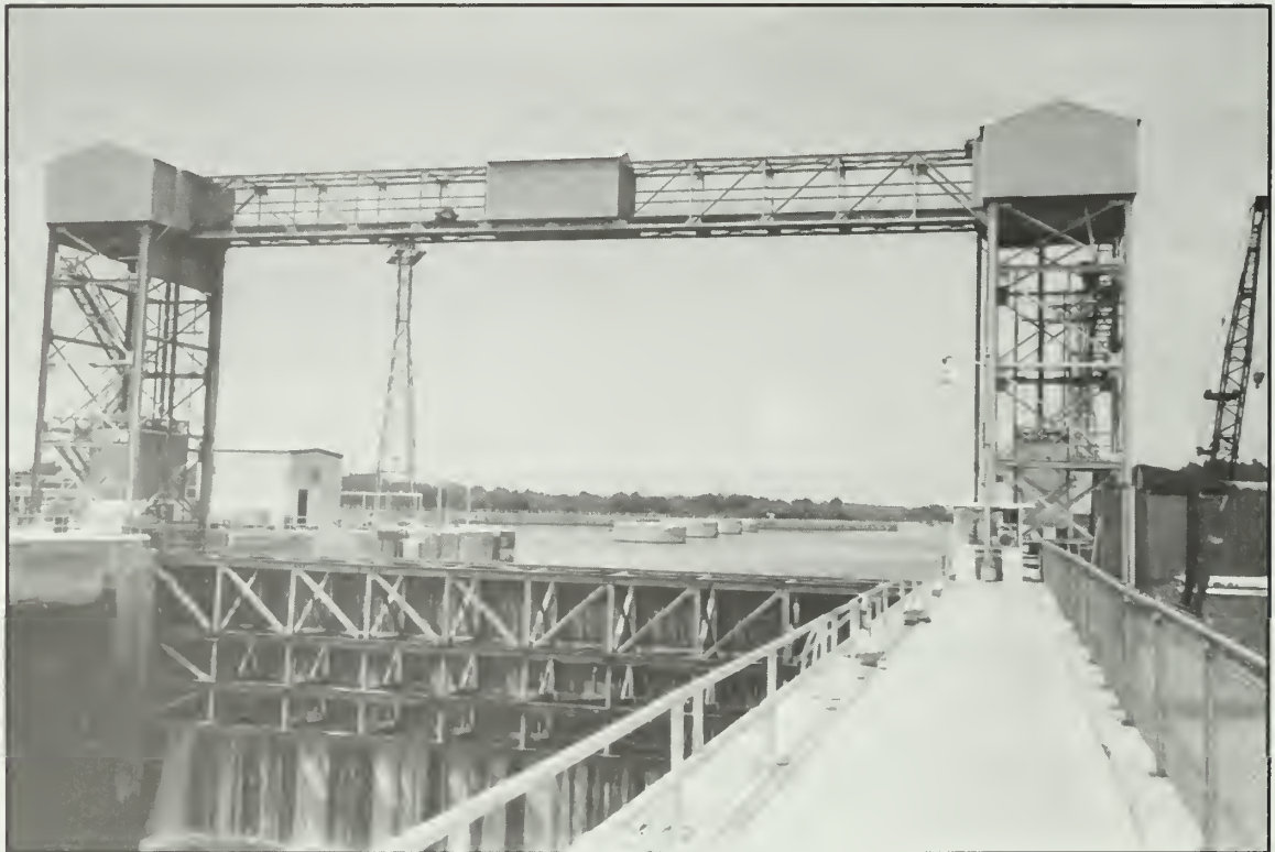
Photo 13. Illinois Waterway: Lockport Vertical Lift Lock (1926), Lockport. Photo by Joseph DeRosa, HAER.
