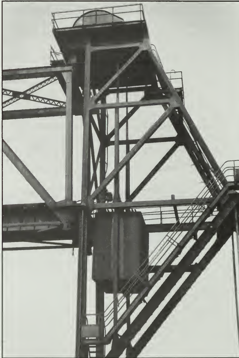
Photo 46. RIRR: Illinois River Bridge (ca. 1900, rblt. 1934) Detail of counterweight, Seneca. Photo by Timothy Whittaker, HAER.
