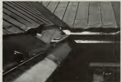
B. Repair roofs and add ice and water shields at eaves and under valleys in cold climates. Photo: Larry D. Dermody.
