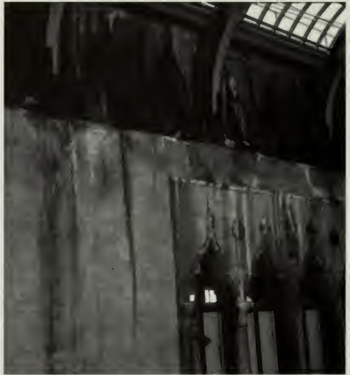
Fig. 7. Condensation dripping from the large overhead courtyard skylight was damaging the masonry in this museum. A new skylight with thermal glazing was installed, replacing the deteriorated single-glazed unit. A new climate control system monitors interior temperature and humidity. Photo: © Isabella Stewart Gardner Museum, Boston.
