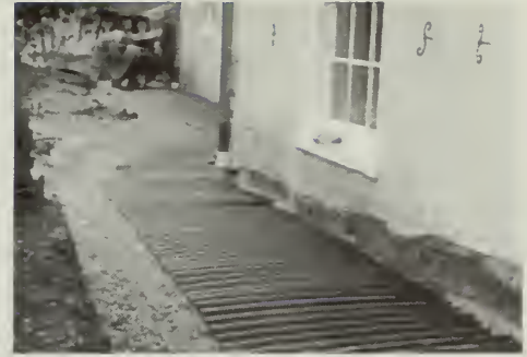
A. Mitigate poor drainage with gravel, filter cloth, or the use of subsurface drainage mats under finished paving. Photo: Larry D. Dermody.
