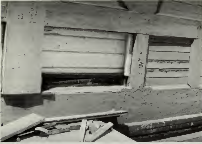
Fig. 8. Damaging moisture conditions can occur during construction. Peeling paint on this newly rehabilitated frame wall was attributed to wall insulation that had become wet during the project and was not discovered. Photo: NPS Files.
