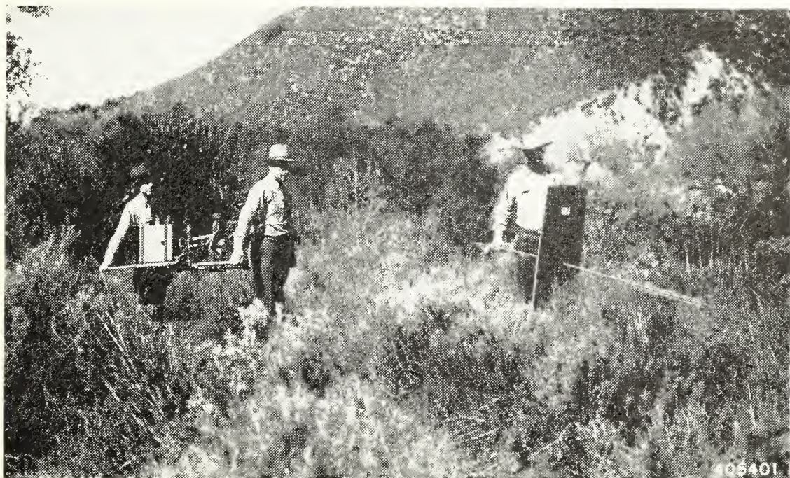
Los Padres portable flame thrower in use as a stretcher-type unit. Note the protecting shield.
