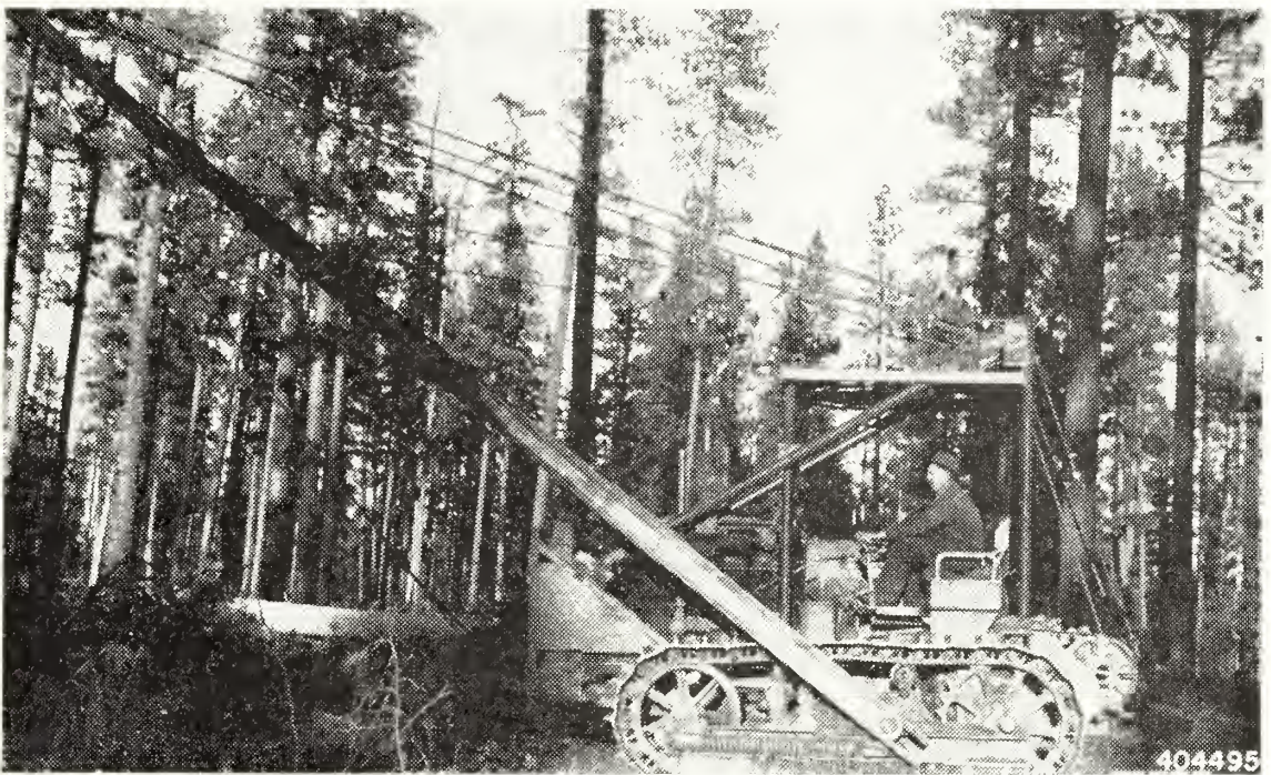
Side view of pusher snag-felling machine used on the Deschutes National Forest.
