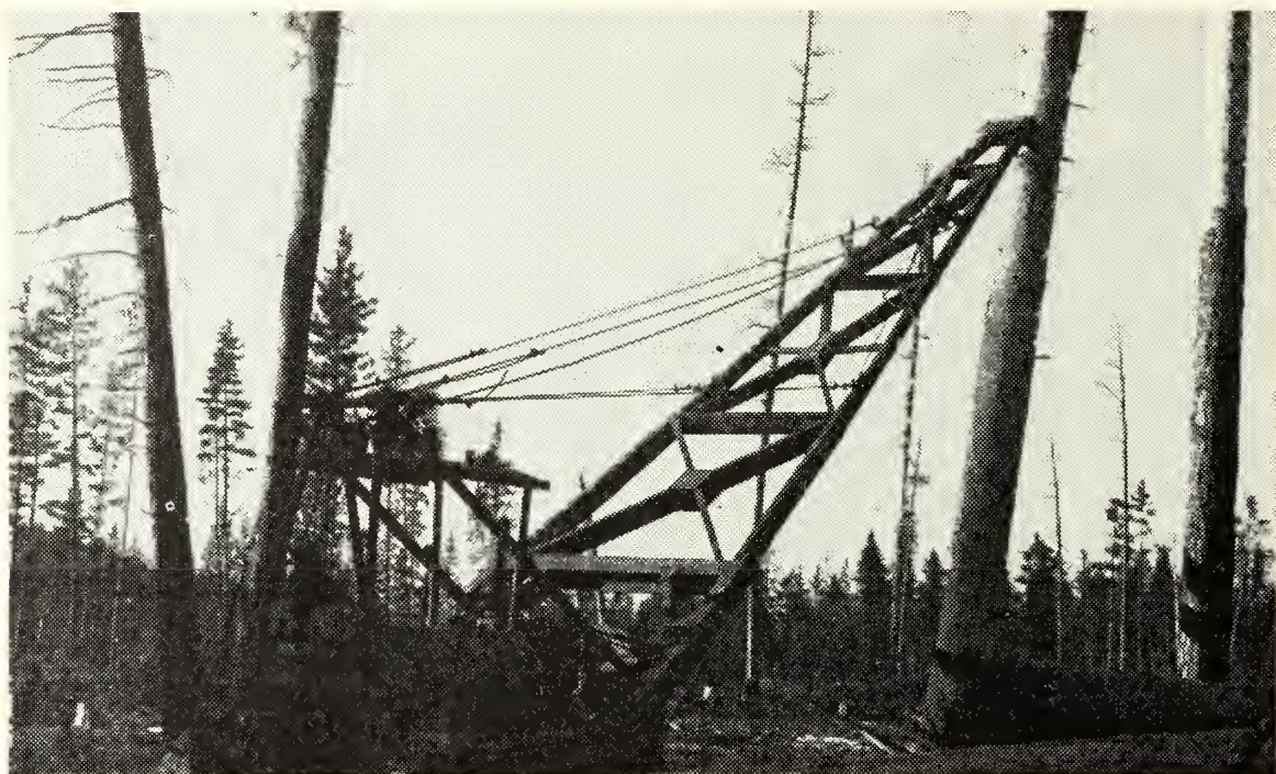
The Deschutes snag-felling pusher in action.
