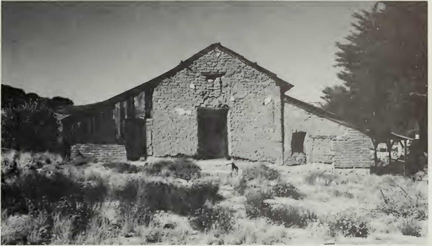
Warner's Ranch, San Diego County, CA. This 1849 adobe ranch house is the major focus of Warner's Ranch, best known for its historic role as a Butterfield Overland Mail stage station from 1859-1861. Adobe walls and roof are deteriorating. An NPS indepth inspection identified needed repair work for this vacant structure. Photo: Courtesy, Gilbert Arnold Sanchez, Inc.
