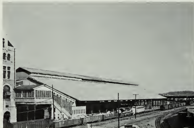
Nashville Union Station and Trainshed, Nashville, TN. The station's trainshed is the largest, single span, gable-roofed trainshed in America. The structural system developed for the trainshed made a significant contribution to the evolution of modern building methods. The trainshed has been vacant for several years, damage to the structural system is accelerating, and new owners are considering moving or tearing the structure down. Above left: Romanesque Revival train station. Above right: Trainshed. Below: Interior of trainshed illustrating steel trusses and I-beams. Photos: Courtesy, Historic American Buildings Survey, NPS.
