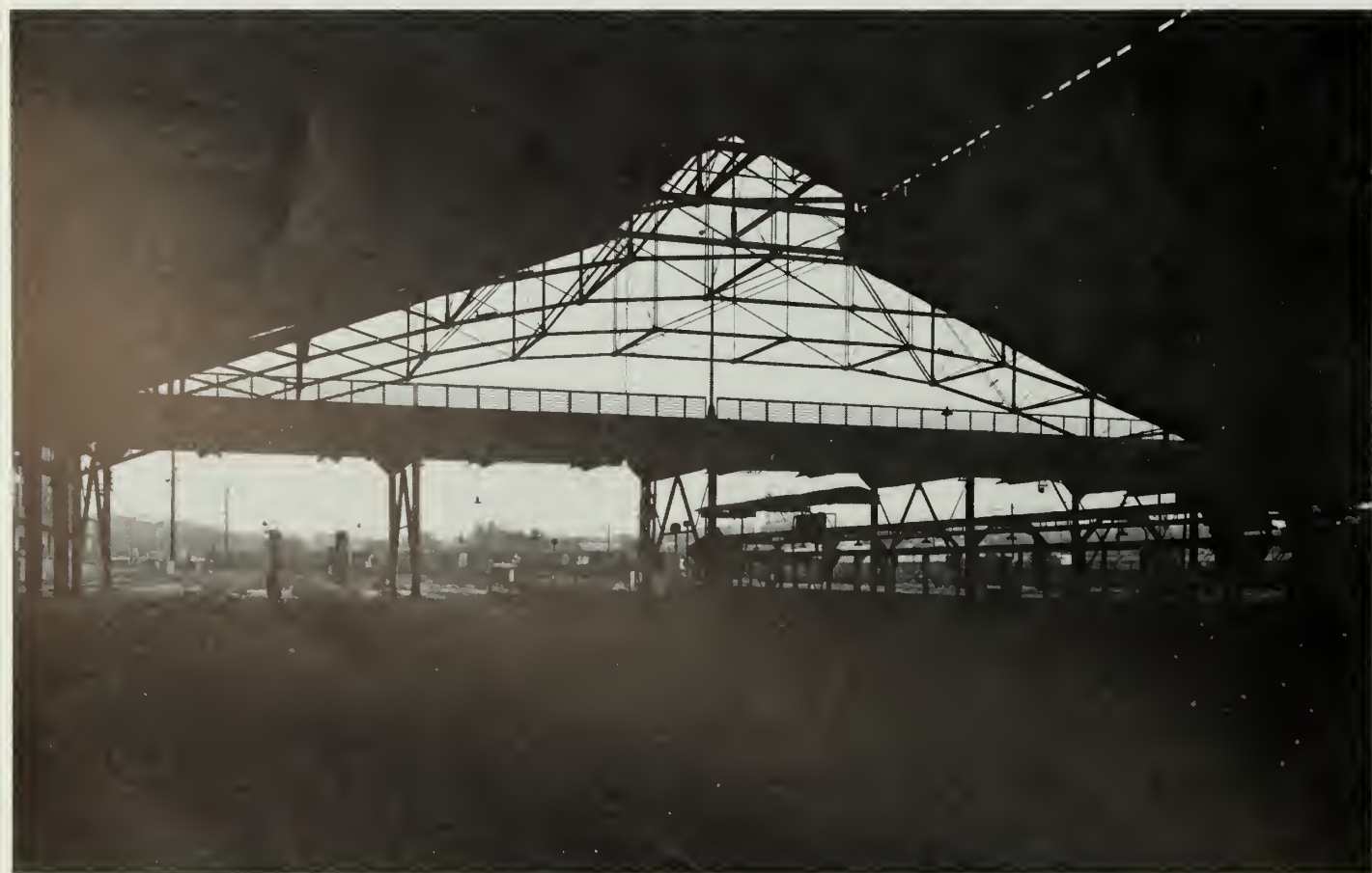
Nashville Union Station and Trainshed, Nashville, TN. The station's trainshed is the largest, single span, gable-roofed trainshed in America. The structural system developed for the trainshed made a significant contribution to the evolution of modern building methods. The trainshed has been vacant for several years, damage to the structural system is accelerating, and new owners are considering moving or tearing the structure down. Above left: Romanesque Revival train station. Above right: Trainshed. Below: Interior of trainshed illustrating steel trusses and I-beams. Photos: Courtesy, Historic American Buildings Survey, NPS.
