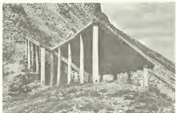
Figure 2.—A jet roof located above the lee slope. Winds trapped between the roof and the terrain are accelerated enough to prevent cornice formation.
