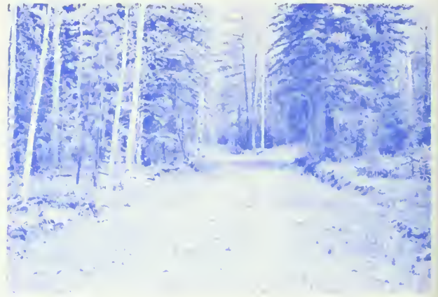
Figure 4.—Graded road with berms and ditches protect the stream channel in White Spruce Gulch.
