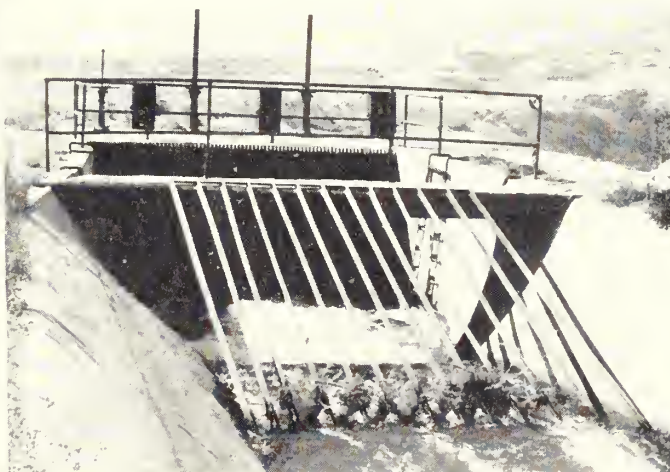
STEEL BARS DO NOT A PRISON MAKE —they are a means of escape from canals. Above, reinforcement bar mats and an escape ramp on the side slopes of the North Branch Canal, Kittitas Division, Yakima project, Washington. At right, handrails and escape ladders at the Jordan Narrows Siphon of the Provo River project, Utah. Photo above by S. T. Larsen, Denver, Colo.; at right by R. W. Reitz, Region 4.
