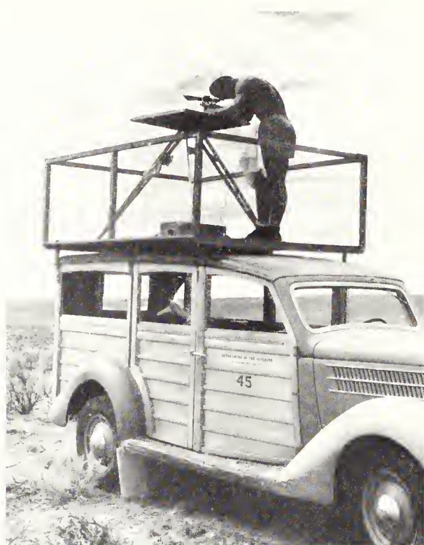
SURVEYING THE LAND in the heat of the August 1937 summer, using a platform on top of a station wagon to improve the topographic view of the Columbia Basin. Photographer unknown.
