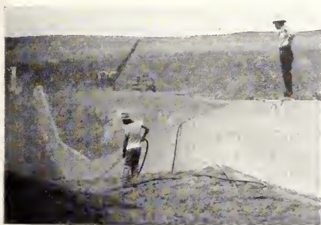
SOUTH DAM'S CONCRETE CORE (below) with "Pot" O'Donnell supervising men to the left who is cleaning up the bedrock. At center, below, the old highway through the Grand Coulee as the water gradually rose in the ice-age channel of the Columbia River. A new highway skirts the east wall of the Coulee. At right, O'Donnell is dwarfed by the giant outlet channels which release water from South Dam into the Main Canal of the project. Photos below by H. W. Fuller, photo at right by F. B. Pomeroy. Both are Region 1 photographers.
