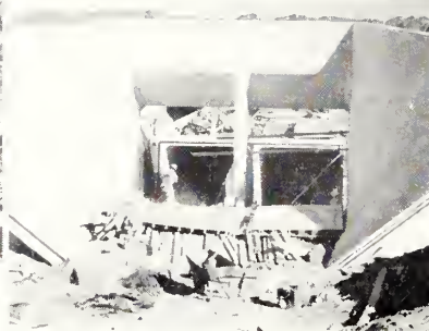
THE FIRST STRETCH —Check and turn-out for the first 8½ miles of the canal (above) and the Wash Siphon (at right). At extreme right, moving the lining machine over the Siphon.
