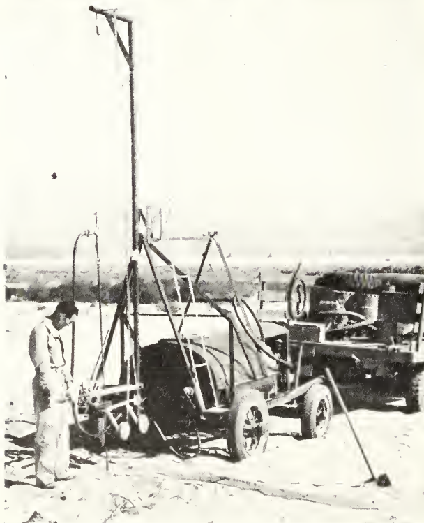
THE PROBE —At top, the hydraulic rotary drill and coring rig used to extract samples and dig observation wells at 42 sites in Coachella. Below, a Coachella Valley County Water District employee installs a piezometer by means of the jetting process. Top photo submitted through the courtesy of the United States Salinity Laboratory, Riverside, Calif.
