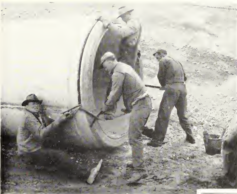
RUBBER GASKETS on the spigot ends of the 20-foot concrete sections of the big water pipe made it water-tight (see above). At upper right, columns supporting the Terminol Reservoir roof. At right, covering Terminol Reservoir No. 2 with a slob roof.
