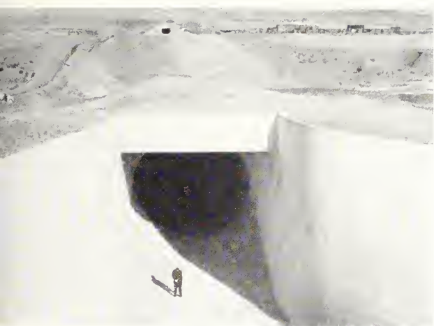
SUBWAY SYSTEM on the West Canal where water travels underground through dry Coulee siphons No. 1 and No. 2, as part of the 60-mile-long route taken by Columbia River on its way to irrigate project lands. Photo by H. E. Foss, Region 1 photographer.
