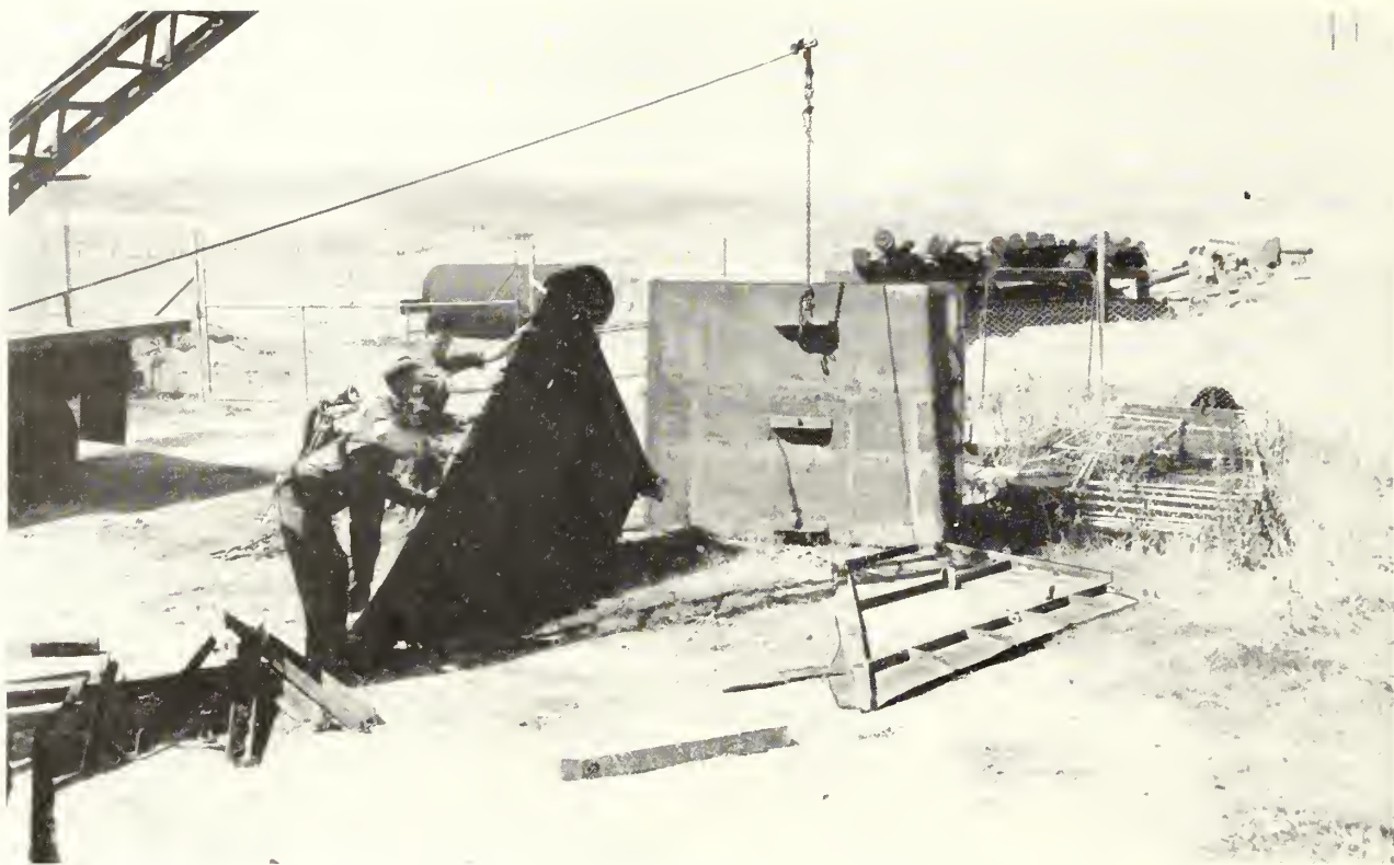
EASY TO ASSEMBLE. —A Contra Costa maintenance crew assembles the newly developed cofferdam in a short time, to meet an emergency.
