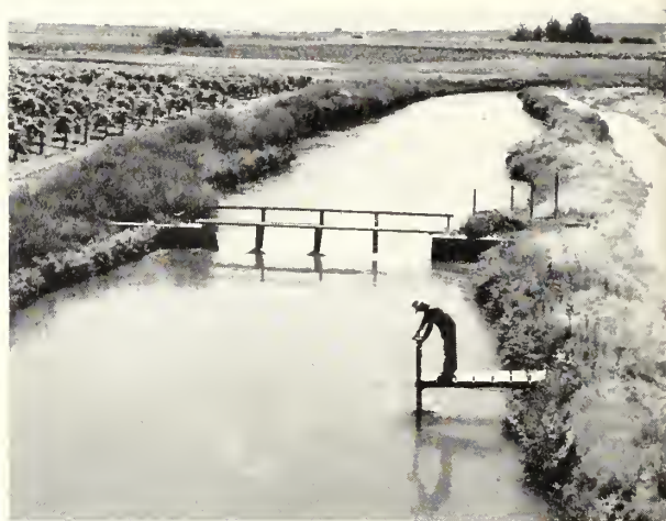
BEWARE OF THE VACUUM! —At left, note the rectangular opening in front of the pipes. When water in Colorado-Big Thompson's Hartsaath Feeder Canal rises above normal, the siphon spillway goes into automatic operation, and a vacuum, strong enough to suck a man into the spillway, is created. Above, currents around check structures (like this one on the Sunnyside Canal, Yakima project, Wash.) are extremely dangerous. Photo at left by A. E. Thompson, above by S. T. Larsen.
