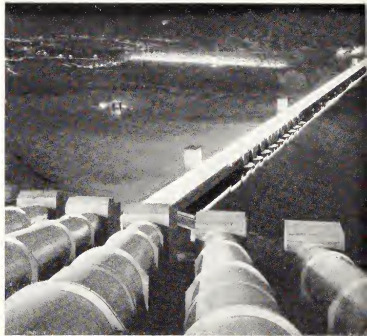
WORLD'S LARGEST PUMPS (above) lift water 280 feet out of the Columbia River, into the Feeder Canal. Farther south the water is held behind Long Lake Dam (at left). Brook Lake in the foreground. Photo above by H. W. Fuller, at left by F. B. Pomeroy, both Region 1 photographers.
