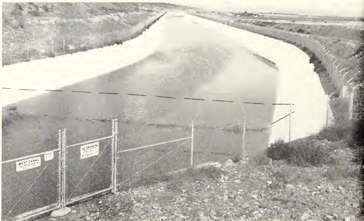
FOUR-WAY PROTECTION along the West Canal, Columbia Basin project, within the city limits of Ephrata, Wash. Fenced banks,
