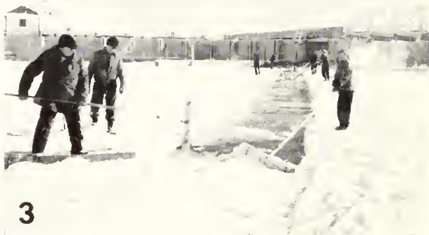
HEADING OFF THE SLUSH FROM THE HEADGATE.—(1) Wind River Diversion Dam and headgate of the Wyoming Canal, with dotted line indicating the location of the by-pass channel when the water back of the dam freezes solid; (2) and (3), opening a channel in the ice behind the dam to carry the slush ice through the log-way, and thereby divert it from the headgate of the canal which feeds water to the Pilot Butte Power Plant. Temperature—25 degrees below zero.
