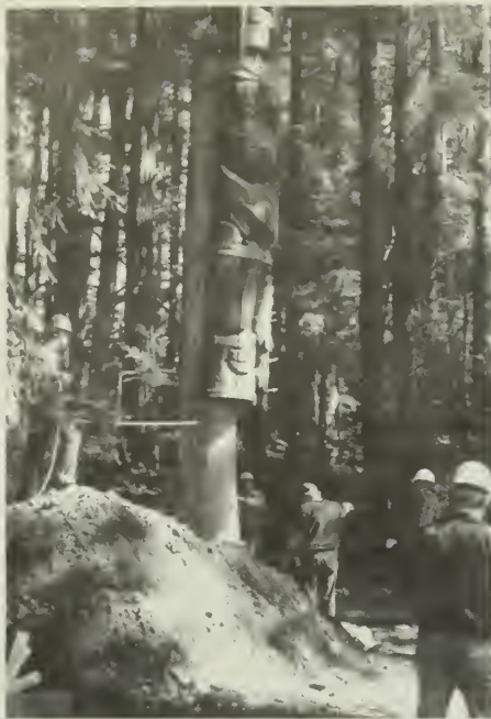
Figure 8. Due to the heavy weight of the totems, they were usually attached to their fitted support post and re-erected at the site.
