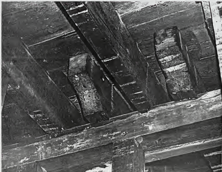
Figure 5 Former exterior cornice, later plastered over.
