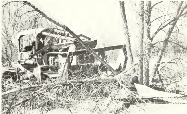
BURNING DEBRIS after all usable timber has been salvaged, at left. Timber is no obstacle to this low-cutting, bulldozer mounted blade above, which clears 5 acres of dense timber in 8 hours.
