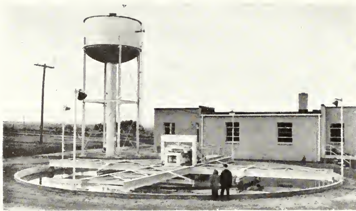
'T WAS A GREAT DAY for Lewiston Orchards when the domestic water treatment plant (above) went into operation. Reclamation and Lewiston Orchards Irrigation District officials inspect filter bed at right. Photos by Stan Rasmussen, Region 1 photographer.
