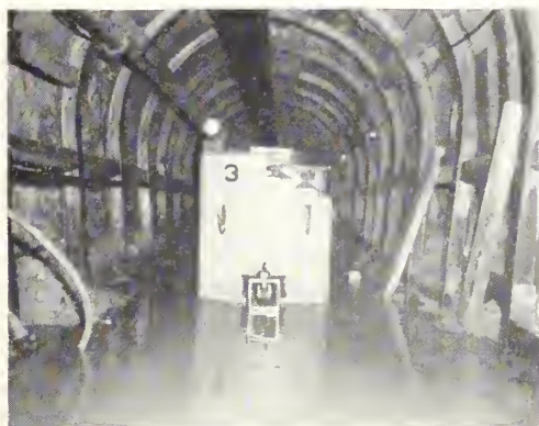
MENACING MOISTURE —Water flowing at the rate of 14 second-feet is 18 inches deep in above photo of tunnel. Above right, Duchesne tunnel, showing cave-in area in old 6-inch steel sets. At right, aerial view of Deer Creek Dam and Reservoir, Provo River project, Utah, which will get water from the other side of the mountain as soon as Duchesne tunnel is completed. Top photos by M. F. Edwards, right photo by Paul E. Norine, both of Region 4.
