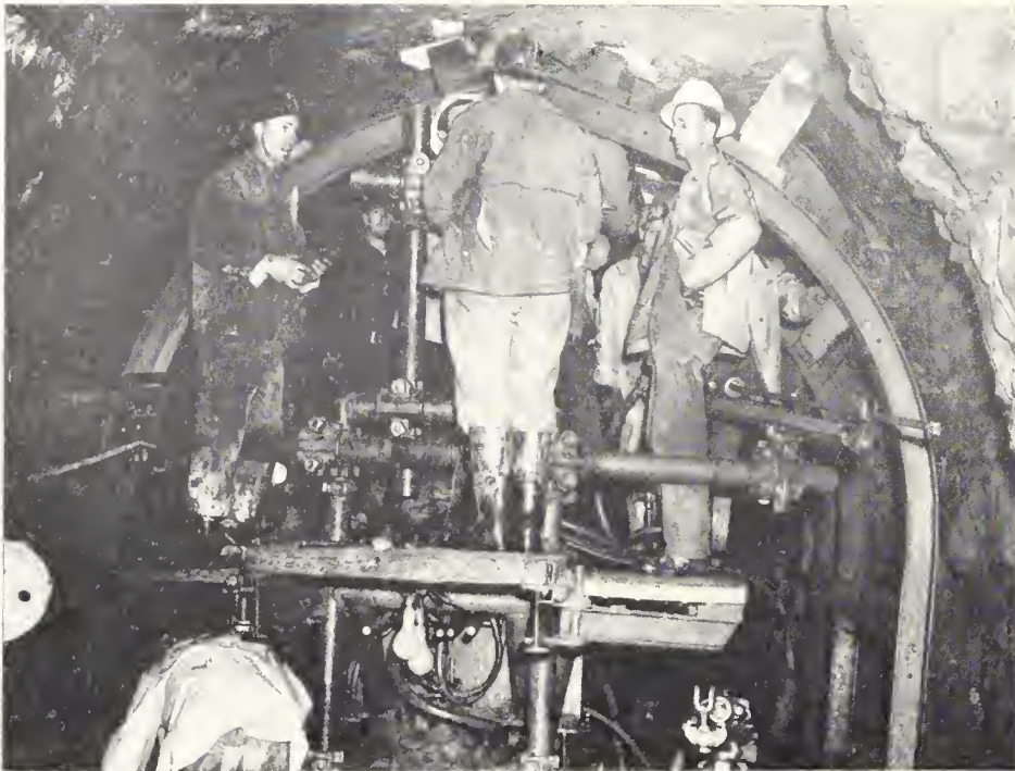
TROUBLESOME TUNNEL— Above, jumbo set-up for drilling in tight spots to install steel supports. Above right, workers' "Subway." Center right, checking the roof. Immediate right, reconditioned tunnel. Next, "Diagram for Destruction." "Diogram" photo by W. Broadfoot, Region 4, "Subway" photo, photographer unknown, others by M. F. Edwards, Region 4.
