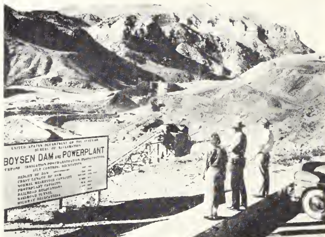
BUILDING BOYSEN —An important key to the development of the Wind River Basin. Photo by T. R. Broderick, Region 6.
