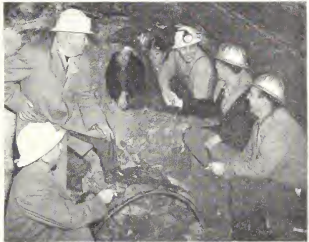
FROM EAST AND WEST—They "holed through" Pole Hill Tunnel on March 15, 1951. After the final blast the usual handshakes from those on the two ends of the tunnel were exchanged. D. E. Cartee, hard-rock miner who helped set off the final blast, receives his handshake from J. H. Knights, district manager, Bureau of Reclamation. Looking on are (at extreme left) Robert Barkley, engineer, Northern Colorado Water Conservancy District, Greeley, Colo., J. M. Dille, secretary-manager, northern Colorado Water Conservancy District, Fort Morgan, Colo., Ren Read, assistant district manager, Bureau of Reclamation, and an unidentified miner. At the extreme right is K. W. Dickey, Bureau of Reclamation field engineer. The Wunderlich Company was the contractor for drilling the 5.6 mile tunnel, part of the Colorado-Big Thompson project, in record time. They started work in September 1949, and holed through in 75 percent of the time anticipated for this part of the job. Photo by N. T. Novitt, Region 7 photographer.
