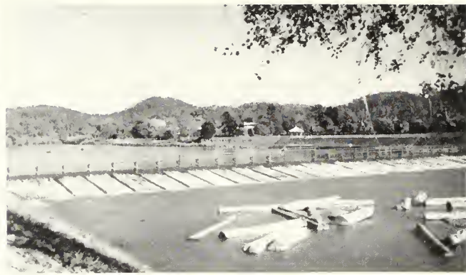
RICE RAFTS made of teakwood float right over the spillway of this diversion dam on the Me Ping River in northern Siam. This is part of the Me Fact project, 16 years old, serving about 40,000 acres, and providing much of Siam's most important crop—rice, plus many other substantial benefits.
