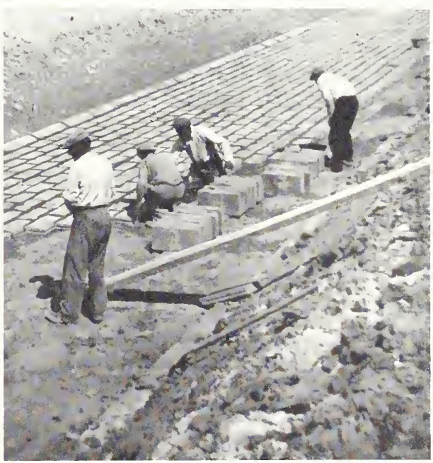
PRECAST CANAL LINING BLOCKS are set in the irrigation canal on Brian project in the Veneto region of Northern Italy.
