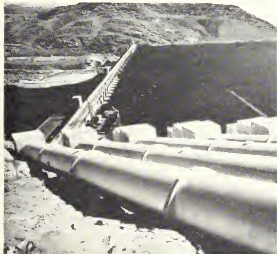
OVER THE HILL —Columbia River water will climb through the huge pipes shown immediately above. The air photo shows what will happen when the first pump starts at Grand Coulee Dam. The first pump unit, located deep inside the pumping plant (drawn in foreground) will start turning as power feeds from the L-1 generator in the left powerhouse. Water will surge up the discharge pipe, far right on the hill, into the winding Feeder Canal (center of photo). The Columbia River ultimately will fill the Grand
