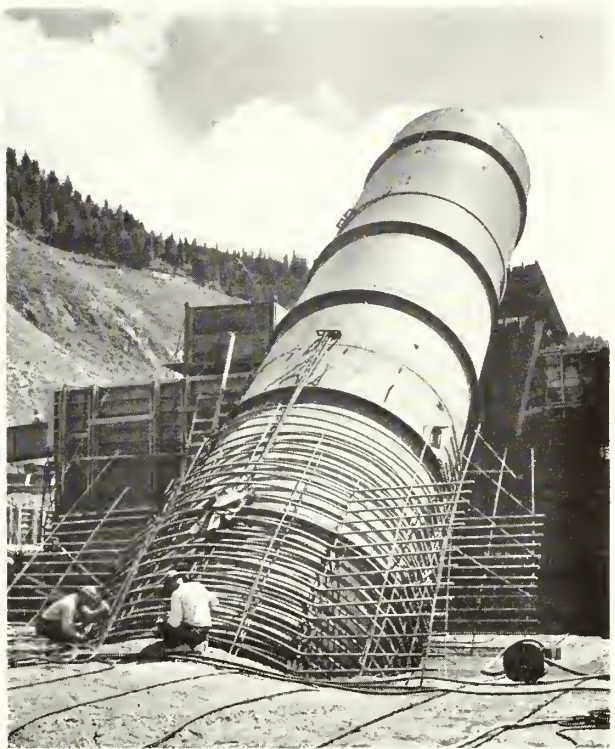
DEFENSE STRUCTURE —As truly as if it were actually the giant coastal gun it resembles is this 13½-foot penstock pipe rising from the massive concrete blocks of Hungry Horse Dam in Montana. Photo by A. E. McCloud, Region 1 photographer.
