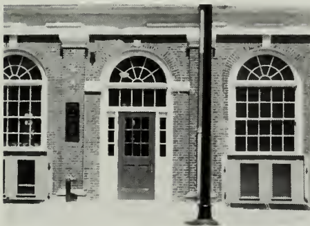
Figure 15. A new entrance to the elevator lobby replaces a window at Faneuil Hall in Boston, Massachusetts. The new entrance is appropriately differentiated from the historic design. Photo: Paul Holtz.
