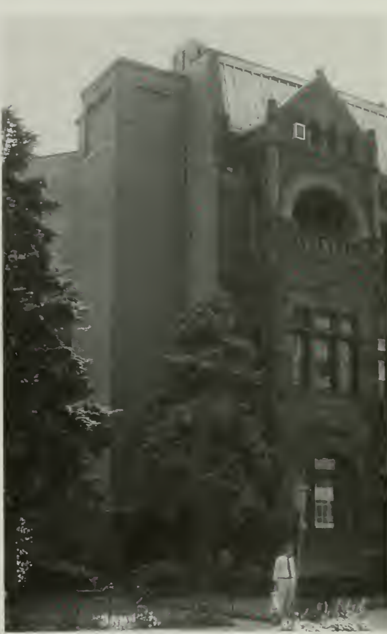
Figure 24. Creating an accessible entrance with a new elevator tower requires a compatible design. This elevator addition blends in with the historic building’s materials and provides access to all public levels. Photo: Sharon Park.
