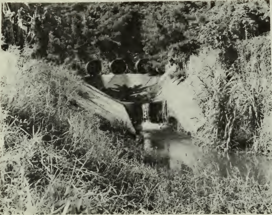
Figure 6. Road and highway crossings often involve elevated culverts (modification type 3). This elevated culvert arrangement was constructed where Kahekili Highway crosses Aolani tributary of Kaneohe Stream, windward Oahu.
