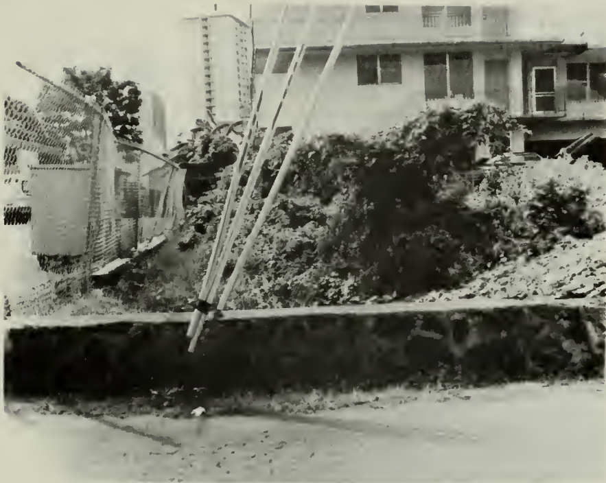
Figure 8. A filled-in portion of Pauoa tributary of Nuuanu Stream, Honolulu (modification type 5). View is "downstream" from former bridge crossing at Iliahi Lane. Foreground rock wall is part of original bridge; former channel extended from fence on left to right edge of photograph.
