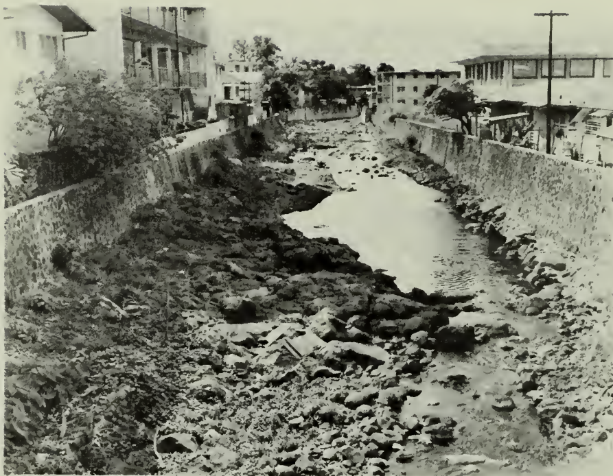
Figure 7. Revetments in Kalihi Stream, Honolulu (modification type 4). Stream bed is natural material; revetted banks consist of mortared rock and concrete sections.
