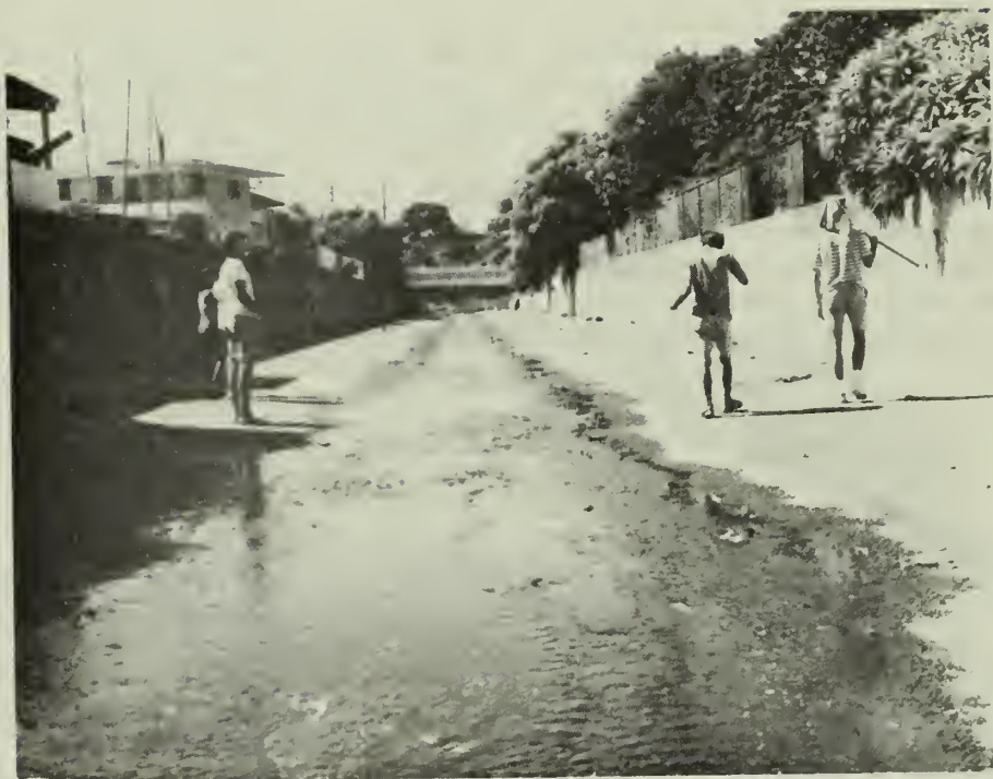
Figure 2. Lined channel of lower Palolo Stream, a tributary of Manoa Stream, Honolulu. Flat bed spreads low-flow water into a thin sheet that provides no shelter for native fishes or crustaceans and causes excessive solar heating.
