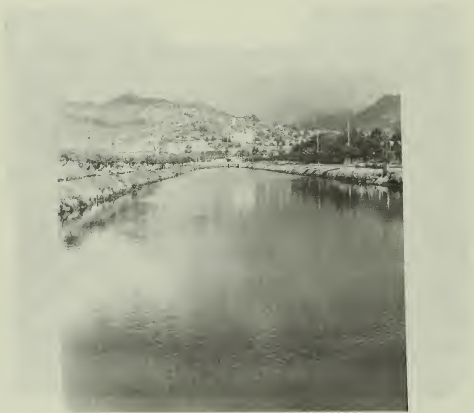
Figure 5. Kapalama Stream, between Dillingham Boulevard and North King Street in Honolulu, is an example of a realigned stream which has also been cleared of riparian vegetation (modification type 2).
