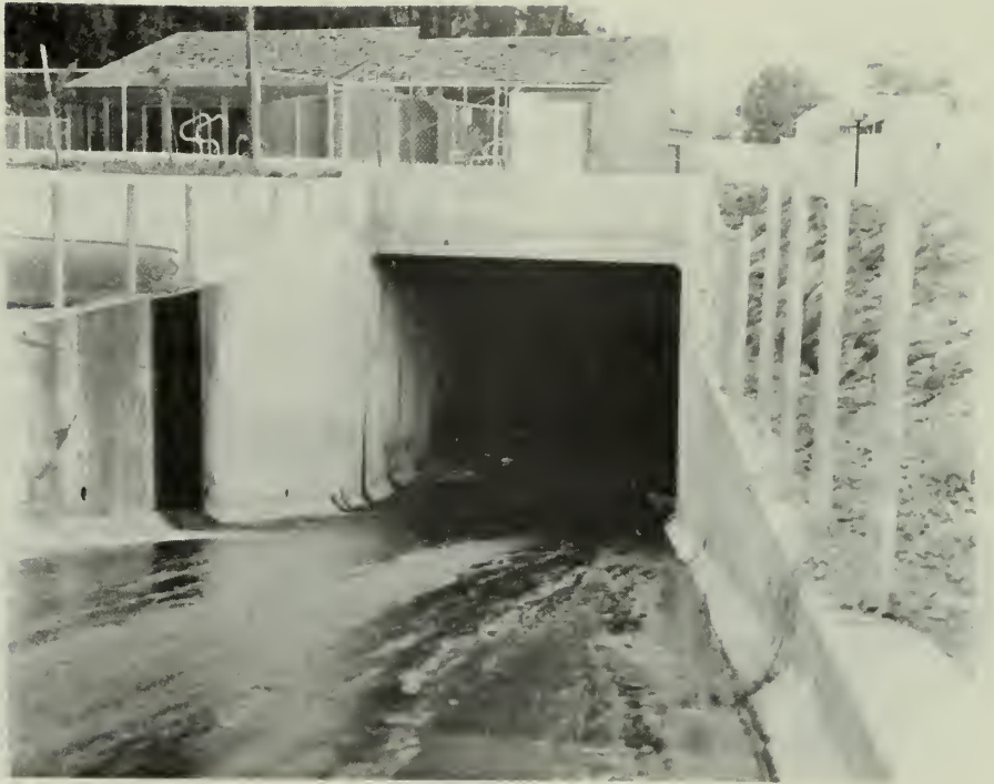
Figure 9. Upstream end of an extended culvert on Kawa Stream at Kaneohe (modification type 6). This structure is located in the Parkway subdivision.
