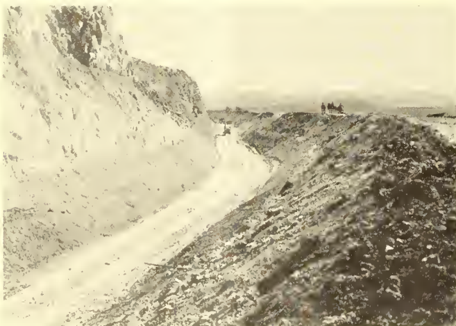
VALE MAIN CANAL, VALE PROJECT, OREGON Left: Placing earth lining. Right: Showing earth lining in place, looking downstream
