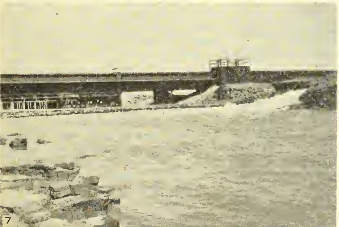
1. Rock drop, 60 feet in 4,000 feet—discharge 250 second-feet; 2, diversion to Little Wood River at crossing structure; 3, completed bench flume across lava beds; 4, sub-grade ready for gravel topping, bench flume; 5, concrete operations under way, bench flume; 6, bench flume under construction, portion of completed flume in background; 7, wasteway into Big Wood River at intake end of Big Wood River flume, discharge 250 second-feet; 8, same as No. 7. Diversion of 250 second-feet for lands on North Shoshone and North Gooding tracts
