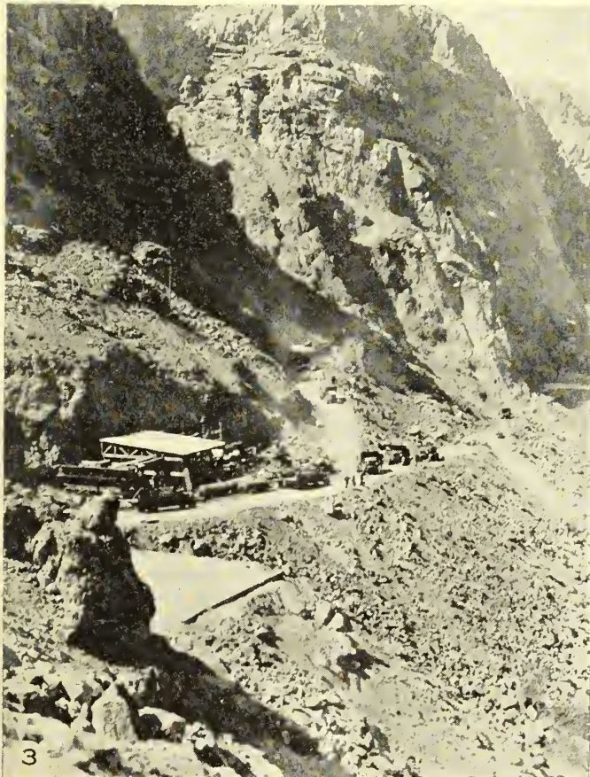
1. Excavation for sedimentation tank, Boulder City water supply. 2. Constructing presedimentation basin and water supply intake. 3. Excavation at outlets of Nevada diversion tunnels. 4. Highway at canyon under construction.
