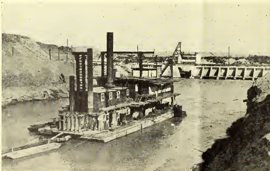
Suction dredge removing silt deposits below headgates, Imperial Main Canal
