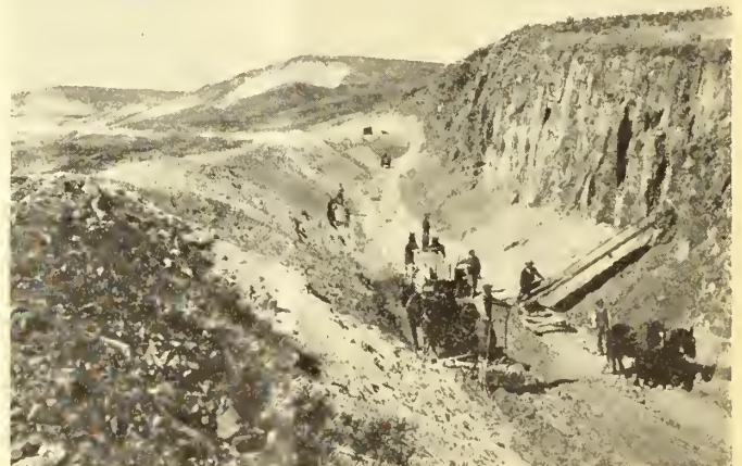
VALE MAIN CANAL, VALE PROJECT, OREGON Left: Placing earth lining. Right: Showing earth lining in place, looking downstream
