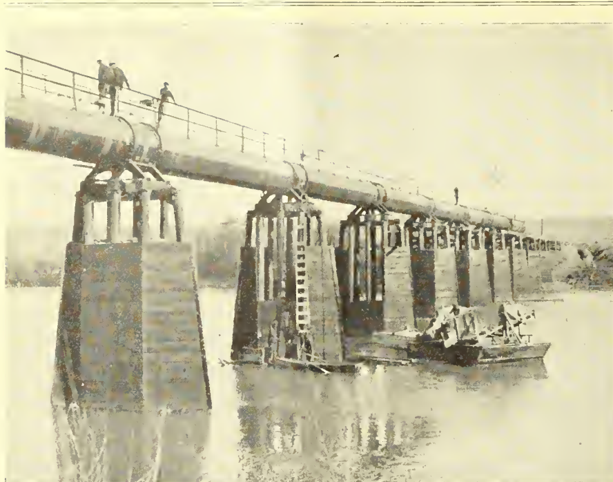
Looking northeast across river. Planking and rock filling in progress. Note skip for hoisting rock at base of pier
