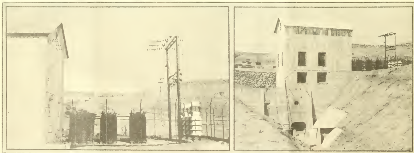
Pilot Butte power plant. Left, transformer yard; penstock, gatehouse, and wasteway intake in background. Right, tailrace view
