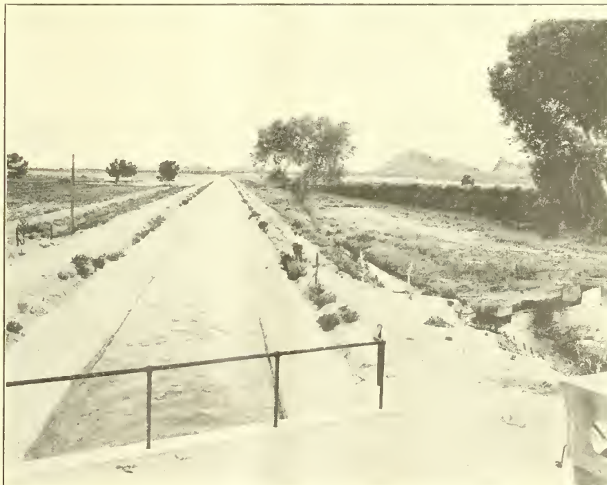
Lined section of Cross Cut Canal, Salt River project, Ariz.
