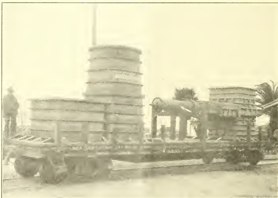
One of twenty 5 feet by 5 feet cast-iron high-pressure outlet gates for American Falls Dam, Minidoka project, Idaho. These gates each weigh 62,000 pounds, or a total of about 1,250,000 pounds of castings. Contract was, executed with the Joshua Hendy Iron Works, of San Francisco, September 24, 1924, and delivery has recently been completed. Every gate was shipped ahead of the contract schedule, and final delivery was completed approximately 50 days ahead of the final delivery date fixed by the contract. Contract price was $127,161.
