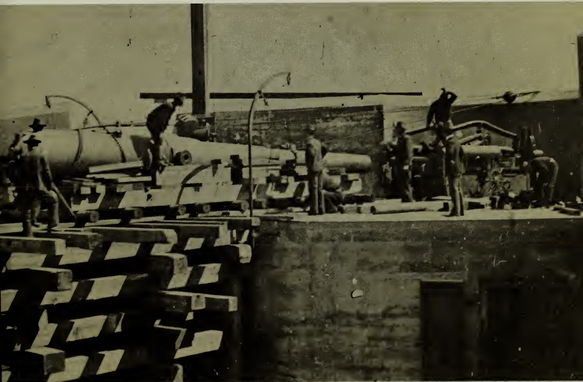
Mounting a 10-inch disappearing rifle was an arduous task without power equipment.
