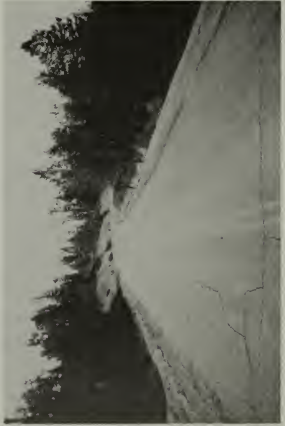
Cracked surface on Rim Road
