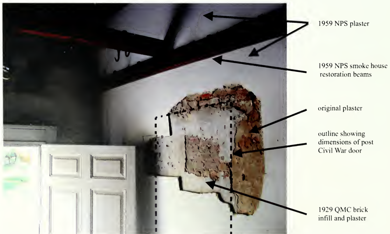
Figure 14. South Dependency, center room, northeast corner, 2002. Recent physical investigation revealed the door opening (created sometime after the QMC took over Arlington in 1861) that connected the center room with the east room. An identical opening was made on the west wall. Both allowed the Gray family interior access to the three South Dependency rooms that they occupied at the time.
