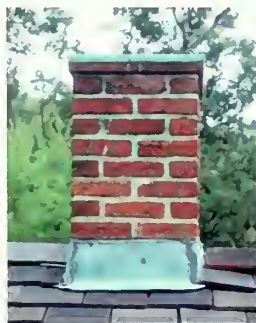
Figure 5. West chimney rebuilt in 1958-59 is currently sealed and capped.
