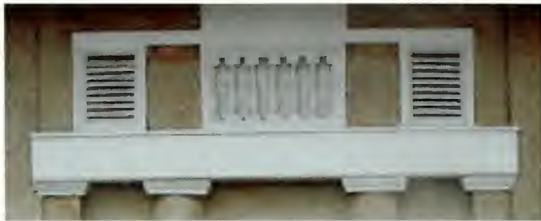
Figure 22. Two rectangular vent openings in the center bay on the south elevation open into the center room and flank a spindled wood feature.
