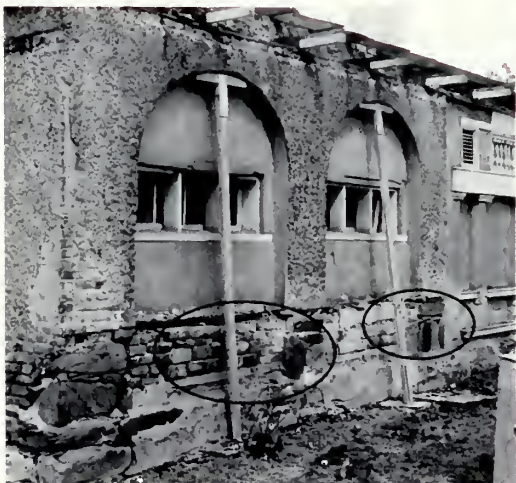
Figure 25. The 1958 photographs, showing stucco removed from lower portion of west arched bay, reveal the presence of a wood nailer strip near the bottom of the stone foundation wall.
