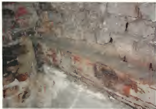
Figure 4. West room attic, southwest corner, 2003 photo showing original joist with pegged scarf joint and lime-washed finish.
