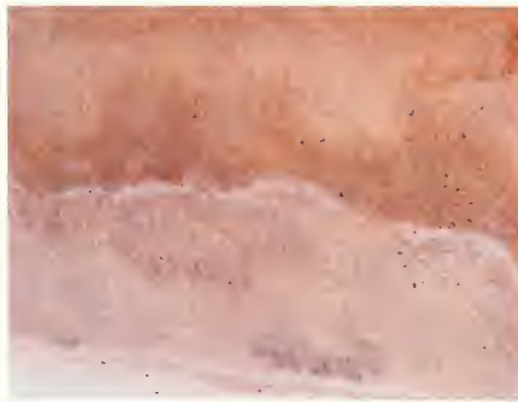
Figure 13. Efflorescence is visible on the east elevation stucco within the recessed areas.
