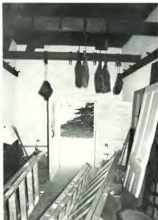
Figure 32. Center room looking north, 2003, showing interior used as storage space with the remnants of the NPS 1950s smokehouse interpretation, including the plaster, beams, hanging hooks, and replica meat. Note also NPS door assembly with inner restoration door and outer viewing door with plexiglass light dating to the 1960s.
