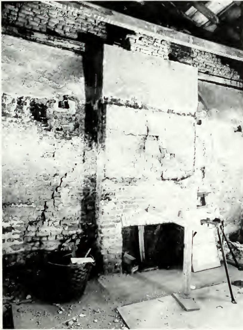
Figure 29 (left). West room, west wall, April 24, 1959 showing NPS restoration work in progress. Note the lower portion of the fireplace partially rebuilt by the QMC in 1929. Most of the upper chimney is original to the structure. The QMC restoration loft is removed exposing the joist pockets that the QMC asserted were original. Also note the plaster and lath marks above that date to the post-Civil War era when the QMC removed the historic loft and converted the space to a single level.
