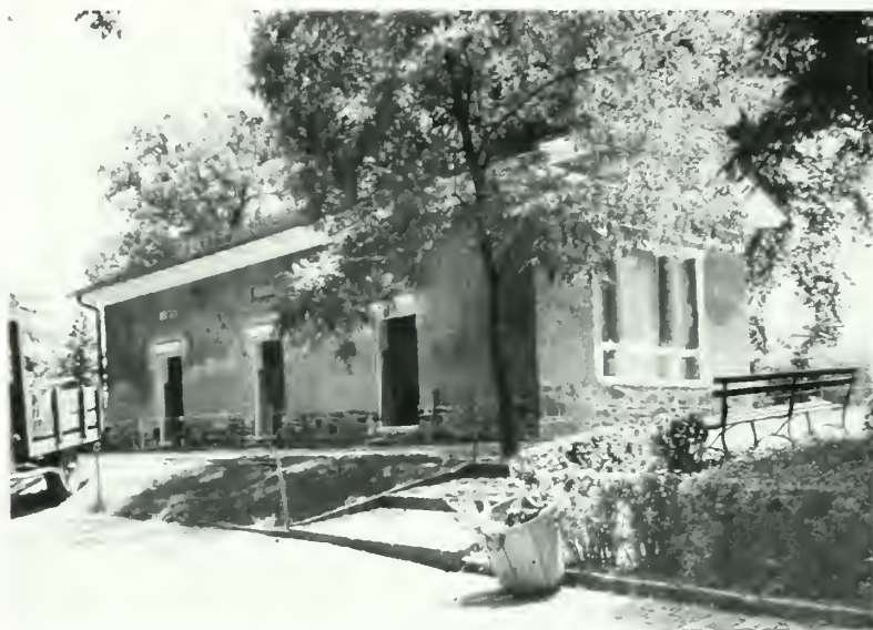
Figure 31. Southwest corner, June 1959 showing exterior following NPS restoration, including new door cornices, repaired roughcast and woodwork, and repointed masonry foundation.
