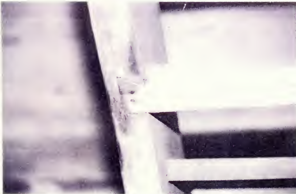
Image 4.90 WC. On the backside of the ladder/stairs was a stabilizer bar. A close up view of the north end of the bar with a delicately cut half dovetail notch into side of stringer. Each end of the stabilizer bar was nailed with two small brads. Note too that the tread dado does not extend through the width of the closed stringer. The back of the treads stopped in the dado prior to reaching the backside of the stair carriage.
