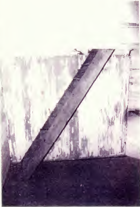
Image 4.85 WC. Ladder stairs located in northwest bedroom R103 against south wall. Made of black walnut expertly hand planed smooth by a master craftsman and nailed together with hand wrought, rose head, spoon bit nails dated 1802-1803. Originally the bottom edge of the stairs touched the east log wall. During the 1979 restoration, the little stairs was reset a few inches west of its original location.
