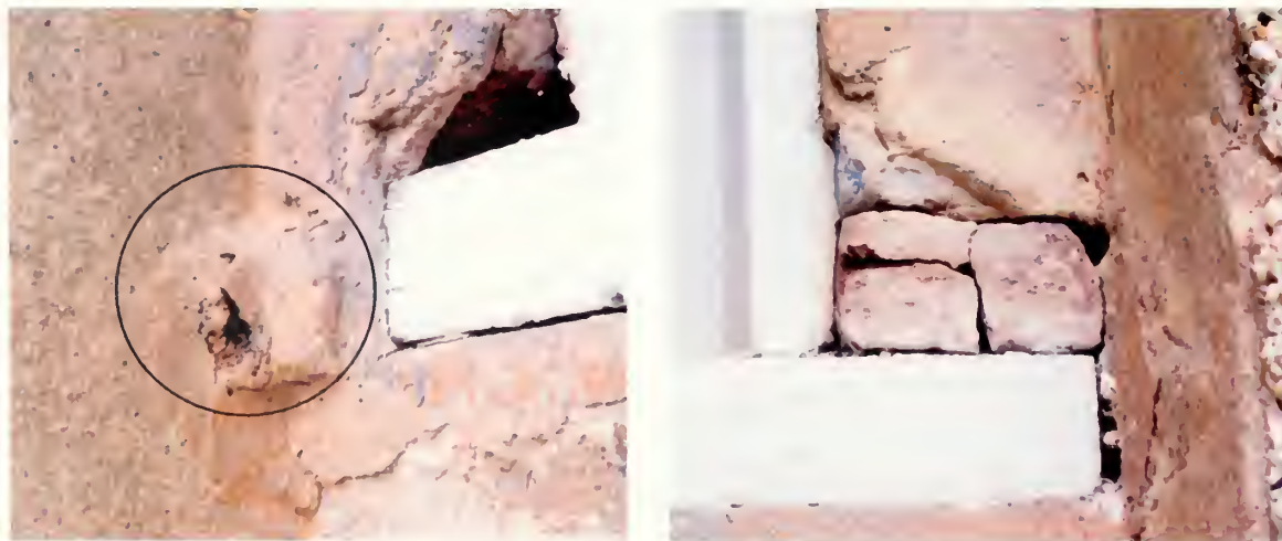
Figures 18 (left). The ears of the window sills extend to the abutting arch wall on the east but have been cut shorter on the west ends. Blocks of wood, presumed to be once the ends of these pieces, are extant in the abutting walls of various openings. Figure 19 (right). Edges and ends of indow sills and frames are exposed to the elements in many locations.
