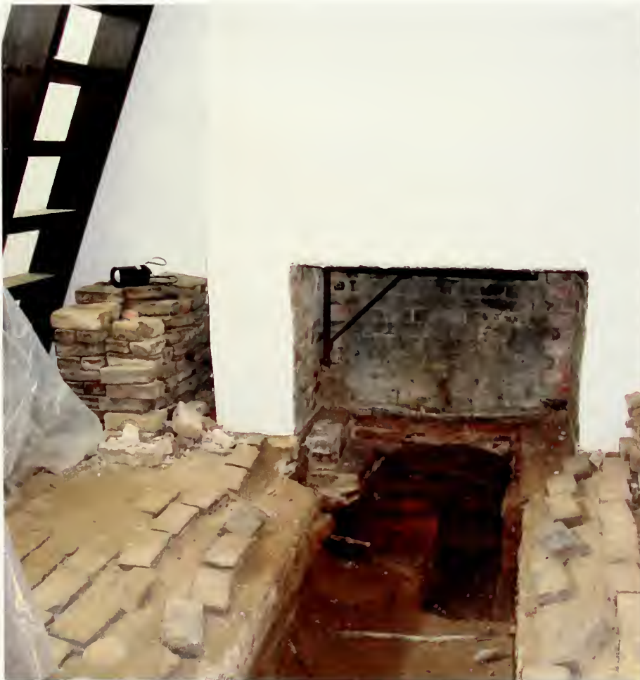
Figure 10. Recent archeology reveals that the historic floor was less than an inch below the current brick floor and that the hearth and floor had a dirt finish, 2004.
