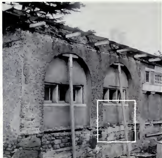
Figure 3. South wall, 1959, showing different brick patterns within arches. The area within the box is where rows of larger blocks appear to correspond to altered surfaces.
