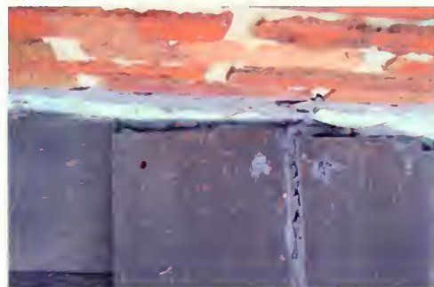
Figure 6. Tar seals to the tile roof have failed in a number of locations allowing water to infiltrate.
