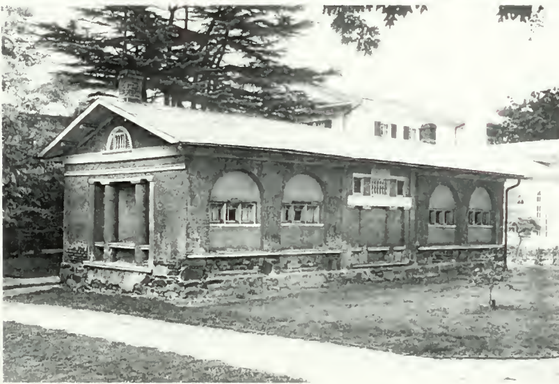
Figure 25 (top left). Southwest corner, 1957, exterior conditions before the NPS restoration. Note deterioration of rough cast along lower third of facade. Metal gates across the doorways allowed visitors a view into each of the rooms.
