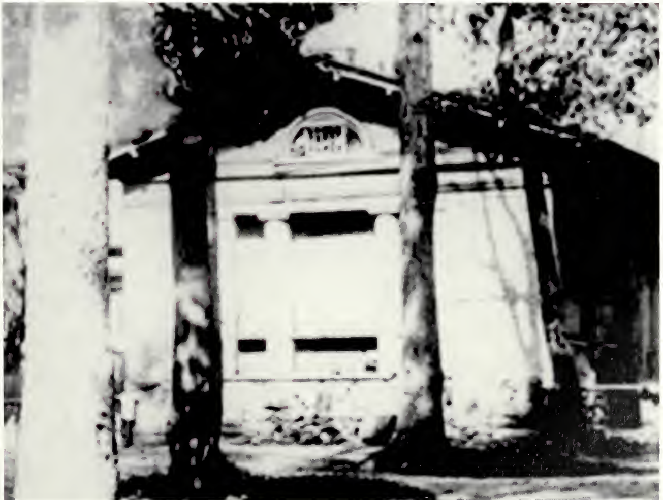
Figure 6 (left and below). West elevation, 1864, original and close-up. Photos by Andrew Russell show that the South Dependency was poorly maintained at the time. Note the missing louvers in the arched attic vent and the deteriorated mortar joints in the exposed masonry foundation.
