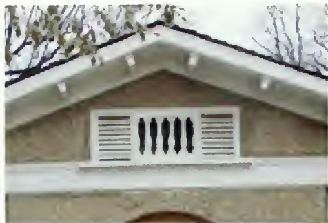
Figure 21. Attic vent on east end needs to be cleaned and painted
