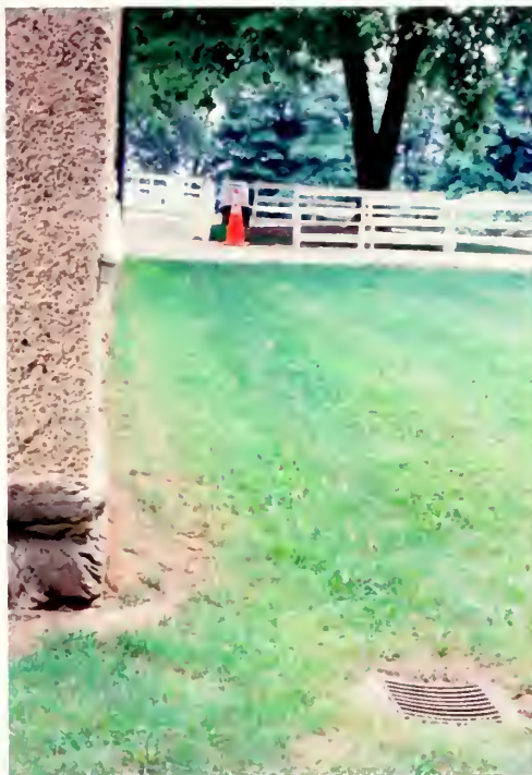
Figure 3. South elevation showing the problematic grade slope and an underground drain cover.
