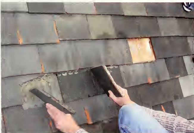
Figure 9. Delamination, chipping, crazing, and structural failure of shingles are widespread.
