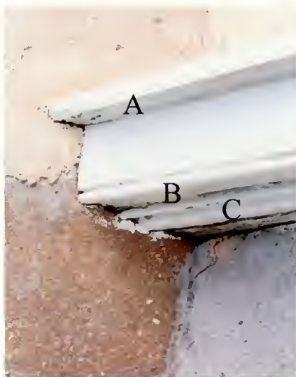
Figure 23 (left). The original configuration for the wood skirtboard that extends the length of the building on the south is a three-piece construct consisting of (A) a simple sill plate, (B) an apron with a molded drip edge, and (C) a molded trim piece set up into the back of the apron to seal and cap.
