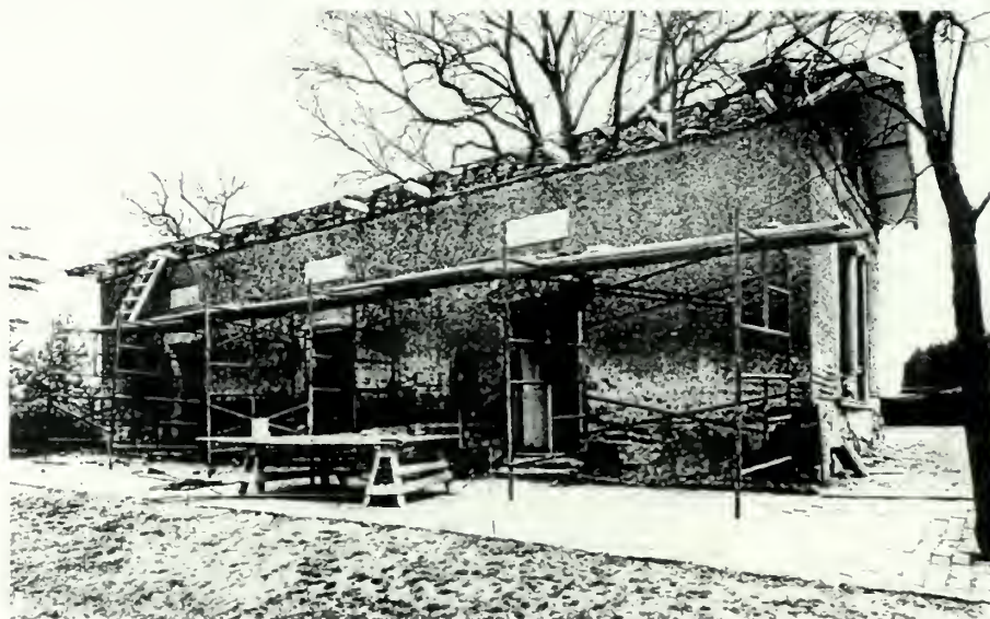
Figure 28. South Dependency, north elevation, showing NPS restoration underway. Note removal of roof sheathing, soffits, cave outriggers, and other wood moldings, March 26, 1959.
