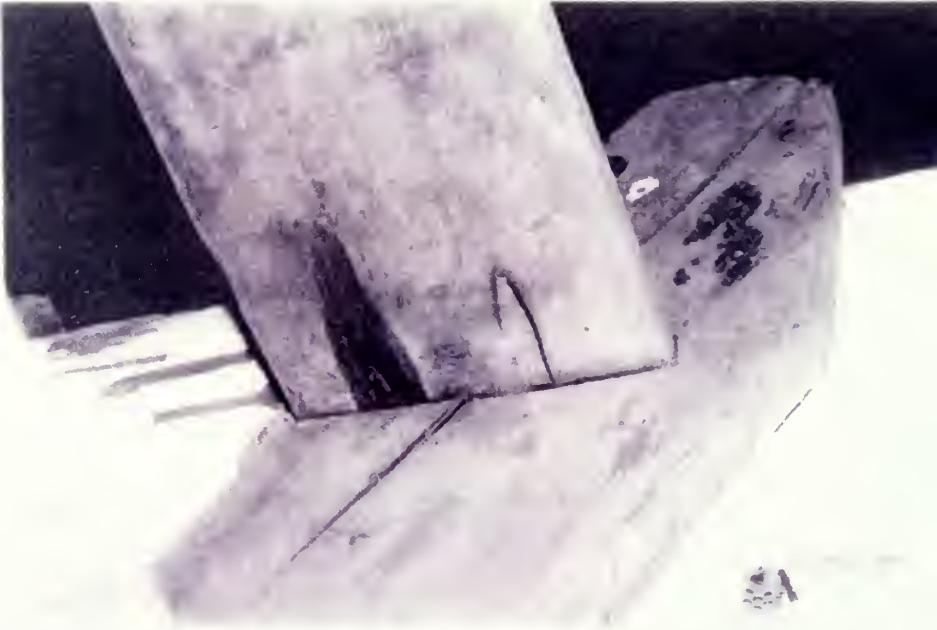
Image 4.87 WC. Underneath side of top tread at south end the split wood revealed a spoon bit nail end used to fasten the stringers to the treads. The treads were set into a recessed dado for support.
