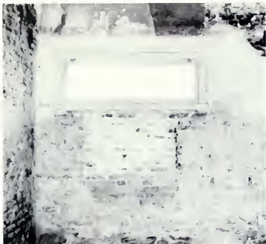
Figure 2. West room, south wall, 1959, showing ghost of former late nineteenth century window opening.
