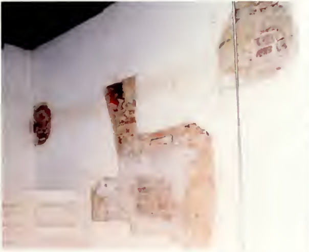
Figure 30. Southwest corner showing evidence of the nineteenth century opening in the west wall which postdates 1860.
