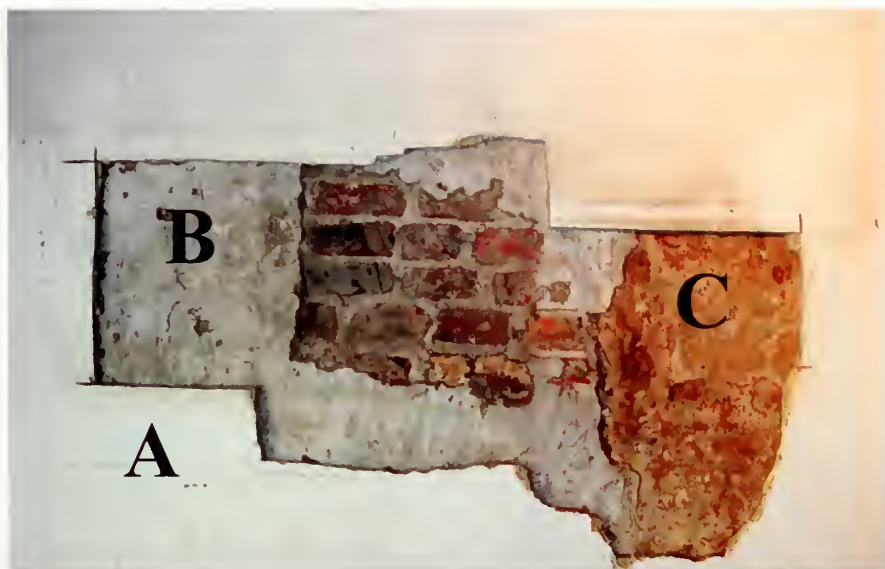
Figure 11. Center room, east wall, 2002. Intact 1959 plaster (A) has been removed revealing QMC plaster (B) covering brick infill over an interior door opening created when the Gray family occupied all three South Dependency rooms after the Civil War and infilled before the 1929 QMC restoration. When examined through a microscope, the original plaster (C) showed a considerable accumulation of soot and oil—remnants of the room's original function as a smoke room for meat.
