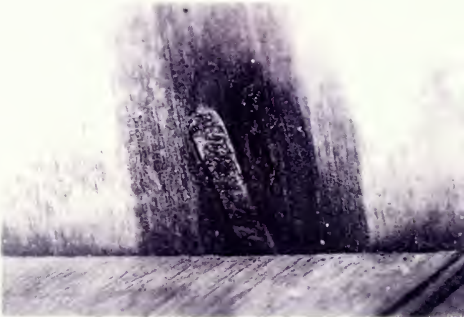
Image 4.88 WC. West Cabin, attic stairs, spoon bit end of hand wrought nail sticking under top tread. Nail dated 1802-1803.
