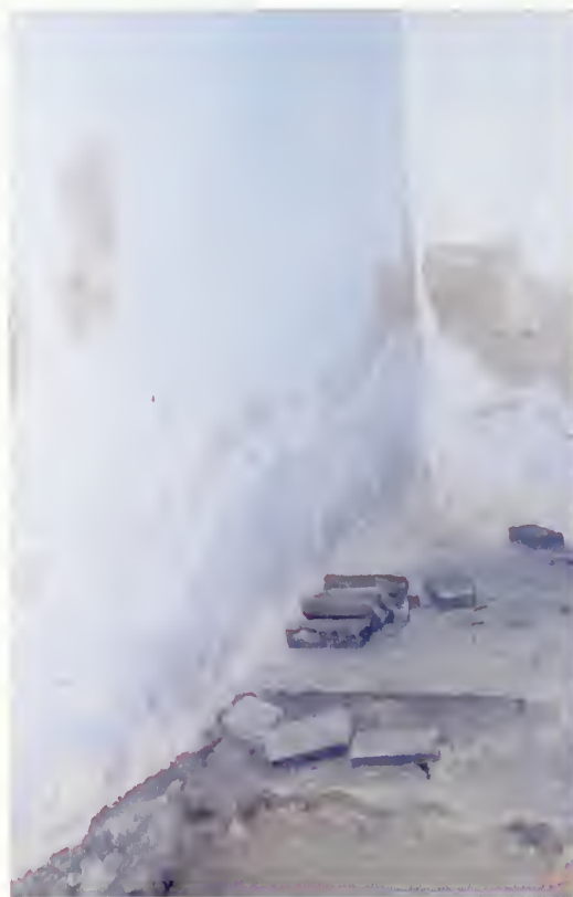
Figure 1. Center room, east and south walls show evidence of rising damp.
