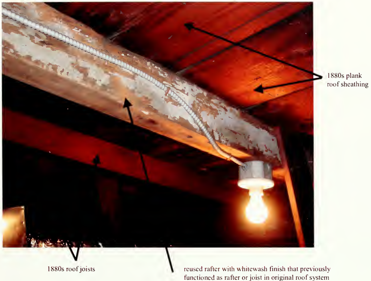
Figure 5. West room attic, south pitch, 2003. This rafter was reused when the QMC rebuilt the South Dependency's roof in the 1880s. Its whitewash finish matches an original joist from the same location that is known to have not been moved to another position ( shown in Figure 4 ). This suggests that though the rafter may not be in its exact original position, it is probably original to the South Dependency roof system.
