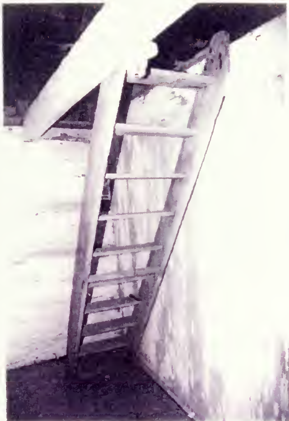
Image 4.89 WC. Back side of ladder/stairs located in northeast bedroom R103. Just above the fourth tread up from floor was a stabilizer bar to keep the lower edges of the stringers sturdy. The top ends of the stringers were originally down lower, flush with the tops of the attic joists.
