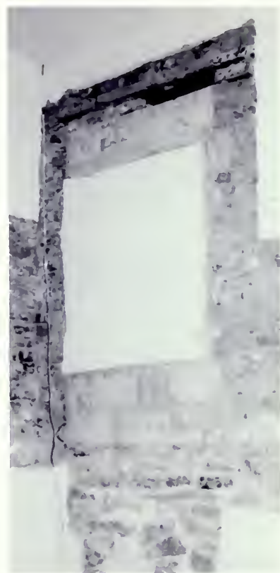
Figure 20. Infilled door opening in center room. This passage had been cut after 1860 to permit the Gray family full use of the three rooms
