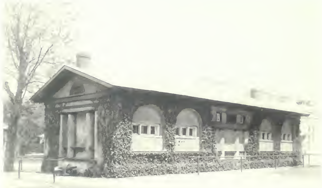
Figure 16. South Dependency, south elevation, 1897. Note the dark color of the moldings on the west elevation and portions of the south elevation. The offset between the window sash and the window mullions currently found on the building are also visible here.
