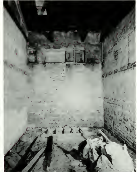
Figure 30 (above). Center room, April 24, 1959 showing removal of QMC smokehouse exhibit during NPS restoration. The 1880s roof structure is seen above and sections of original plaster are visible on the walls.
