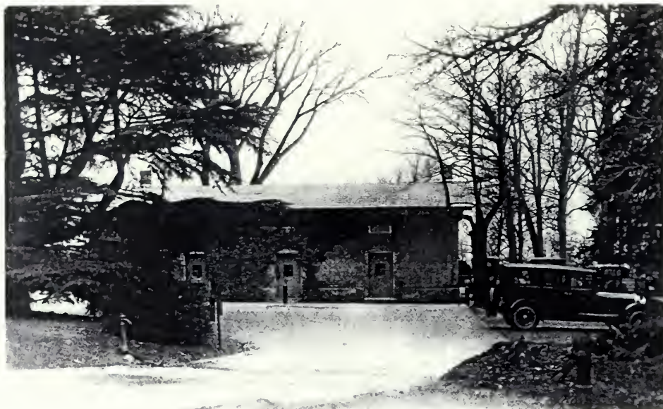
Figure 18. South Dependency, north elevation, shortly after the QMC restoration, 1923. Ongoing moisture issues are plainly evident on the lower portions of the wall.
