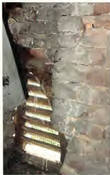
Figure 28. The header is missing from above the attic ventilation unit, west wall.
