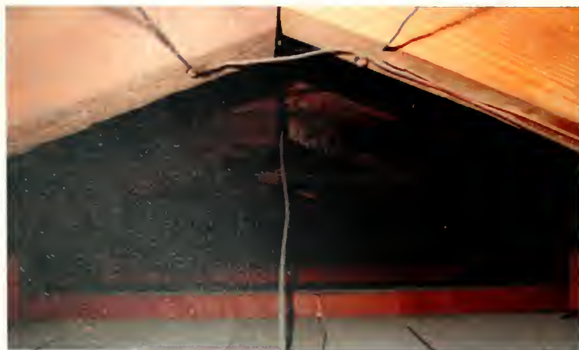
Figure 7. Counterbalanced rafter design roof construction without a ridge board dates to the 1880s.
