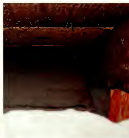
Figure 8. Outrigger formed from continuous ceiling rafters that cantilevered past the bearing walls.
