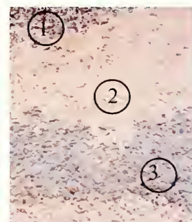
Figure 15. Three different applications of rough cast stucco: 1. The Army's brown 1929 restoration mix, 2. The 1958 NPS restoration mix and 3. A gray repair mix applied more recently by NPS.
