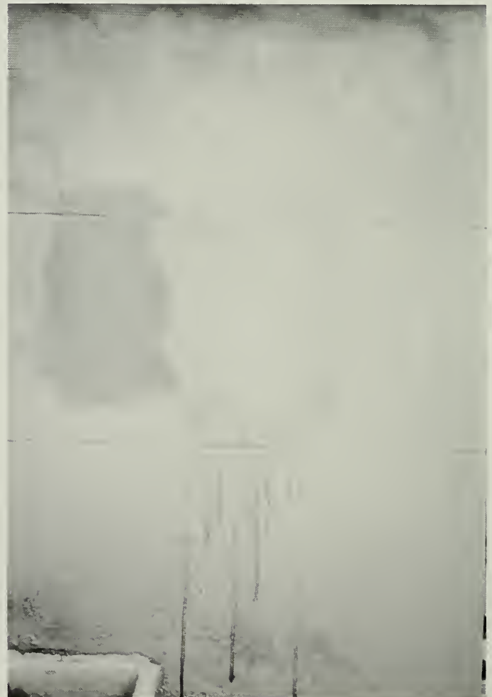
Figure 6. Although an aerosol graffiti remover has taken off much of the graffiti, it has left new stains where it dripped down the masonry surface. Photo: Ken Lustbader.
