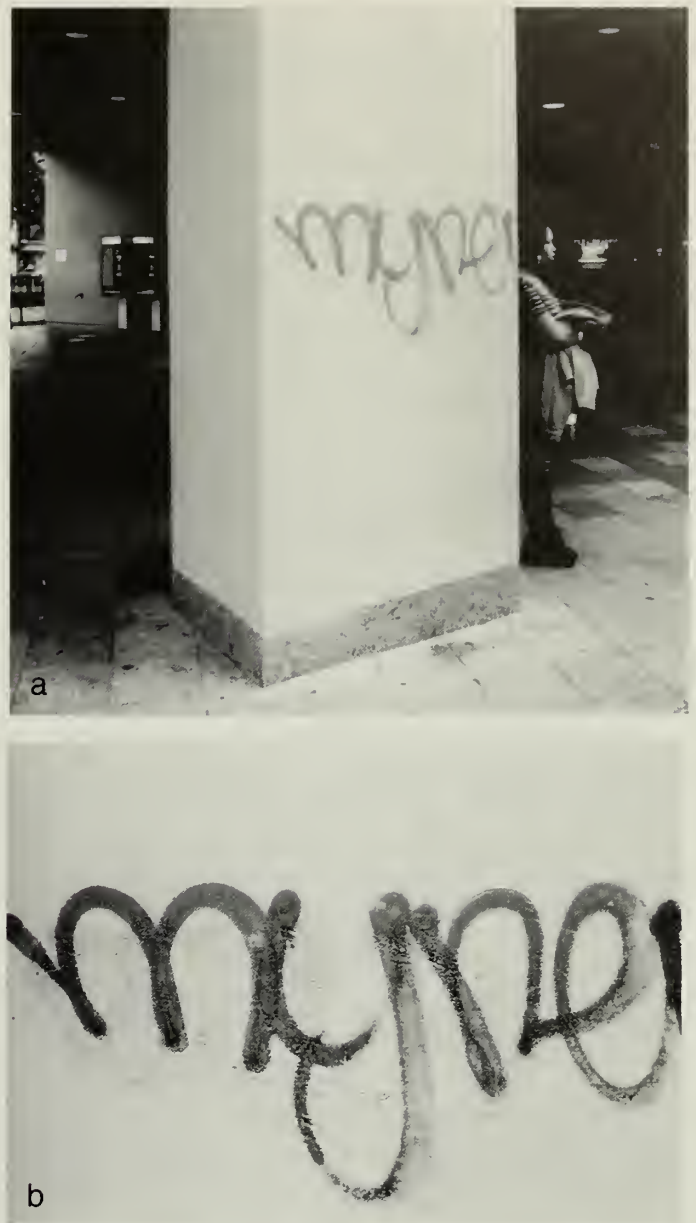
Figure 7 (a-b). The first time this spray-painted graffiti appeared it was removed abrasively. As a result, the graffiti was permanently etched into the limestone and cannot be concealed even by the pigmented barrier coating painted over it later. The barrier coating did, however, facilitate non-abrasive removal of graffiti the next time it was applied. Photos: Anne Grimmer.
