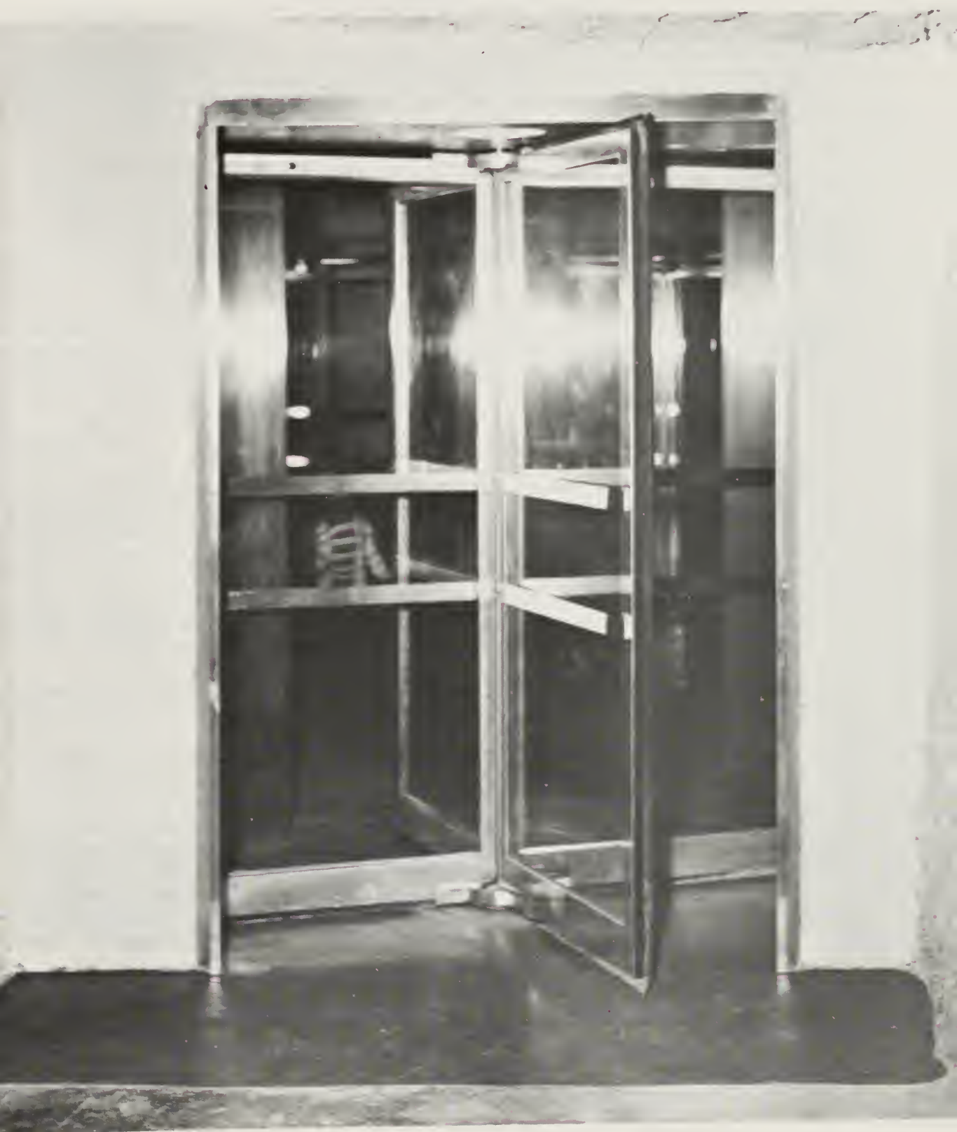
FIG. 4. REVOLVING DOORS BETWEEN UNDERGROUND LUNCHROOM AND ELEVATOR LOBBY RETAIN WARM, HUMID CAVE AIR. CACA Photo.
