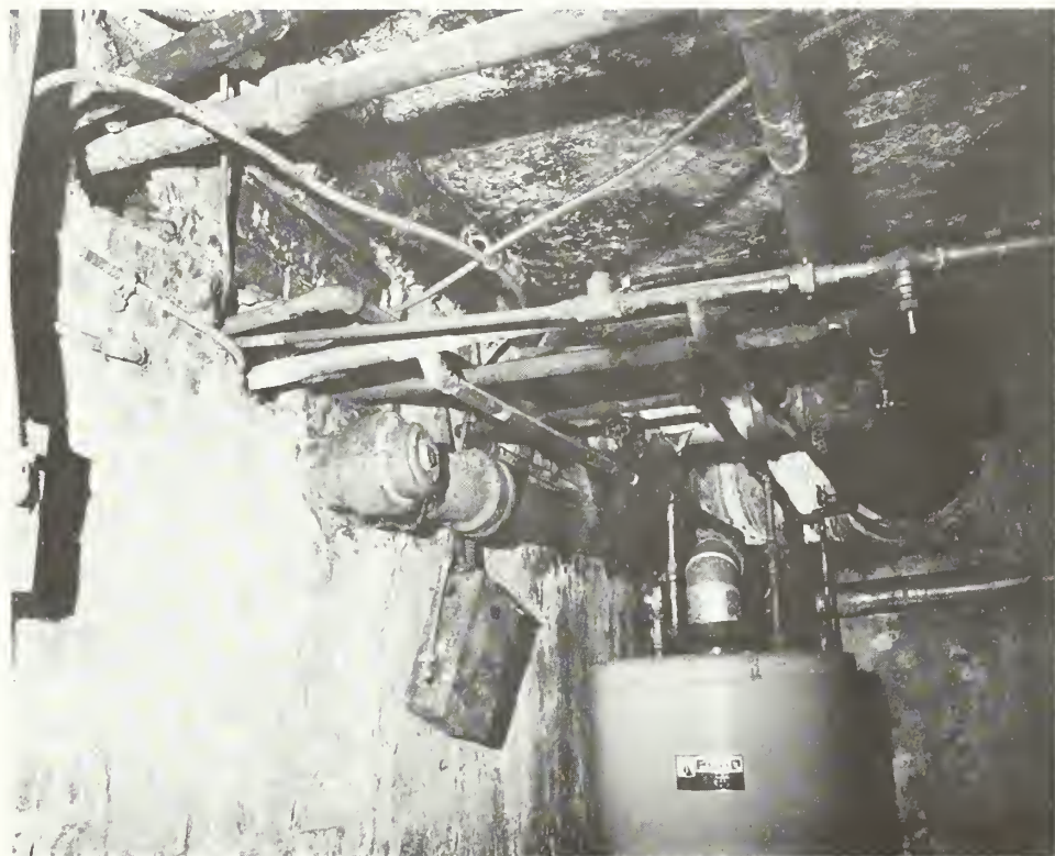
The general deterioration and needed replacement of furnace equipment makes NPS liable for this building it owns.
